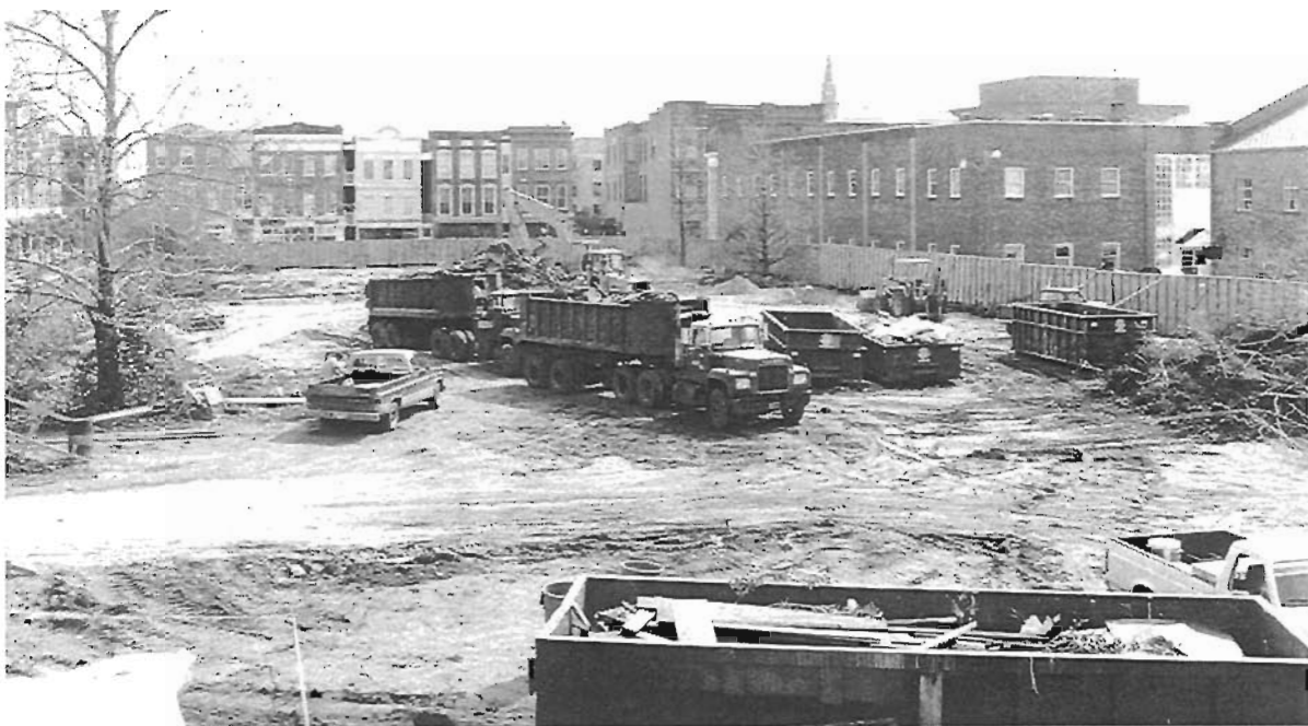
Figure 55. Eastern half of the project block showing construction activity and the removal of the demolished bank building.
