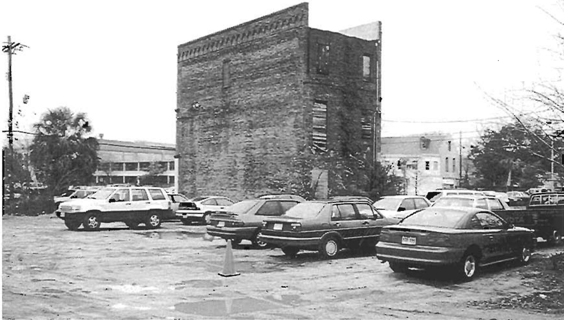
Figure 39. Western half of the project block, view toward the northwest showing the standing structure on the corner of Archdale and Market streets.
