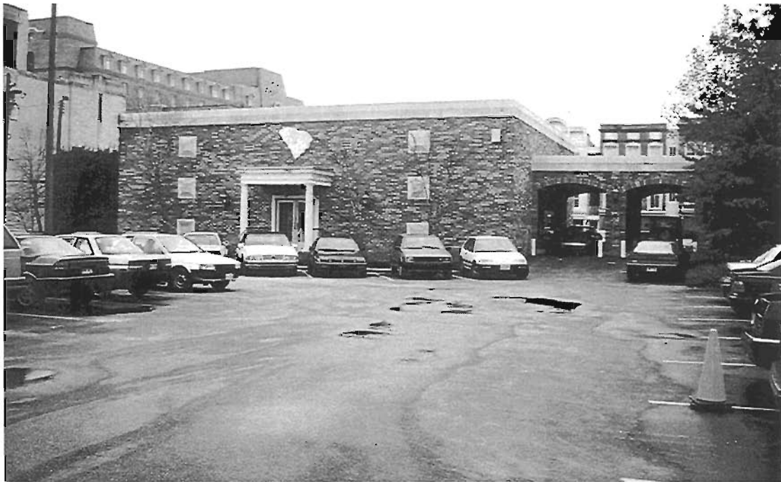
Figure 40. Eastern half of the project block, view to the northeast showing the vacant bank building.
