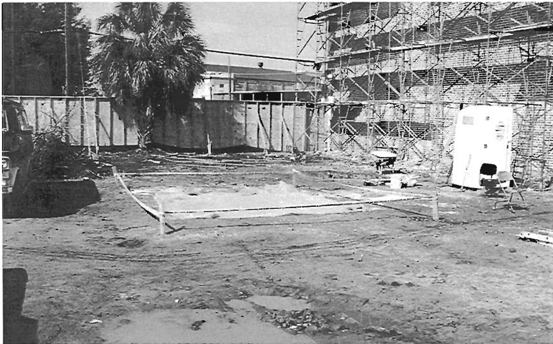
Figure 63. Area of Unit 3, south of 40 Archdale Street, behind 38 Archdale. View to the northwest.
