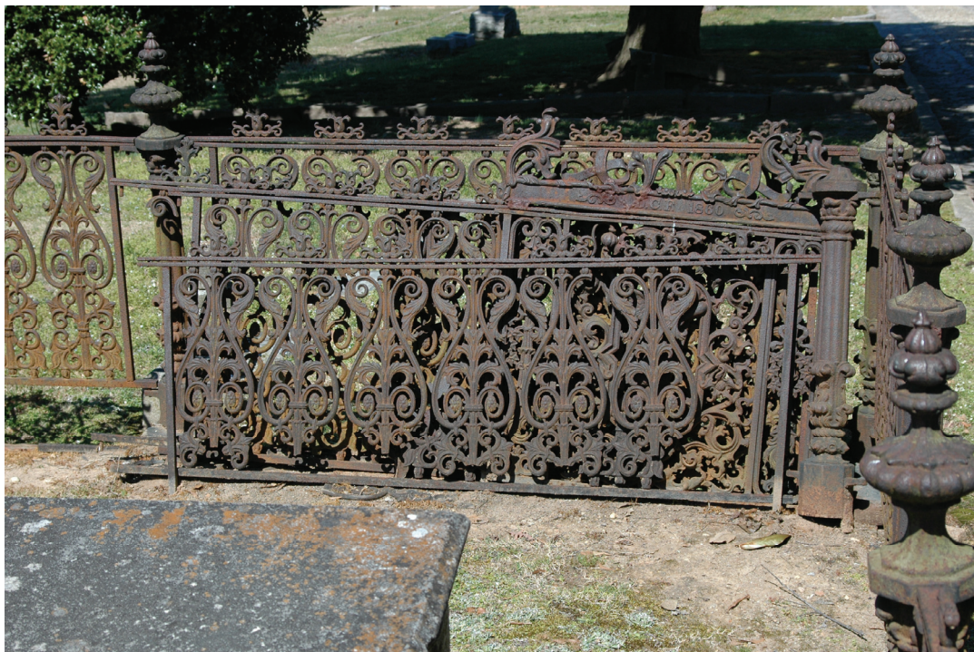
Figure 33. Fencing that invites theft and vandalism. The top photo shows an unsecured gate that could be stolen in minutes. The bottom photograph shows stacked fencing and a gate that are unsecured and could be easily stolen.
