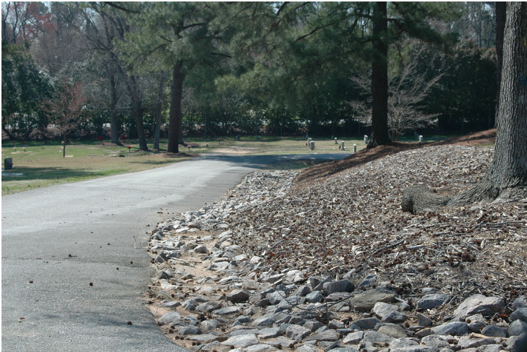
Figure 28. Erosion in Mount Hope. Top photograph shows an area of erosion. Areas have landscape timbers or mulch being used for control. Bottom photograph shows excellent use of granite rip rap to control erosion. This approach should be expanded throughout the cemetery.
