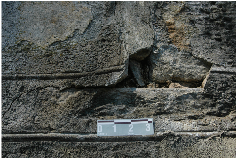
Figure 41. Spalling of a concrete stucco on the Mount Hope mausoleum.
