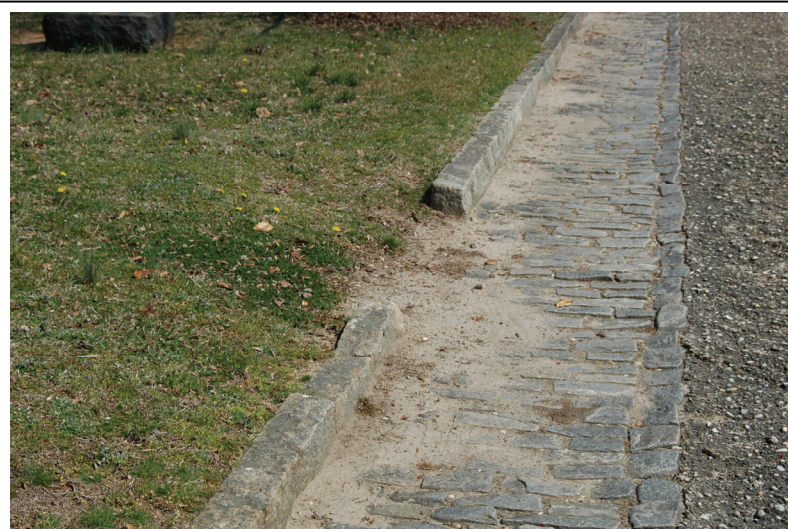
Figure 24. Loss of granite curbing. This requires replacement in order to prevent additional damage and cost.
