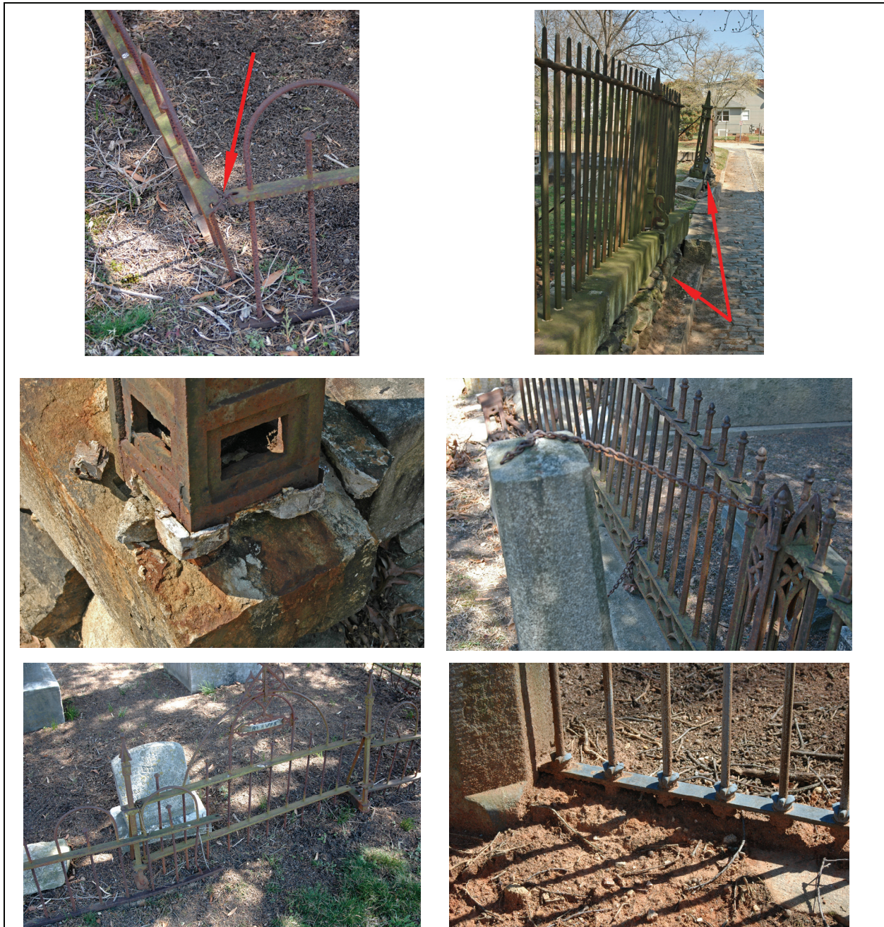
Figure 38. Typical fence problems. Upper left shows a fence being held together with ferrous wire. Upper right illustrates the failure of the fence coping, resulting in leaning and eventual collapse. Center left shows extensive iron jacking and dislocation of the lead used to set the fence. Center right photo reveals a plot chain being used to retain an adjacent plot fence. Lower left shows a gate that no longer fits its opening and that is unsecured. Lower right shows the O'Rourke fence partially buried in soil – which exacerbates corrosion.
