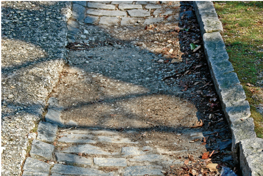
Figure 23. Inappropriate repair of damaged granite blocks using concrete.
