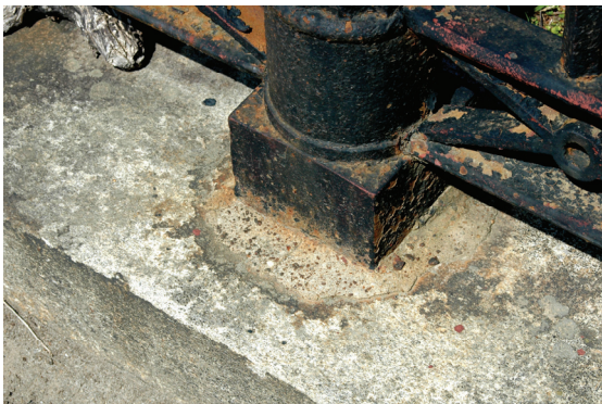
Figure 40. Boundary fence problems at City Cemetery. Upper photos show extremely poor efforts to replicate finials. Middle left shows missing cap with exposed central rod. This is allowing corrosion within the post. Middle right illustration shows a line post with corrosion that has penetrated the sides. Lower left photo shows a line post reset in concrete. Note also the extensive corrosion. The lower right photo shows damage to the fence and granite coping caused by an adjacent tree.
