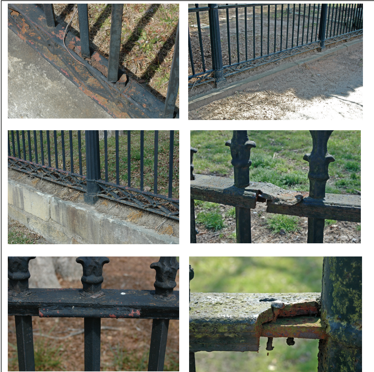
Figure 39. Boundary fence problems at City Cemetery. Top left shows paint failure and resulting heavy corrosion. Top right and middle left both illustrate sections of fence partially buried in soil. Middle right and lower left show inappropriate welds that no longer allow movement of the fence sections. The weld in the first photograph has failed because of this. This weld also illustrates extensive corrosion resulting from poor workmanship. The lower right photograph shows a slip joint with the top rail connected to the line post using a rivet. This allows appropriate expansion and contraction of the fence section.
