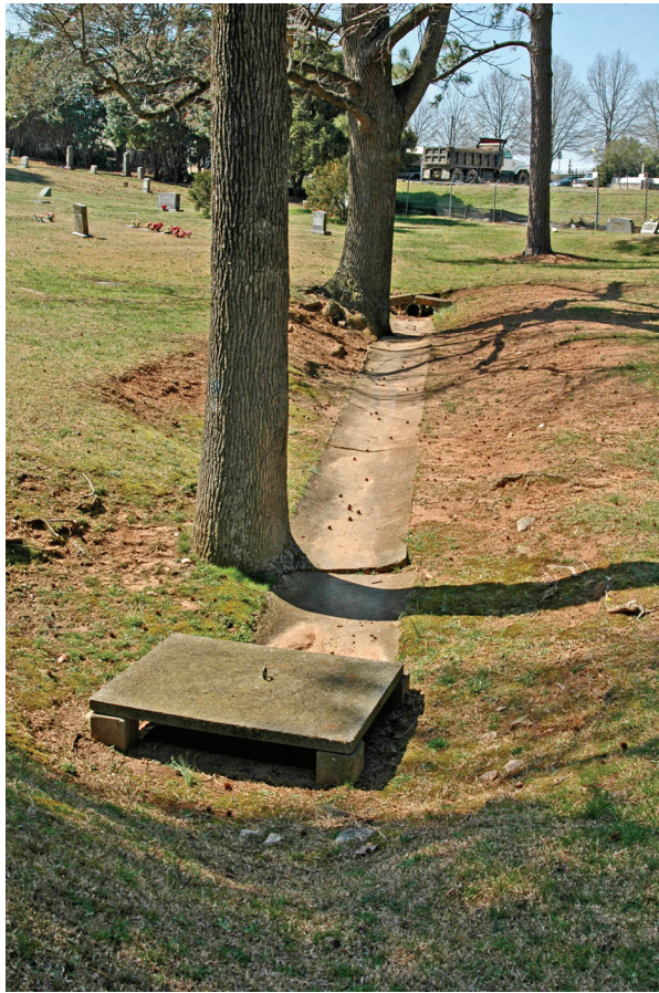
Figure 29. Unattractive open drain in Mount Hope. This could be improved through the addition of rip rap.
