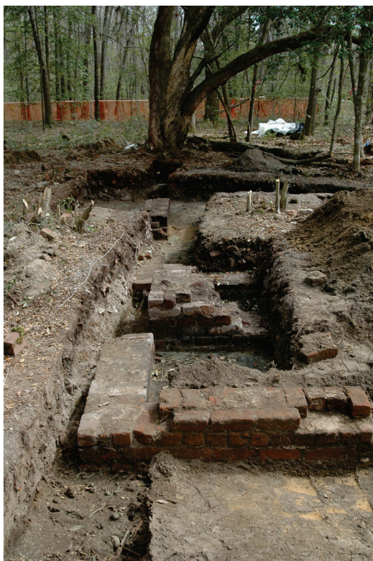
Figure 24. North wall of the eastern structure exposed by excavations and stripping. View to the east.
