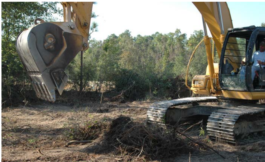
Figure 14. Use of heavy equipment to bisect the wells, allowing for safe excavation.
