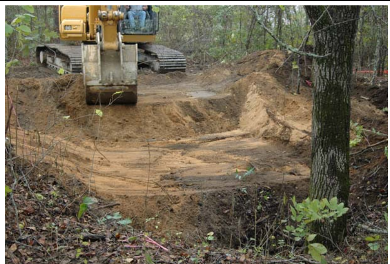
Figure 21. Opening the excavation area. The feature is in the right foreground.
