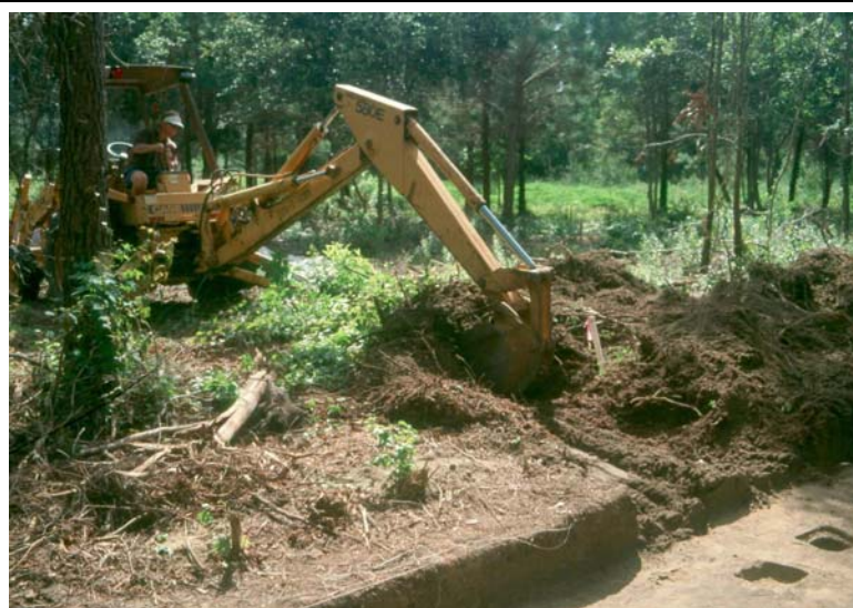
Figure 17. Use of a backhoe to expand recovery of structural patterns.
