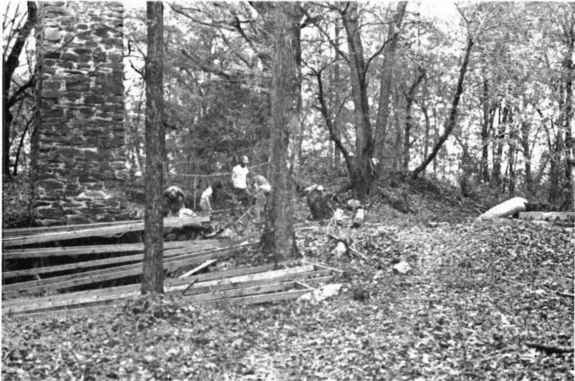
Figure 8. General view of the site area in November 1985, view to the west.
