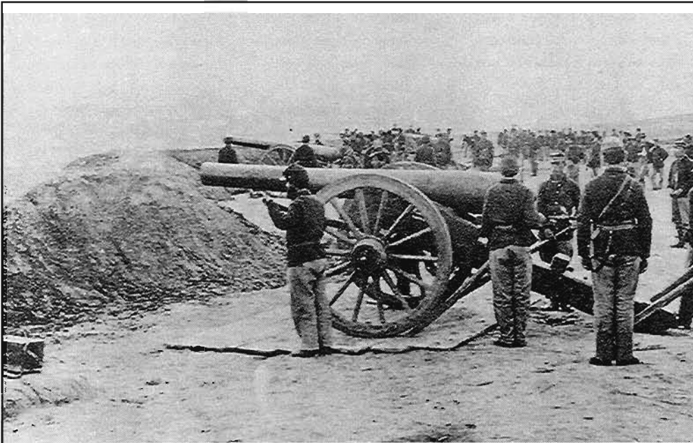
Figure 5. Battery of siege and garrison rifles on siege and garrison carriages firing "en barbette" over a quickly erected indented line (US Army Military History Institute).
