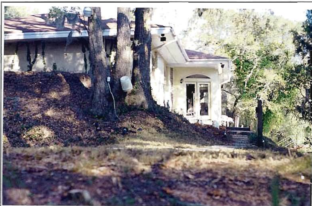
Figure 18. Battery Palmer (38CH1799, Site 3) with house built partially on the parapet (view is to the southeast).
