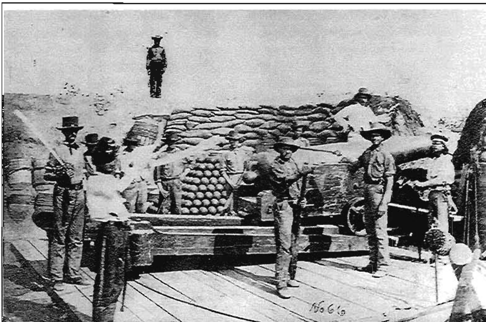
Figure 6. Confederate battery using a Navy seacoast gun, probably a 32-pounder on a seacoast carriage, firing embrasure. Note the sandbags and barrels forming the interior slope of the parapet and the wood gun platform (U.S. Army Military History Institute).
