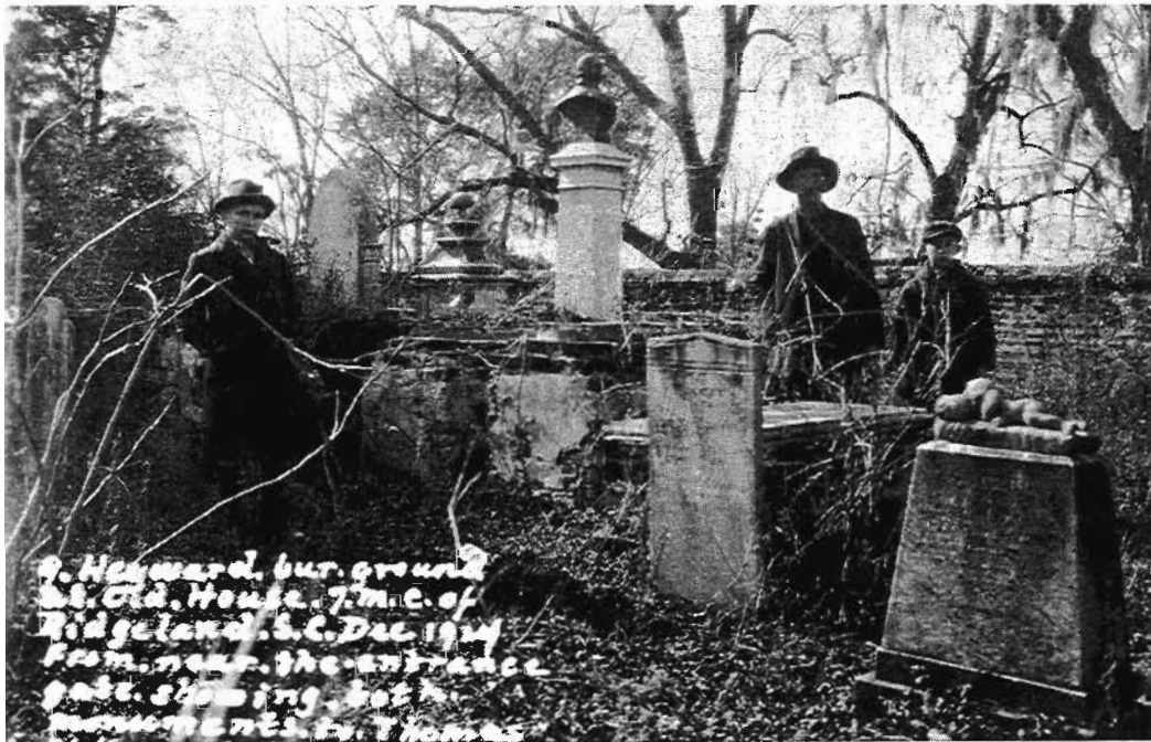
Figure 38. Thurston photograph of the Heyward Grave Yard "from near the entrance," taken in 1924.
