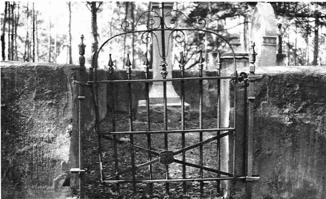
Figure 35. Close-up of the Stewart Iron Works shield on the inner gate, view to the north.
