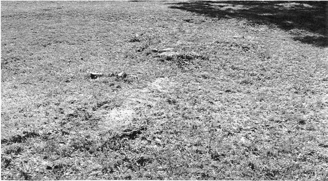
Figure 49. Brick foundation rubble associated with the main house between 203R190 and 203R220, view to the west-northwest.
