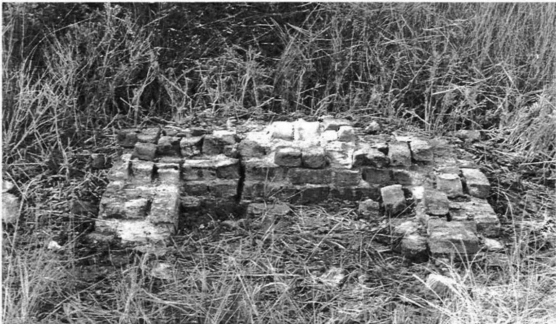
Figure 54. Marsh Structure 5, at the southeast edge of the site. View to the north.
