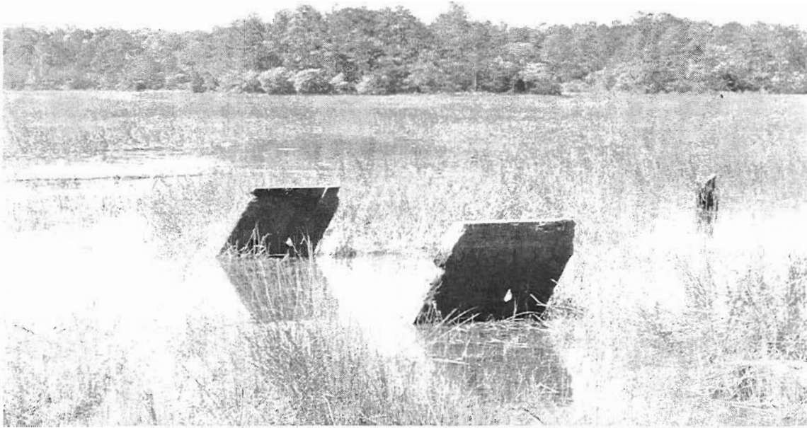
Figure 59. Brownstone flood gate supports south of the mill, view to the southeast. The photograph was taken at seasonal high tide.
