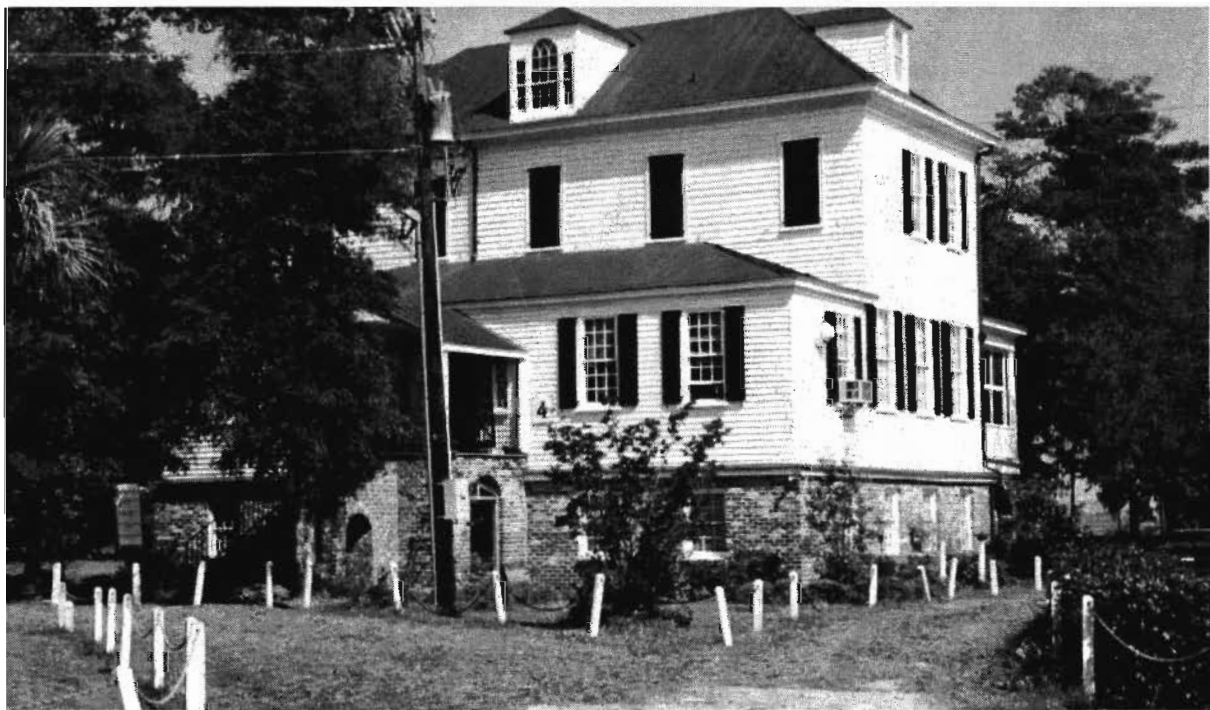
Figure 55. South facade of the Marshlands house.
