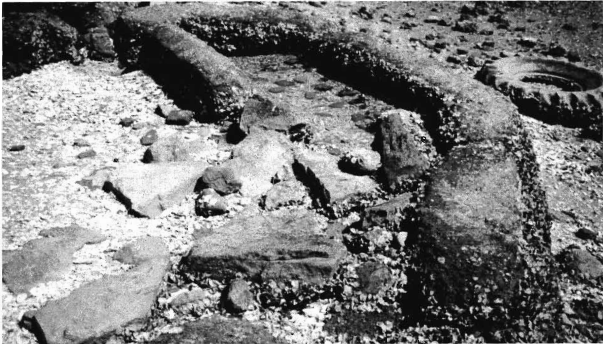
Figure 50. Bastionete at the east edge of Fort Johnson, exposed at low tide. Note erosion and debris.
