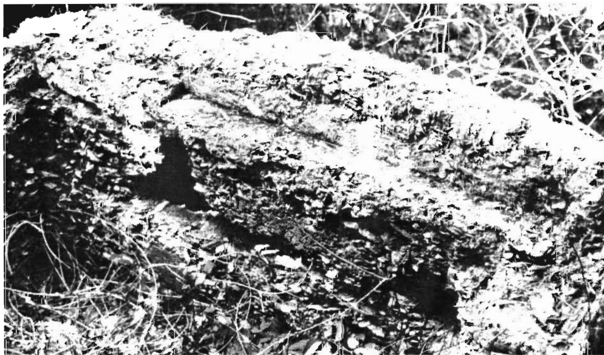
Figure 47. Interior wall of tabby structure at Area 6.
