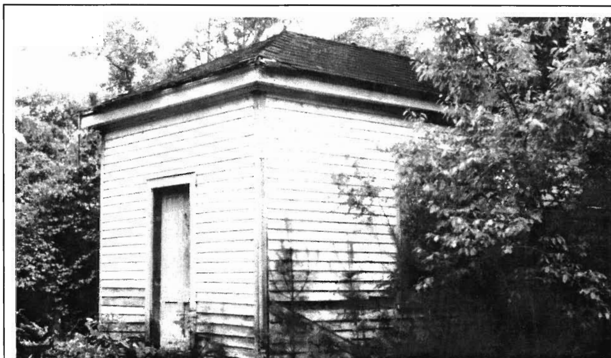
Figure 59. Pump House associated with ca. 1940 construction at Fort Johnson.
