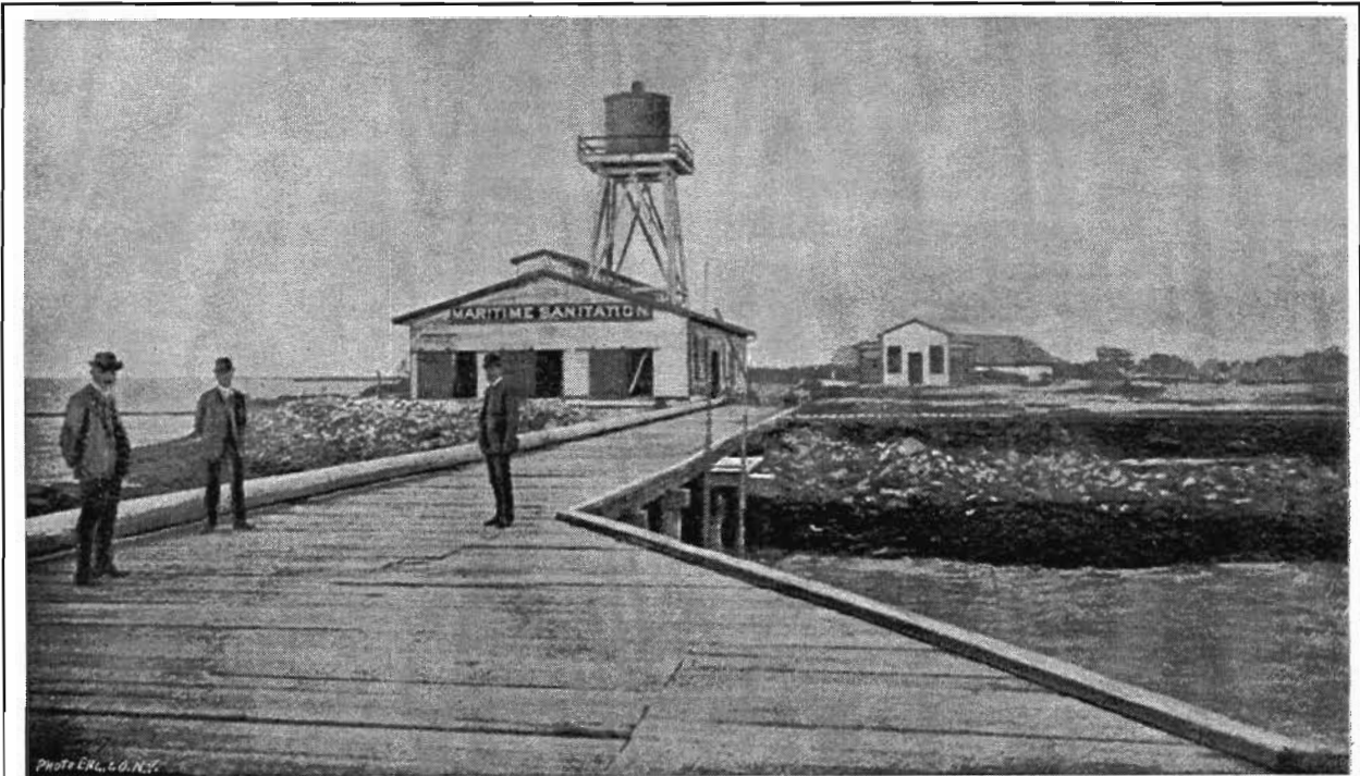
Figure 26. View of "maritime sanitation" buildings. To the right are the quarters for the ship's crew.
