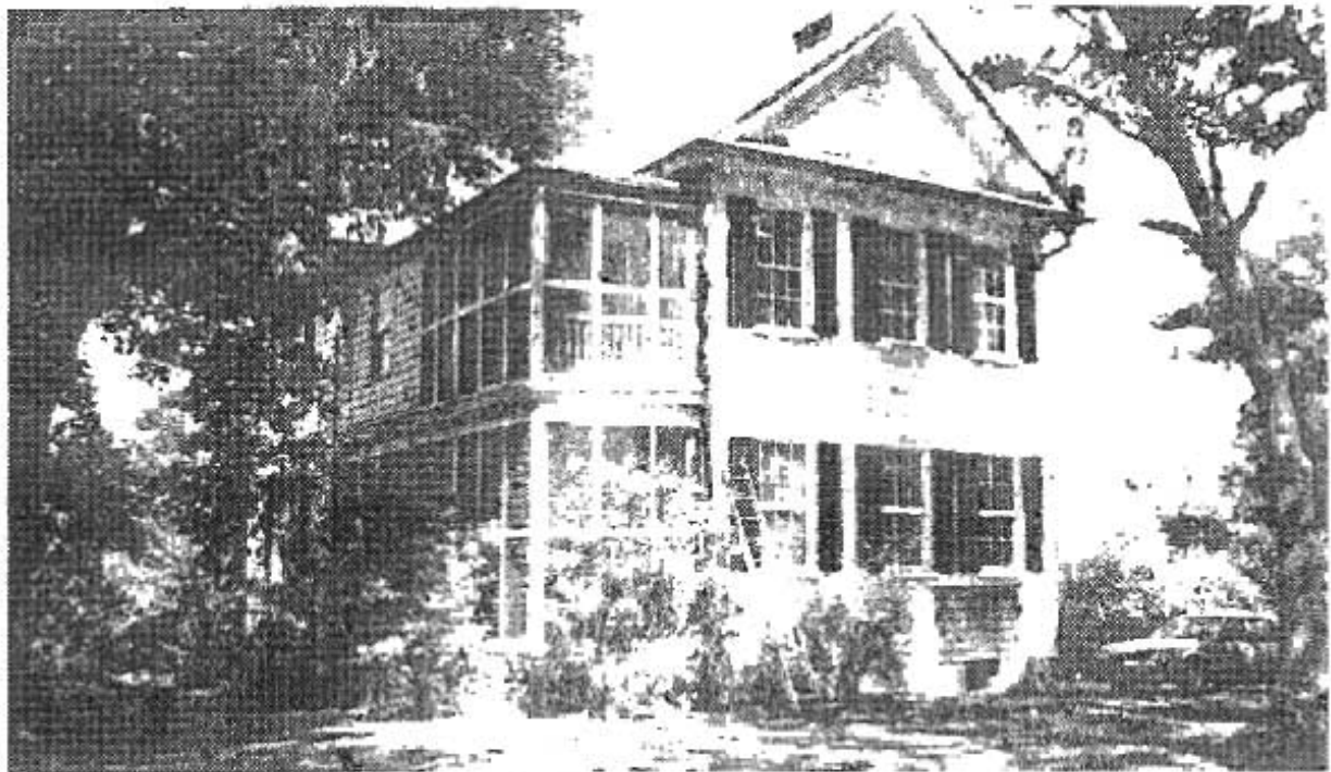
Figure 56. Quarantine Officer's House, view to the northwest.
