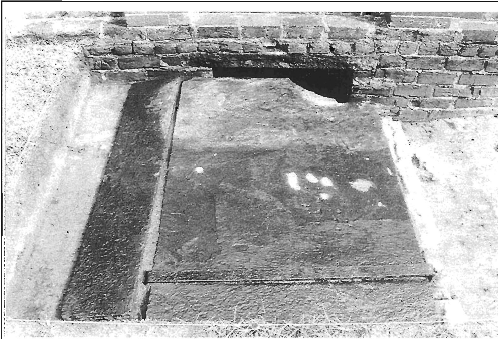
Figure 17. Units 2 and 3, view of slate cover with side slate removed and brick wall exposed. Tomb entrance is also exposed with the removal of the slate slab and concrete.
