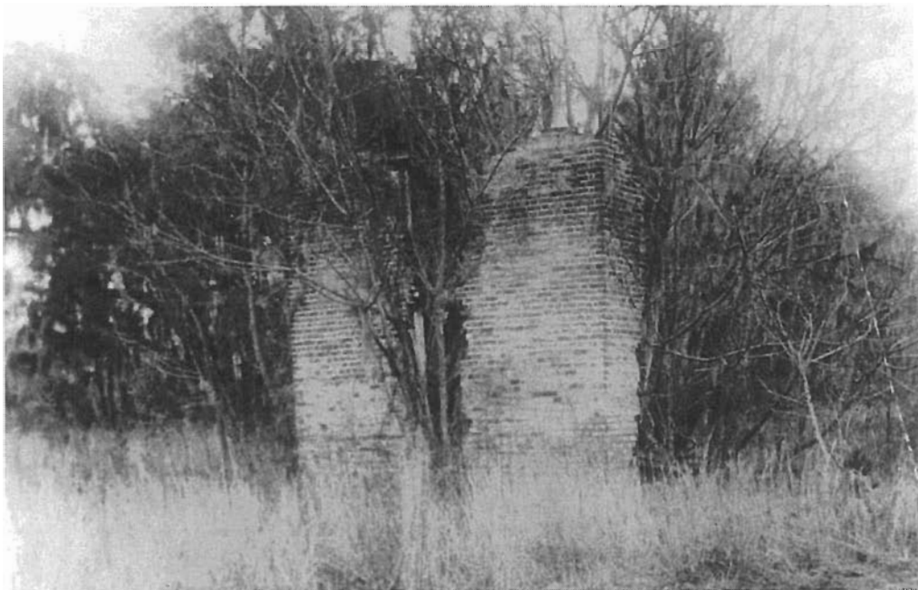
Figure 17. Photograph of the "ruins of out building to south of residence" at Broom Hall, taken in the 1930s (South Carolina Historical Society, William Henry Johnson scrapbook, 34-293/295).
