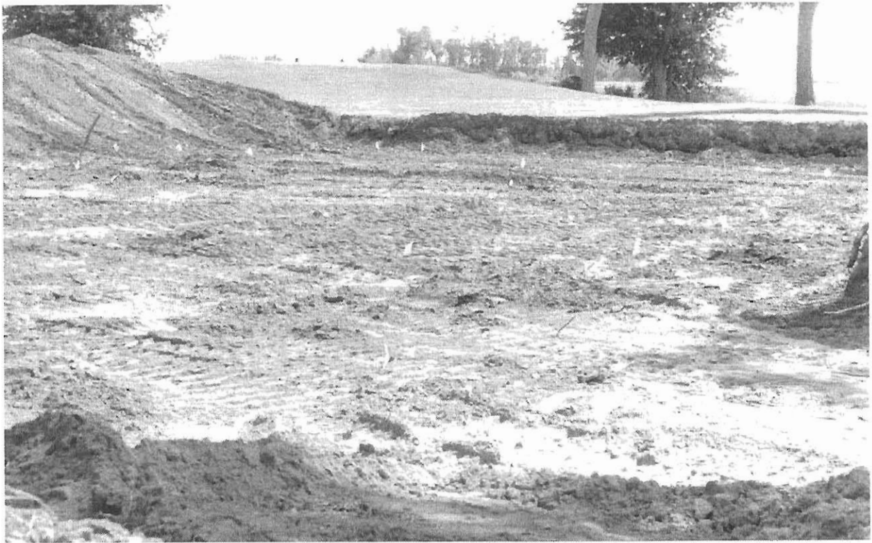
Figure 18. A portion of 38CH175 after stripping.
