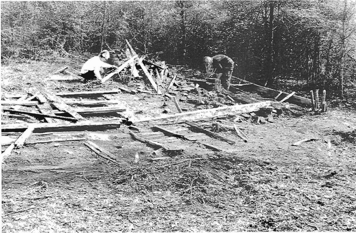
Figure 48. Exposing Structure 3 prior to excavation.
