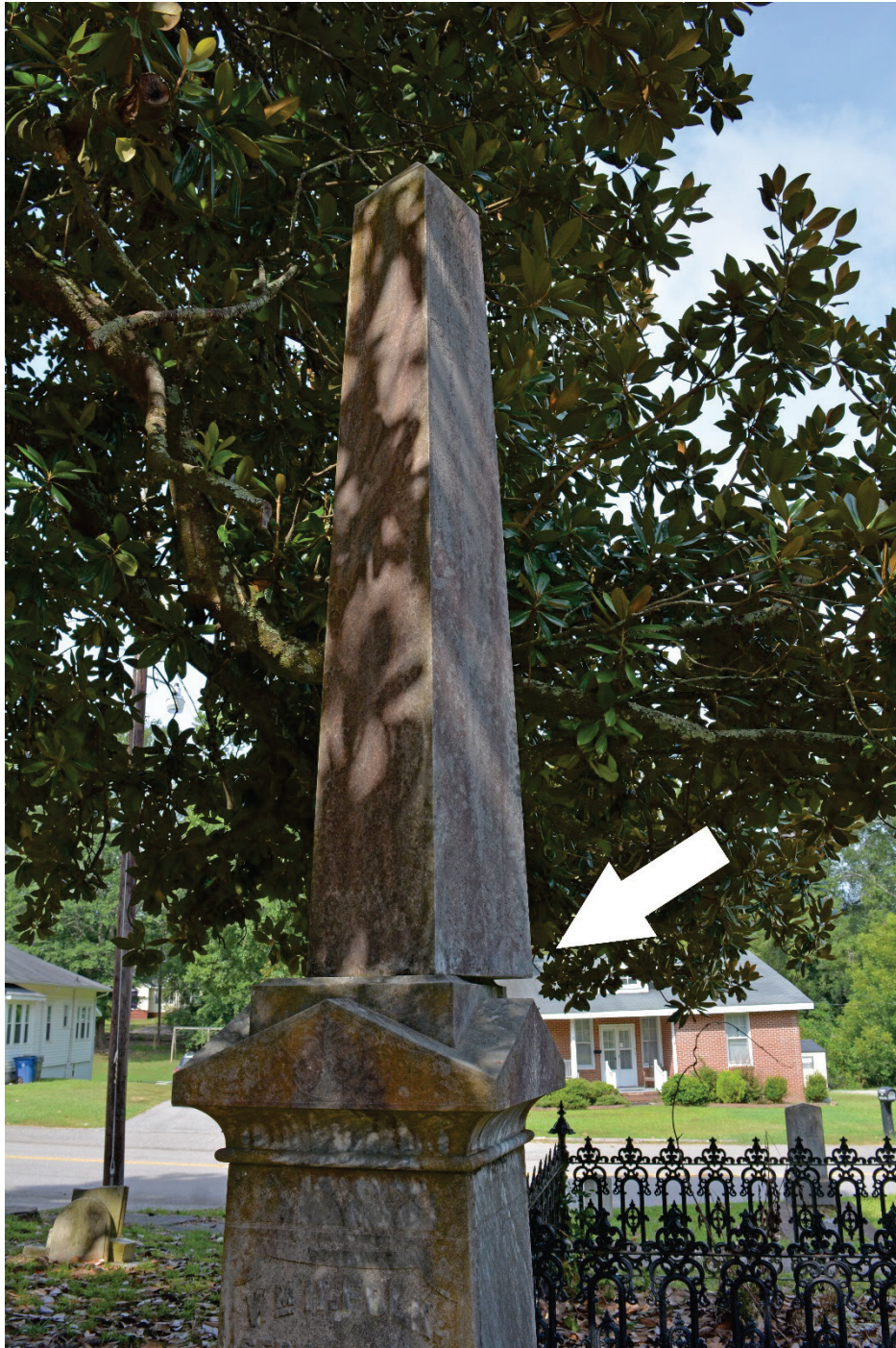
Figure 54. Extremely dangerous monument. This monument, which is clearly not pinned, has shifted on its base (note arrow) and poses a significant threat to the public.
