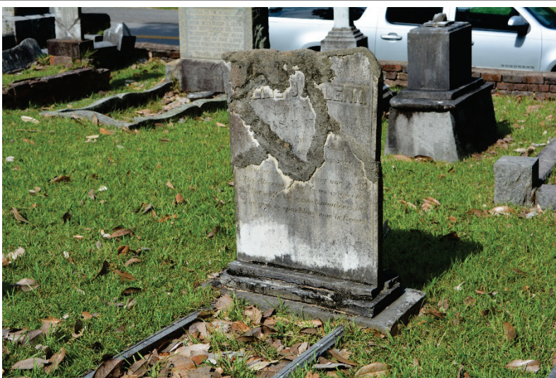
Figure 51. Very old repair using ordinary Portland cement (OPC). This is no longer an acceptable treatment option as the material is too hard for the marble.
