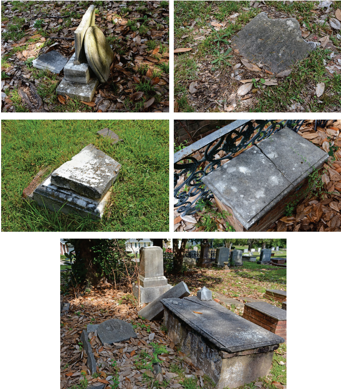
Figure 55. Broken stones. Upper left tab in socket is broken into three pieces and the tab was previously repaired using inappropriate OPC. Middle right shows a ledger cracked in two. The lower photograph reveals extensive damage. Not only is the obelisk toppled and broken, but its impact also broke the ledger and toppled an adjacent monument.
