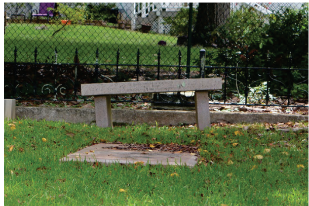
Figure 28. Benches in Willowbrook also require maintenance. The iron bench at the top requires securing to the fence or tree, as well as cleaning and painting. The granite bench below requires resetting to make it stable and safe.
