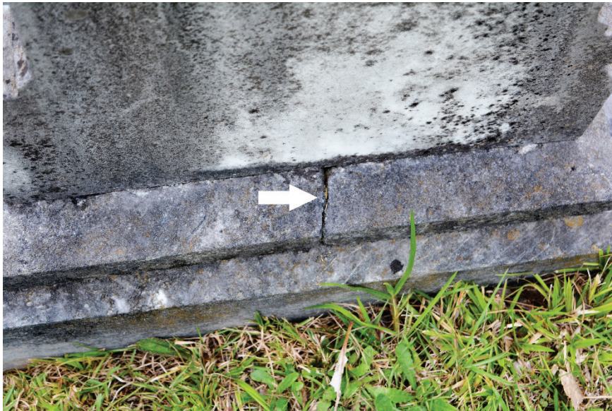
Figure 56. Example of iron jacking in the cemetery.
