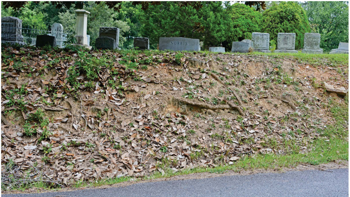
Figure 16. Erosion along Church Street. The upper photograph shows a section of failing brick wall with significant tree damage. The lower photograph shows a very steep soil bank.
