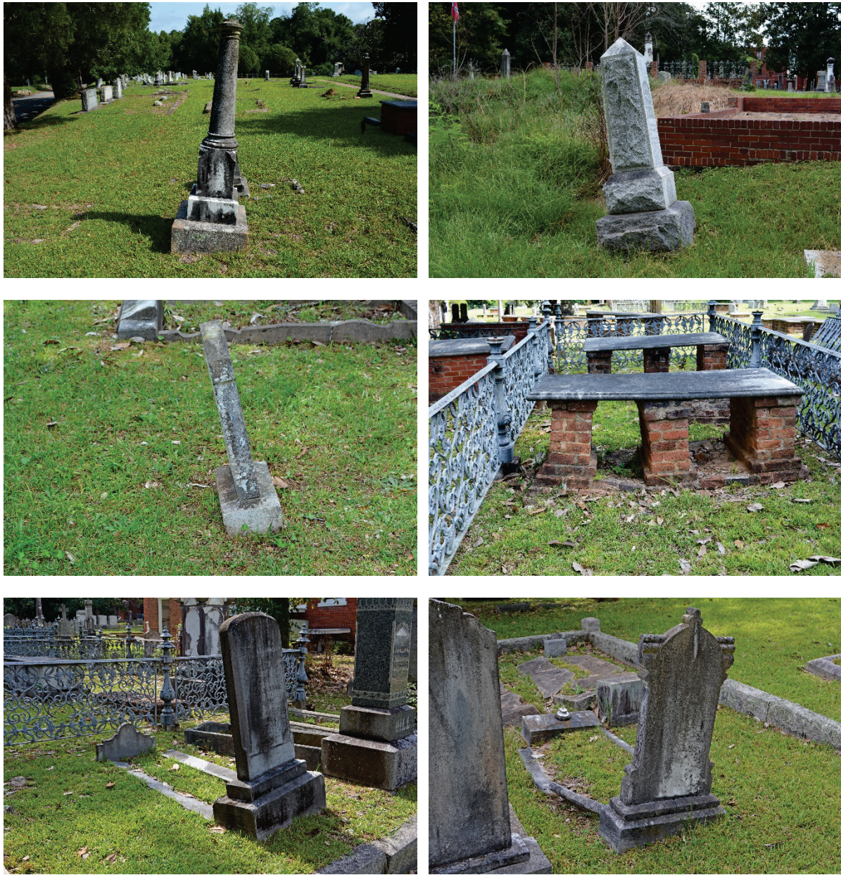
Figure 52. Examples of sinking and tilted monuments that require resetting, before additional (and more expensive) damage is done. Upper row photographs shows pedestal tombs with poor foundations sinking into graves. The middle left photograph is a simple die on base tilting into the grave. Middle right photograph shows a marble ledger beginning to bow as its supports collapse into the grave. Lower photographs show two cradle graves with collapsed sideboards and the headstone tilting.
