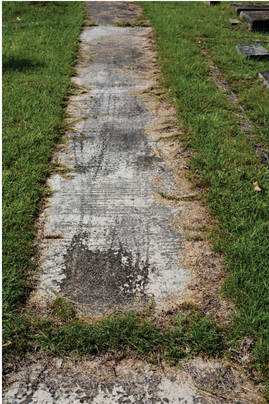
Figure 18. Concrete sidewalk showing its neglected condition with grass growing in cracks and mowed grass accumulating along the edges.
