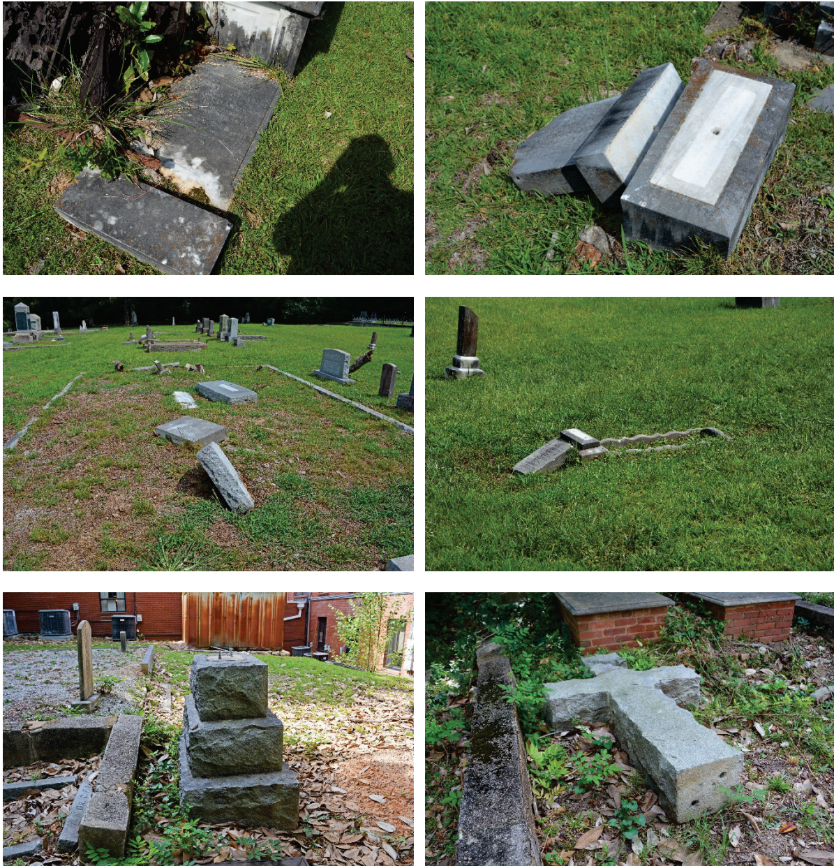
Figure 53. Fallen monuments. Upper row photographs show two die on base monuments that have fallen and require resetting with pins. The middle left photograph shows stones toppled by a tree. Middle right photograph is another toppled die on base. The lower two photographs show the large granite cross at the DeVore grave, likely toppled by vandalism or tree (based on the presence of still intact pins). The cross is now broken into three pieces, making the repair even more expensive.
