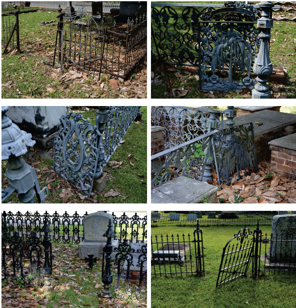
Figure 25. Examples of fence conditions. Upper left, gate no longer attached, post missing elements; upper right, gate and gate post no longer attached, iron jacking of granite foundation, missing elements; middle left, gate broken and elements missing; middle right, gate and gate post no longer attached, sections leaning; lower left, fence painted, but gate missing; lower right, fence painted, but gate no longer attached.
