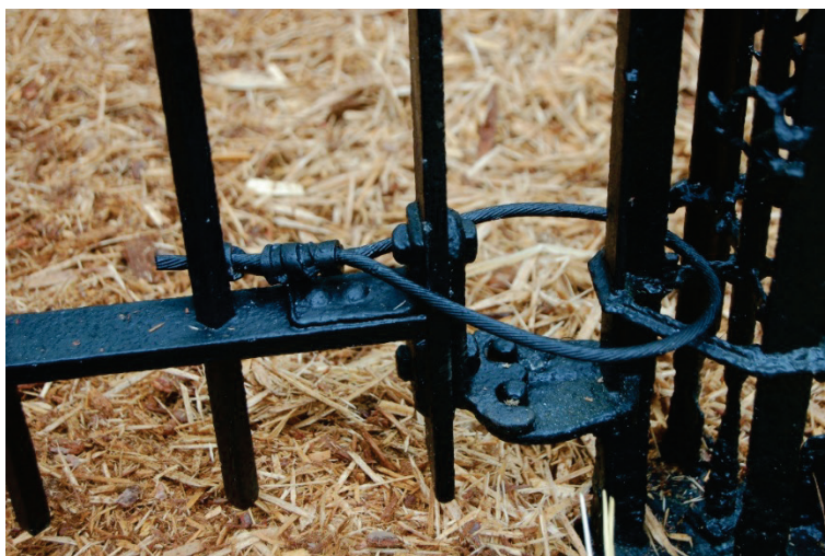
Figure 23. Example of a gate protected with stainless steel cabling that has been painted to blend with the fence.
