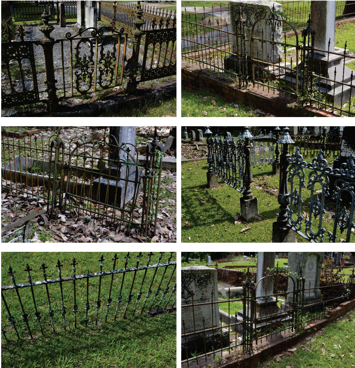
Figure 26. Examples of fence conditions. Upper left, cast and wrought fence in good condition, but it requires painting; upper right, mild steel fence in good condition, but it requires painting; middle left, mild steel fence with damaged gate and gate posts, that also requires paint; middle right, gate is missing, but fence is otherwise in fair to good condition; lower left, the fence bottom rail is buried in soil and requires resetting and painting; lower right, fence in good condition, but it requires paint.
