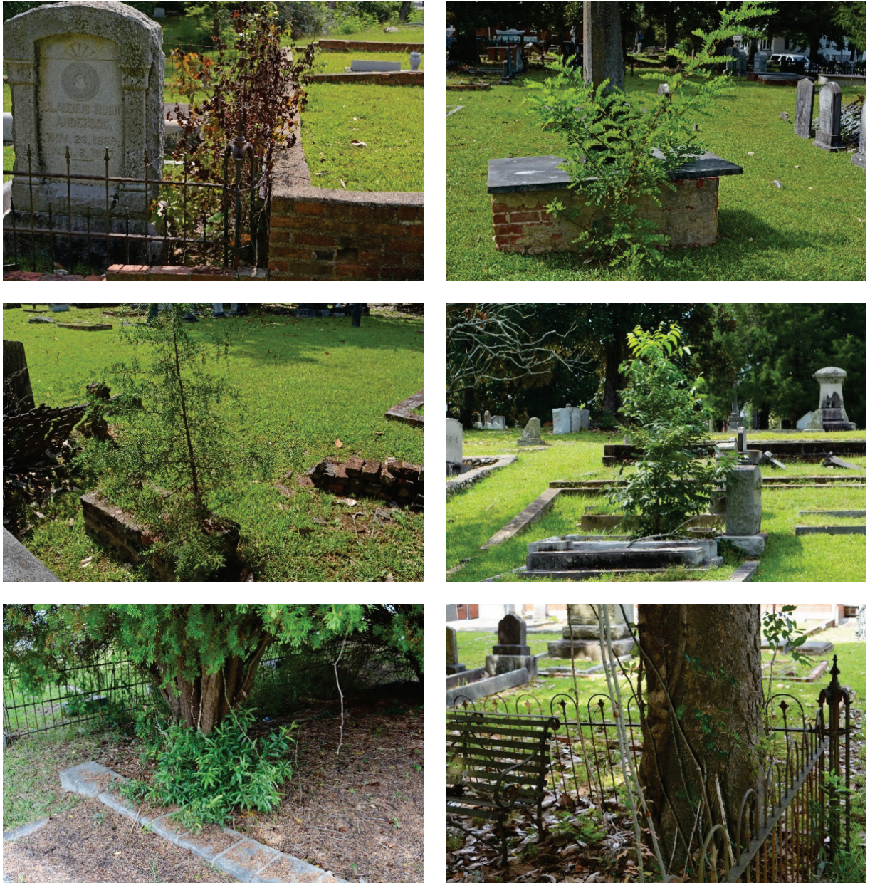
Figure 37. Tree problems. Upper left photograph shows trash vegetation growing up between a brick wall and iron fence. Upper right photograph shows a scrub tree immediately adjacent to a brick box tomb. Middle left photograph shows a bird-planted cedar growing up in a child's box tomb. Middle right photograph shows a trash tree growing up in a cradle grave. Lower left photograph shows scrub oak at the base of an arborvitae. Lower right photograph shows a tree that has been allowed to grow too close to an iron fence and is now impacting the stability of the fence.
