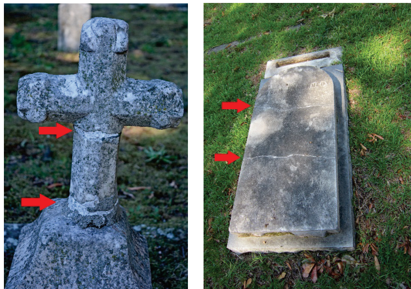
Figure 45. Examples of previous repairs in the cemetery. On the left is a cross with two breaks, probably repaired with a white Portland cement. On the right is a tab in base broken in two locations and missing its tab, laid flat on a OPC slab.
