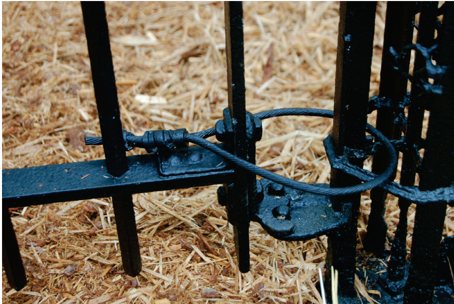
Figure 25. Example of a gate protected with stainless steel cabling that has been painted to blend with the fence.
