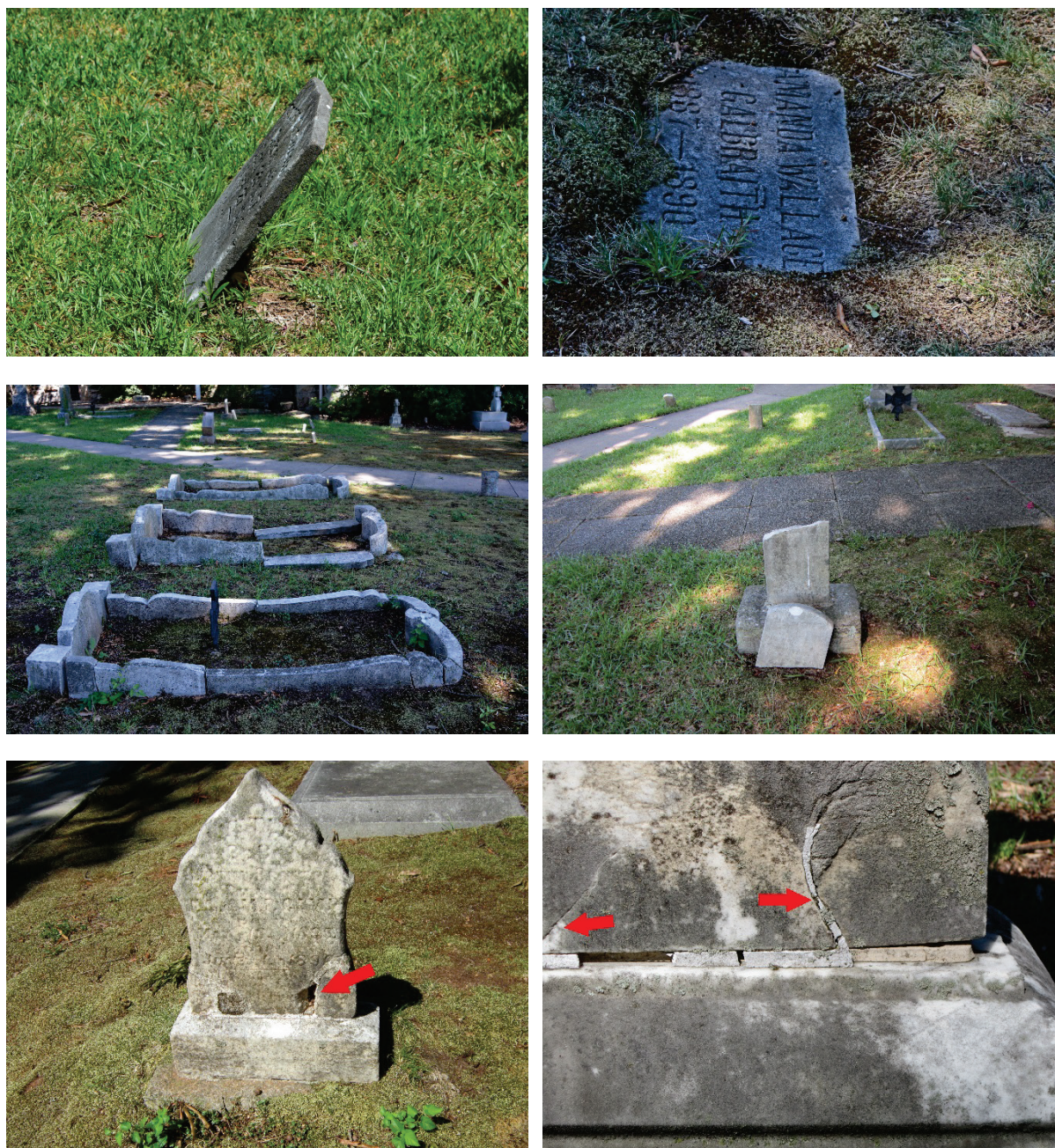
Figure 46. Examples of stones requiring conservation treatment. Upper row left shows a badly tilted stone. Upper right shows a sinking lawn marker. Middle left shows three cradle graves that are broken, displaced, and sinking. Middle right shows a broken tab in socket stone. The lower photos show two die on base markers attached using ferrous pins that have corroded and caused damage to the monuments.
