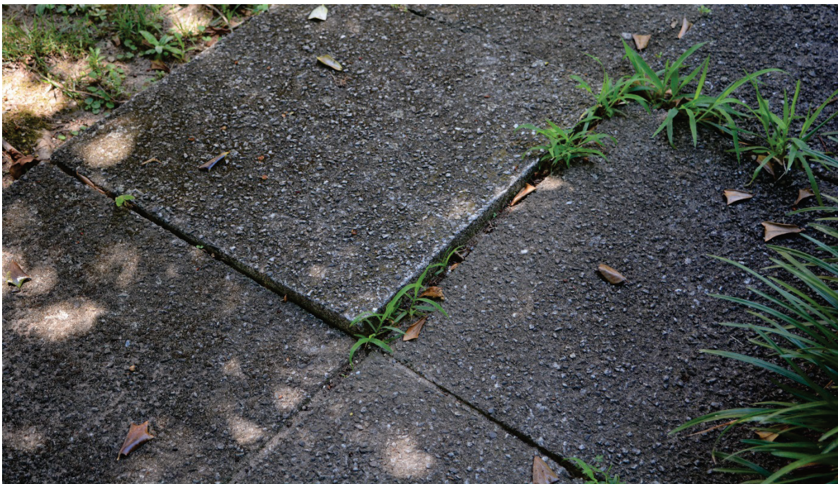
Figure 20. Poorly maintained paver pathway on east side of the cemetery. Many pavers pose a trip hazard and no effort has been made to control grass and weeds.
