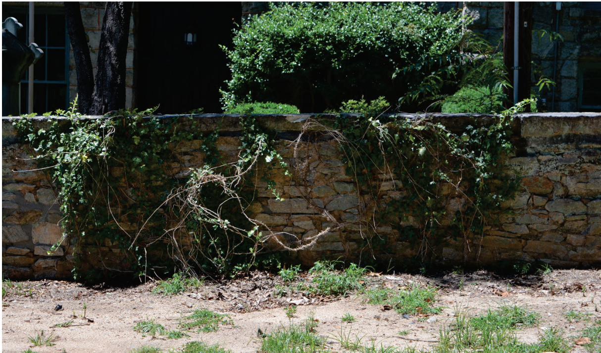
Figure 22. Stone wall along the east edge of the cemetery. Upper photo shows the three courses of random rubble. The lower photo shows heavy vine growth that must be removed.
