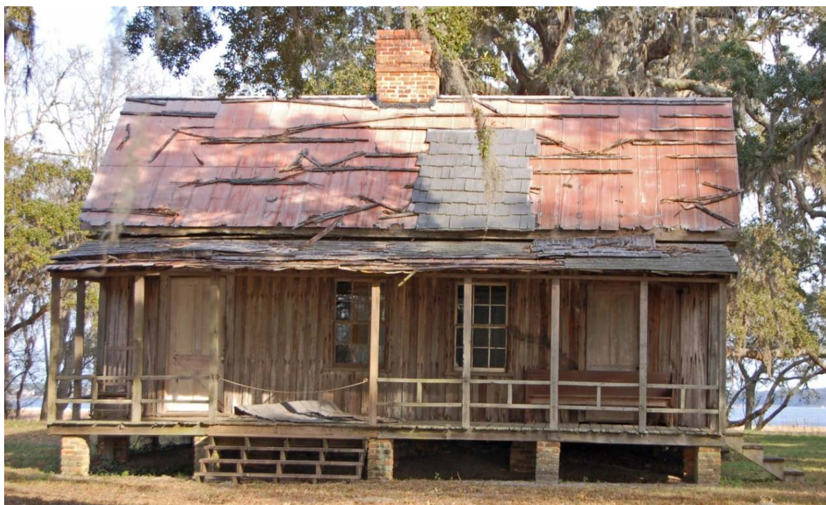
Figure 7. Standing structure at 31BW787**7. Top photograph is an oblique view to the southeast. Below is a view of the front, looking east.
