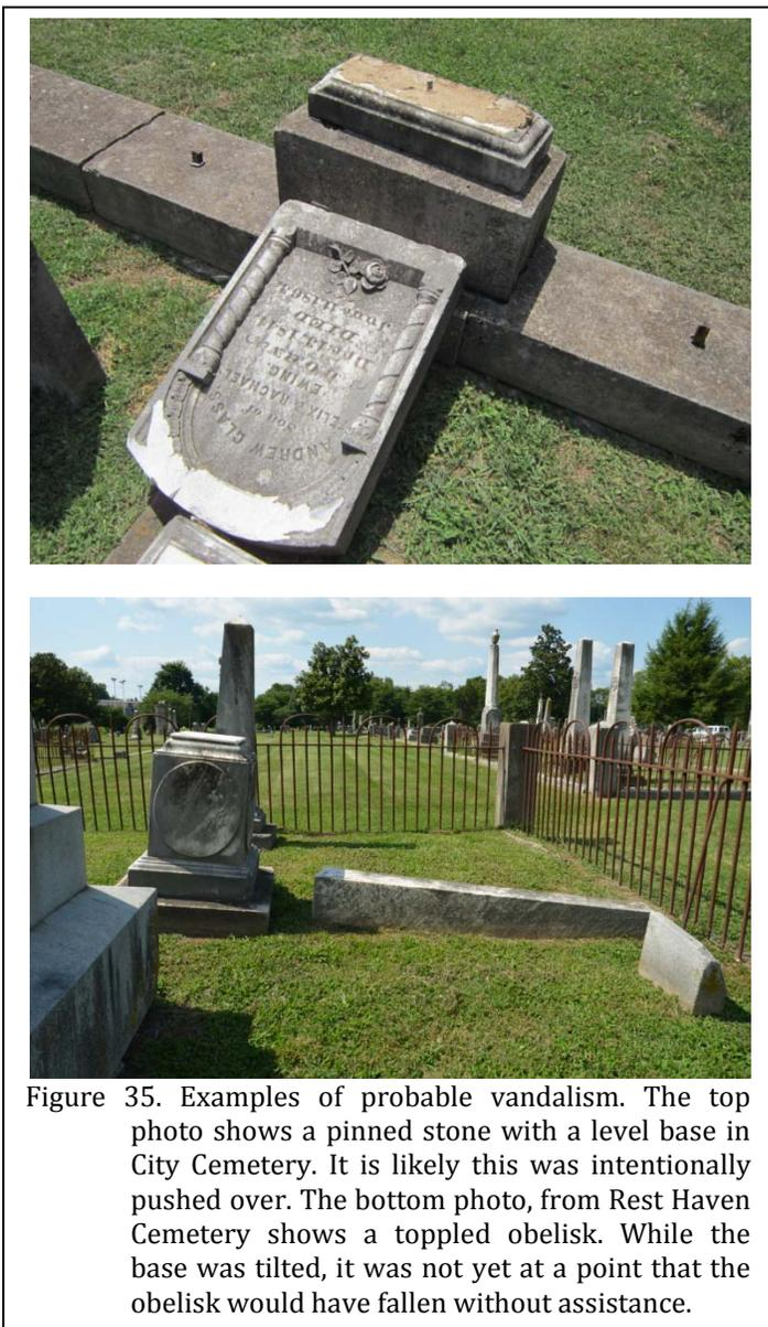
Figure 35. Examples of probable vandalism. The top photo shows a pinned stone with a level base in City Cemetery. It is likely this was intentionally pushed over. The bottom photo, from Rest Haven Cemetery shows a toppled obelisk. While the base was tilted, it was not yet at a point that the obelisk would have fallen without assistance.
