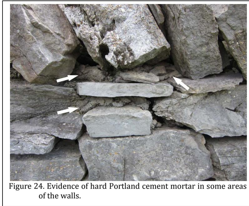
Although the wall is typically called dry laid (see, for example, Tyler and Coffing (2006:4), there are many portions with large amounts of a hard Portland cement mortar (Figure 24). It is not known if this extends throughout the length of the wall or only reflects recent, inappropriate repairs.
