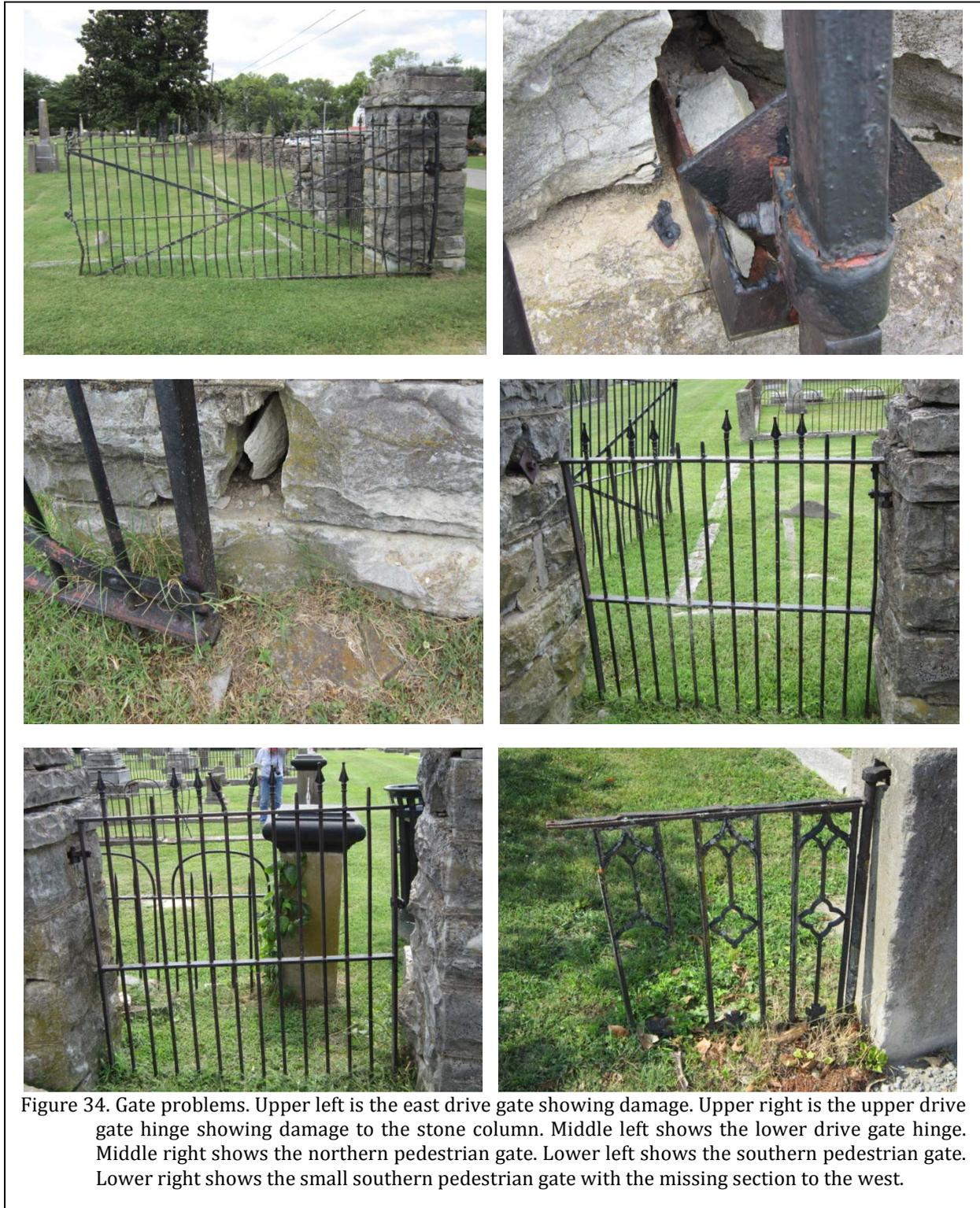
Four finials are missing and two pickets are bent. The hinges appear sound, although there is no closing/locking mechanism present.
