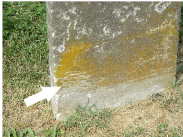
Figure 57. Examples of nylon string trimmer damage at Rest Haven Cemetery.
