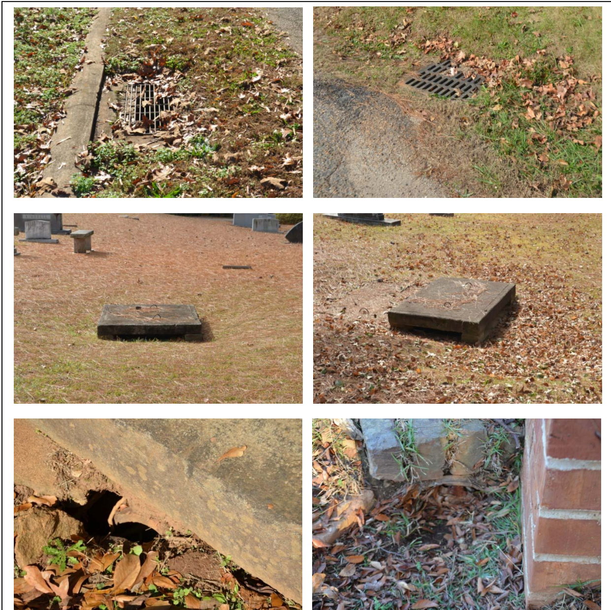
Figure 104. Cemetery below grade drain problems. Upper left photo shows a below grade drain along River Road. Upper right photo shows a below grade drain at the edge of the road in Section H. Middle left photo is a below grade drain in the middle of Section H. Middle right photo is another below grade drain in Section H. Lower left photo is a below grade drain in the Valley Section, largely obscured by a set of stairs. This drain is at least 75% clogged. The lower right photo shows a below grade drain in the West Hill Section that is at least 90% clogged.
