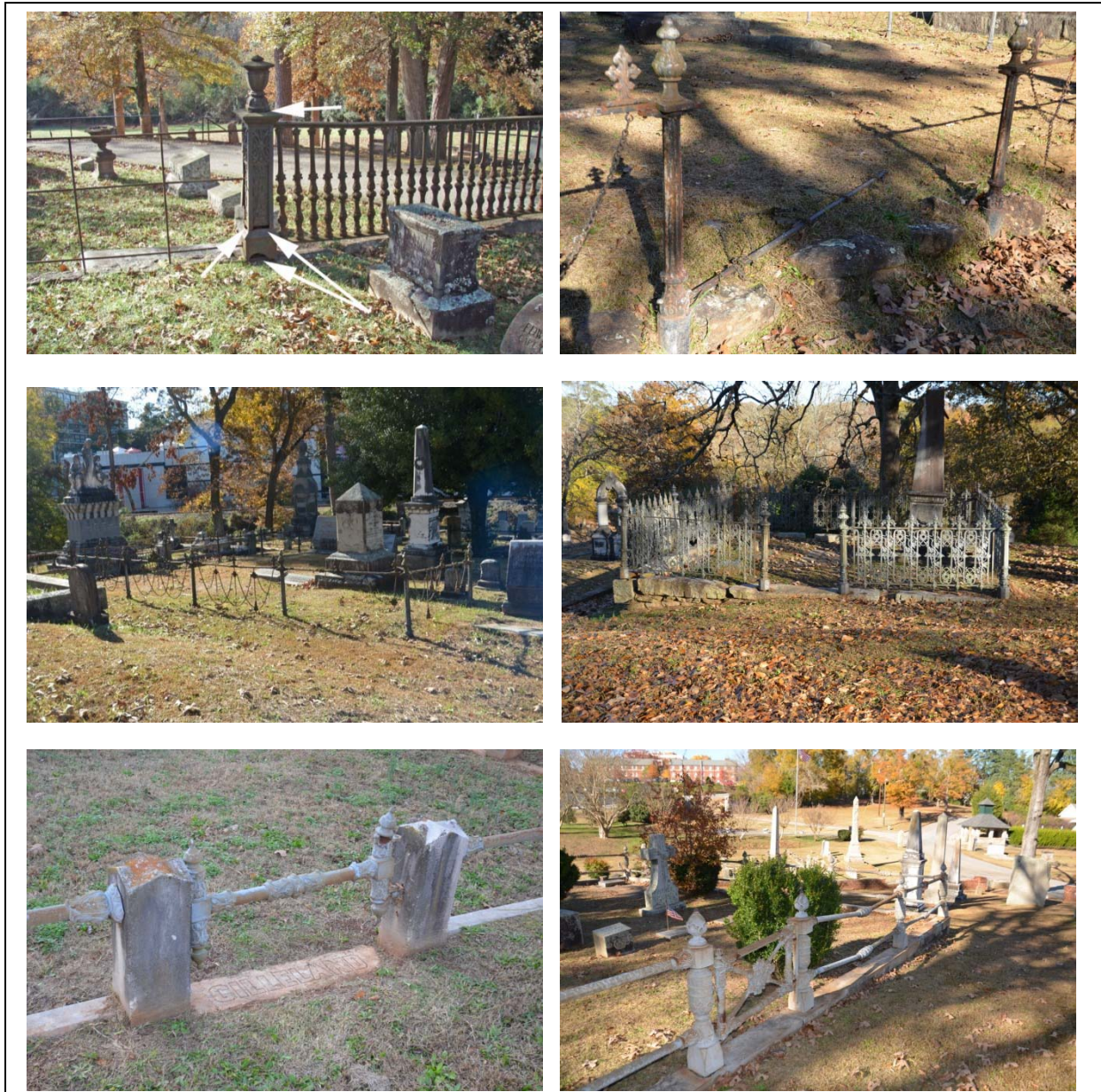
Figure 122. Fence types and common problems at Oconee Hill Cemetery. The upper left photo shows an iron fence in East Hill that has made good use of a “ghost” section to provide support and enclose the lot with minimal expense. The arrows, however, point to areas where water is entering the fence and causing damage. The upper right photo shows a fence in poor condition with parts lying on the ground. The middle left photo shows an iron fence in fair condition. The middle right photo shows an iron fence that had been painted white, but is now in failing condition. The lower two photos show typical gas pipe fences with corrosion breaking through the galvanized coating.
