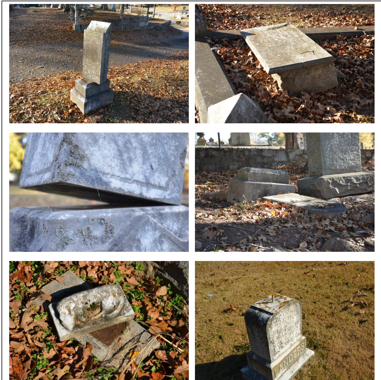
Figure 114. Examples of loose or fallen monuments. The upper left photo shows a monument twisted on its base and ready to collapse. The upper right photo shows a ledger loose and displaced on its box tomb. The middle left photo shows how easy it is to tip over a monument that is not pinned to its base. The middle right photo shows an unpinned monument that has fallen in the Cemetery. The lower left photo shows a lamb decoration loose on its stone. This could be easily stolen and is the type of monument sought for garden decoration. The lower right photo shows a monument that has lost its urn already. Note the pin is still in place.
