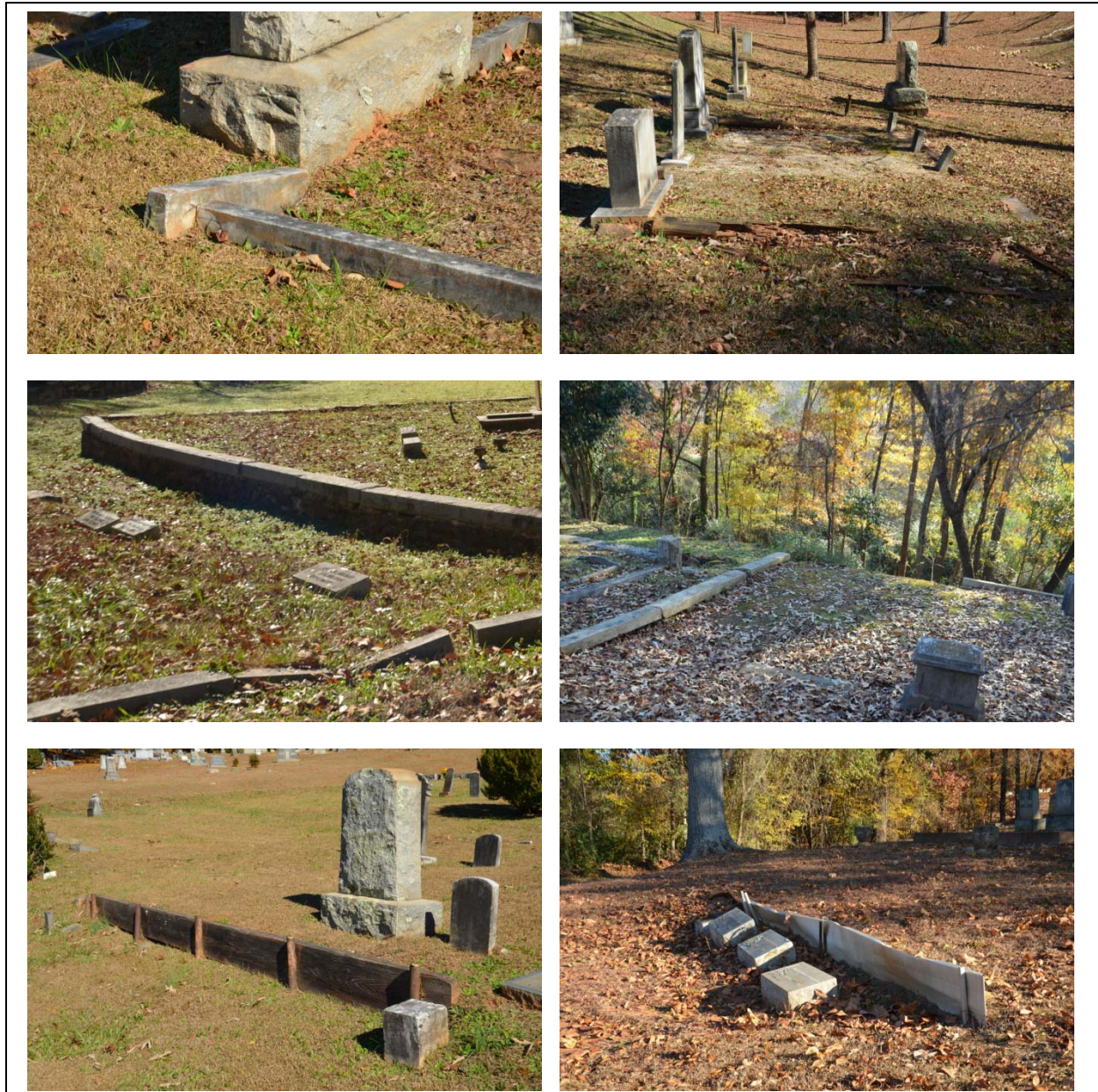
Figure 109. Plot curb issues in the Cemetery. The upper left photo shows displaced marble coping sinking into a grave. The upper right photo shows badly deteriorated wooden railroad tie curbs. The middle left photo shows broken and sinking concrete curbing. The middle right photo shows the loss of curbs over the side of a slope due to unrestrained erosion. The lower left photo shows a wood board, held by pipes that is apparently being used to control sheet erosion. The lower right photo shows a similar situation where metal skirting or siding panels have been similarly used.
