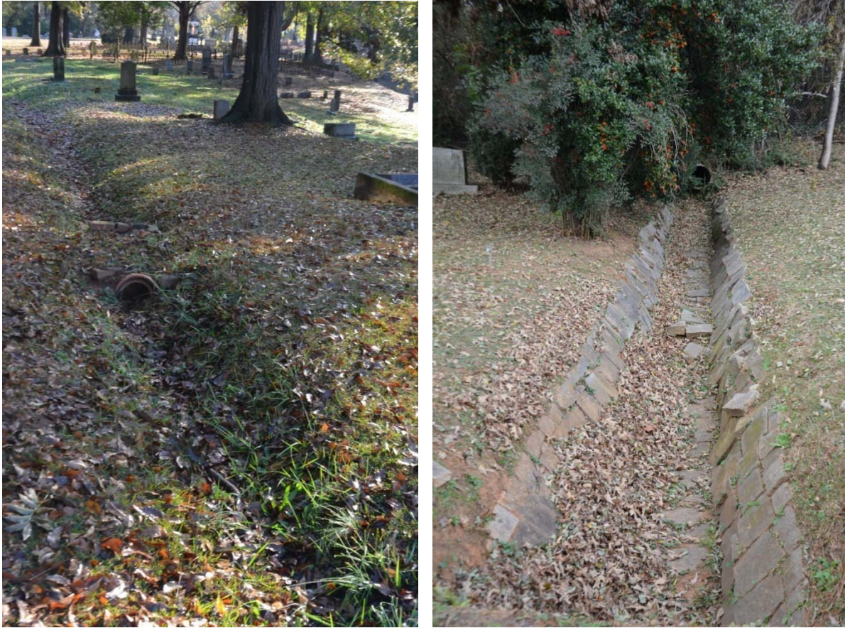
Figure 103. Cemetery surface drain problems. The upper left photo shows drainage ditch and culvert along the road of Factory Section that is not maintained. The upper right photo shows a surface drainage ditch that runs from off the cemetery property through Old G Section to a below grade drain. This drain requires cleaning and repair of the rock facing.
