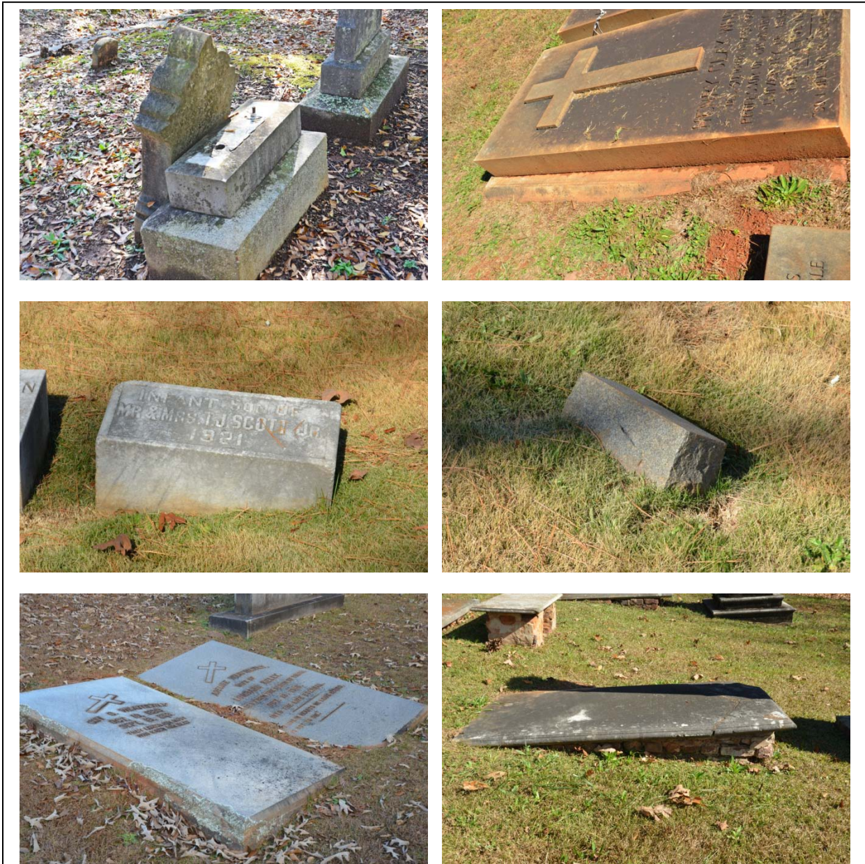
Figure 112. Displaced or sunken monuments. The upper left photo shows a die on base that has fallen off and requires resetting. The existing pins may need to be replaced. The upper right photo shows a granite ledger displaced off its base, probably by a mower. The middle left and right photos show monuments sinking into their graves for lack of a good foundation. The lower left photo shows a very large granite ledger sinking into a grave. The lower right photo shows what appears to be a brick box tomb that has sunk out of sight at one end, while the other is still partially supported by remnant bricks.
