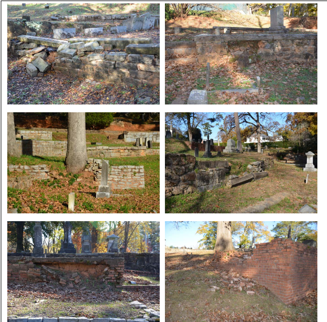
Figure 119. Examples of walls requiring repair or replacement. Damage has resulted from foundation settling which causes diagonal cracking through masonry units or the bed joints; displacement of walls, at times by out-of-plane loading, but more often by pressure resulting from trees; or failure to maintain the walls (including a lack of pointing).
