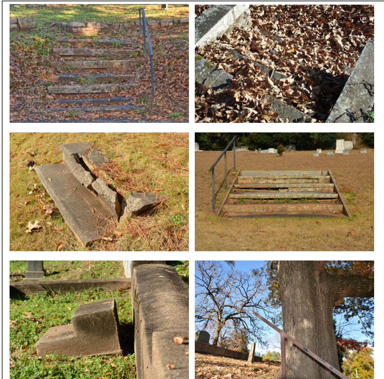
Figure 35. Stair and handrail problems. The upper left photo shows stairs with different height risers and treads of various widths. The upper left photo shows the hazard resulting from the failure to clean stairs on a regular basis. The middle left photo shows hazardous concrete stairs with extensive deterioration. The middle right photo shows stairs with damaged risers that are allowing grass to grow. Lower left photo shows stairs that have sunk into a lot, presenting a significant hazard to users. The lower right photo shows a handrail that poses a penetration hazard to pedestrians who might lose their footing on the steep slope leading to the stairs. Many of these issues require immediate intervention.
