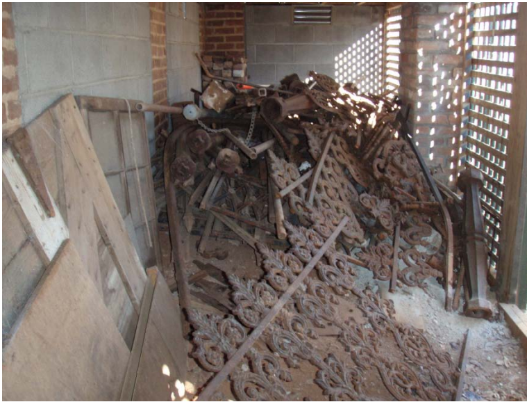
Figure 39. Storage under the Sexton's Cottage. This area must be cleaned and better organized.
