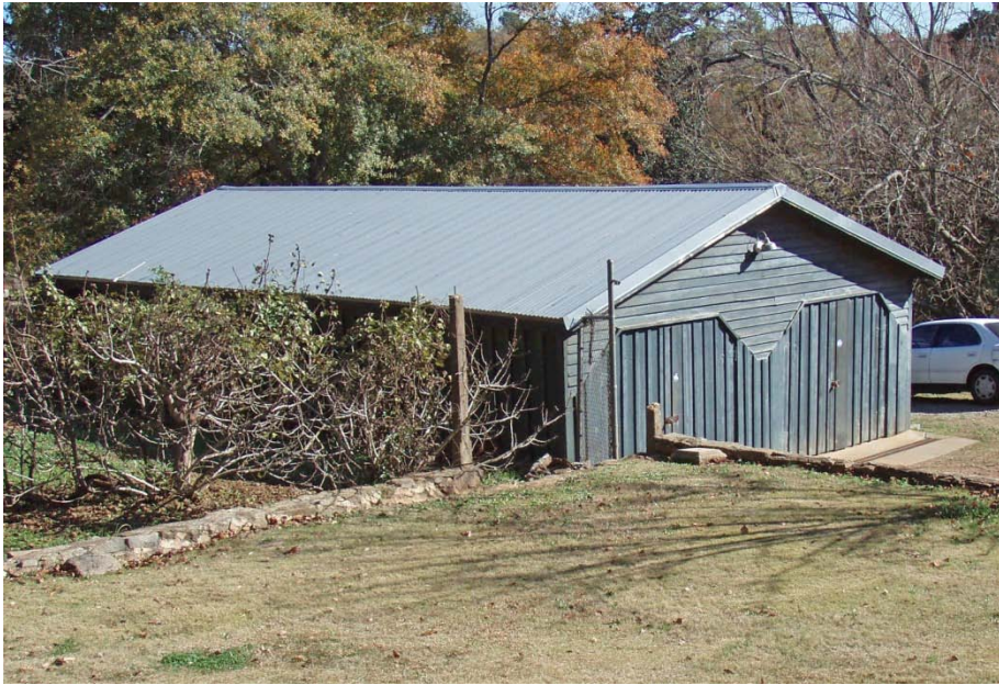
Figure 43. Oblique view of the maintenance building, looking southeast.
