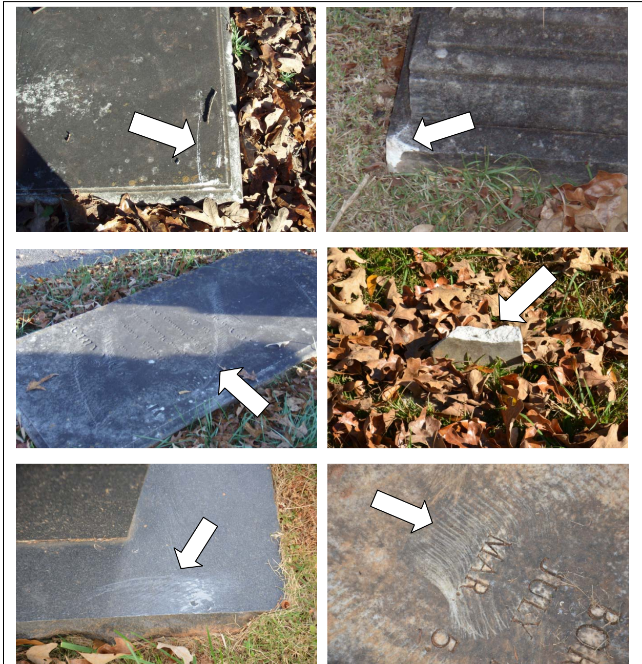
Figure 76. Damage to stones resulting from inappropriate mowing techniques. The upper left photo shows blade damage to a marble ledger. The upper right photo shows edge damage to a marble base. The middle left photo shows tire tracks across a marble ledger. The middle right photo shows a scalped marble footstone. The lower left photo shows scraping of polished granite. The lower right photo shows blade damage to a marble ledger.
