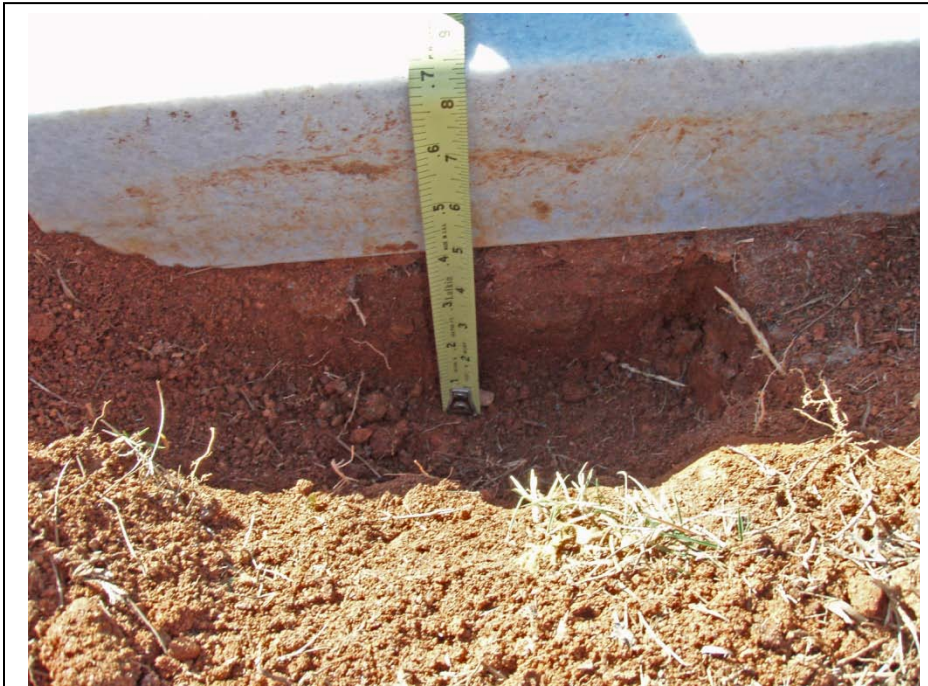
Figure 108. Monument set in 2013 showing virtually no concrete foundation – only clay soil. Scale is in tenths of feet on the left and inches on the right.
