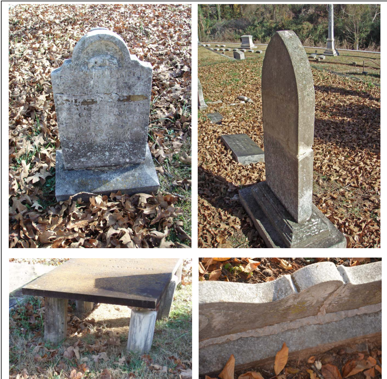
Figure 110. Examples of incorrect and poor repair practices at Oconee Hill Cemetery. Upper left shows a stone with a simple epoxy repair. The epoxy has been used as infill and has yellowed through UV exposure. Upper right is a repair using some type of mortar that has been smeared across the face and sides of the stone. There is also loss along the edge. The lower left photo shows a table tomb with a sunken leg that has been “fixed” by inserting a brick fragment in an effort to level it. The lower right photo shows a damaged marble monument repaired using some type of caulk.
