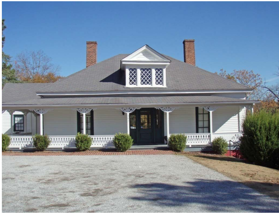
Figure 38. Front façade of the Sexton's Cottage, looking east.
