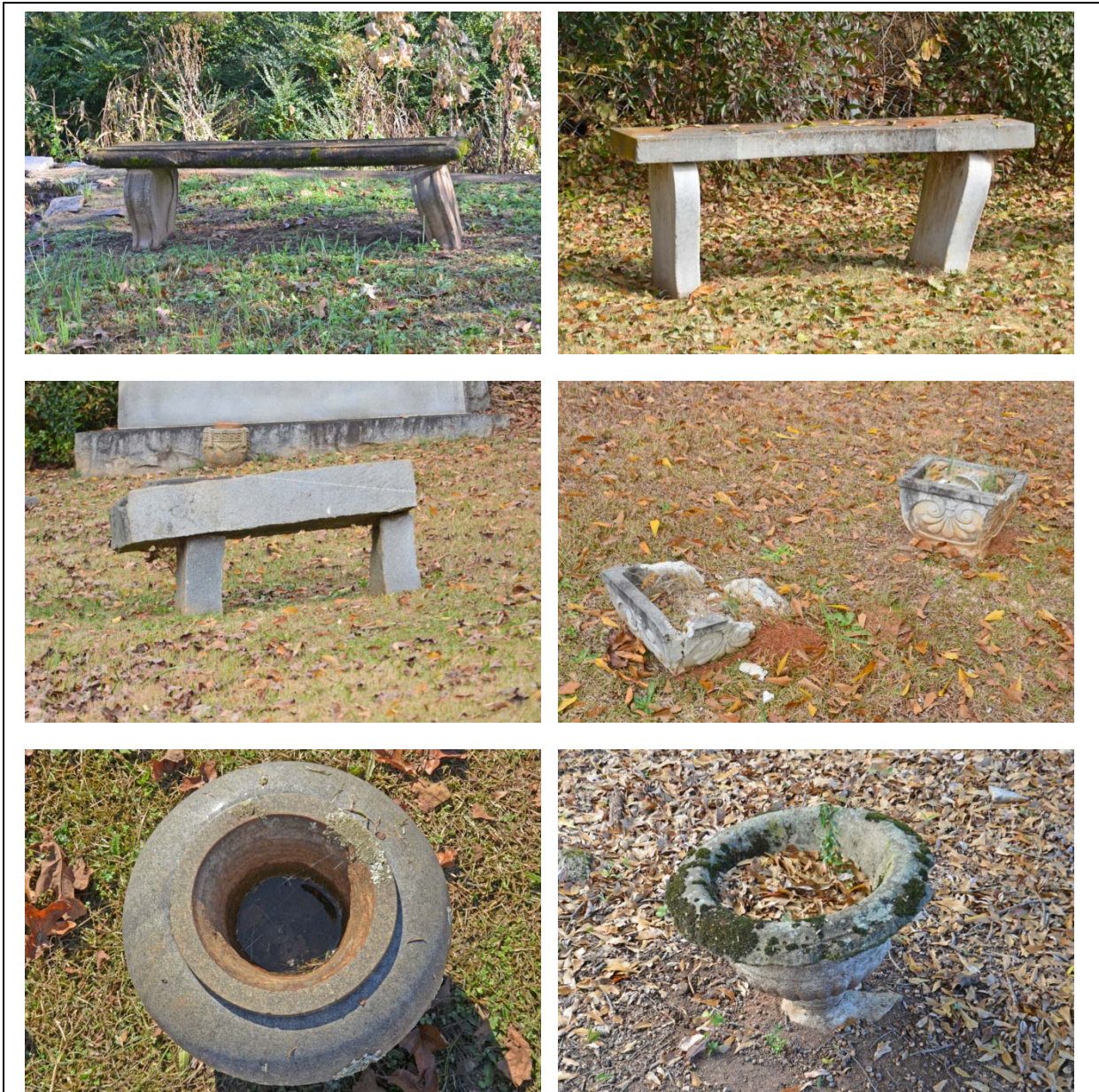
Figure 60. Bench and urn problems in the cemetery. The upper row shows two unsafe, poorly supported benches, one concrete and the other granite. The middle left photo shows a poorly set granite bench that is a safety hazard. Middle right photo shows two concrete urns, neither of which are planted. The urn on the left shows typical freeze-thaw deterioration and should be removed. The urn on the right is filled only with trash. The bottom left photo shows a polished granite urn that is partially filled with water. The bottom right photo shows a marble urn that is filled with trash and debris and which is settling in the ground.
