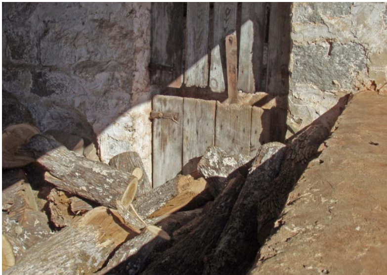
Figure 42. Animal pen. The upper photo shows the animal pen with a shed roof. To the left is the raised bed garden. The lower photo shows logs thrown into the pen – these must be removed. Note also the original hardware.
