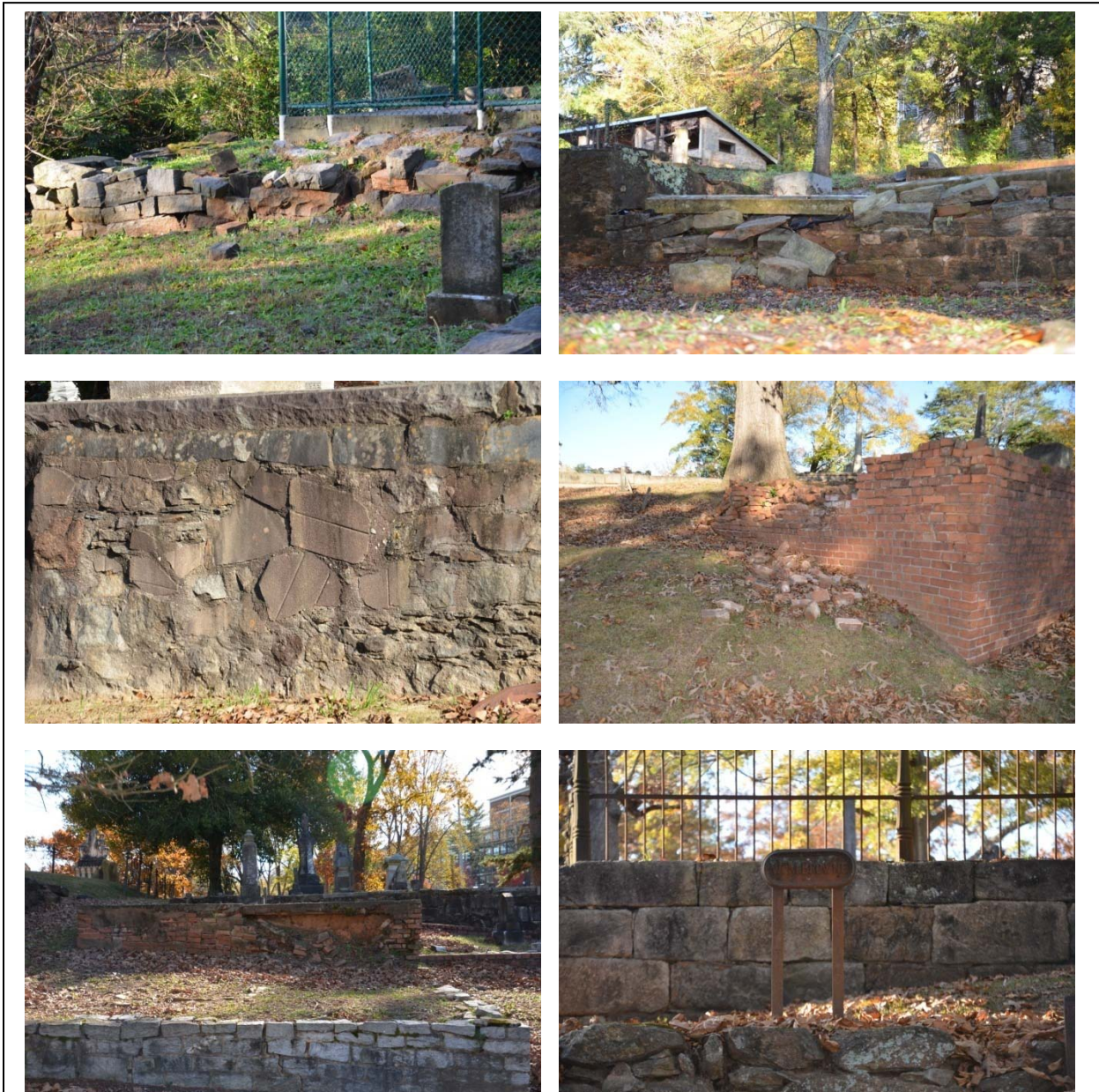
Figure 118. Variation in wall designs. Upper left photo shows a dry laid wall of pitched-face granite in Factory Cemetery (wall is in failure). Upper right is a coursed rubble granite mortared wall in Factory Cemetery (in failure). Middle left photo shows a mortared random rubble wall in West Hill that is in good condition. Middle right photo shows a brick wall in West Hill laid up in running bond, although there are two courses of headers at irregular intervals. This wall is in poor condition. The lower left photo shows a mortared coursed rubble wall (bottom) in West Hill (wall is in good condition). Lower right photo shows a squared rubble wall laid in mortar in West Hill (wall is in good condition).
