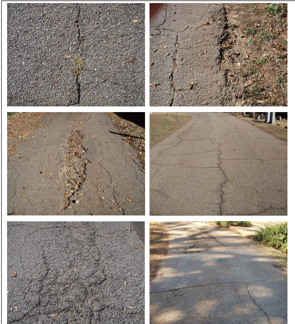
Figure 28. Typical road conditions at Oconee Hill Cemetery. Upper left photo shows a longitudinal crack with grass growing in the crack. Upper right photo shows pavement edge damage. Middle left photo shows an unrepaired pothole. Middle right photo illustrates longitudinal and transverse cracks. Note how water is retained in the cracks, causing further damage to the underlying base. Lower left photo shows raveling. Lower right photo shows a permanent patch.
