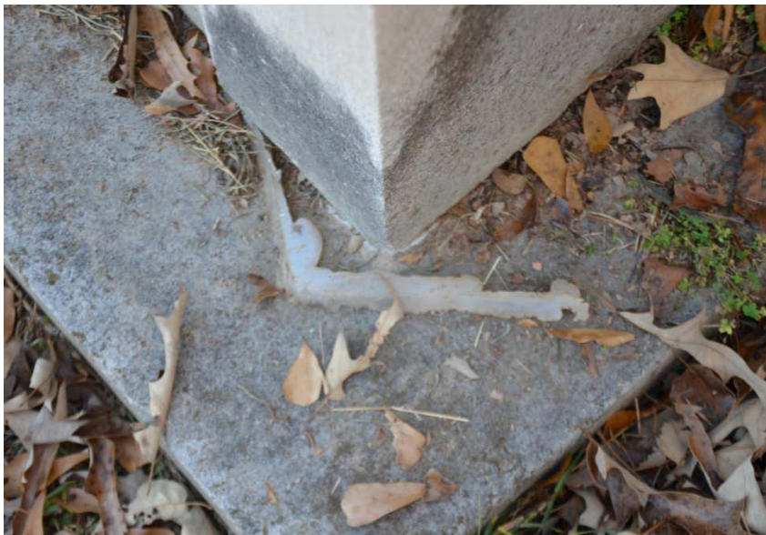
Figure 56. Silicone caulk that has failed on the Glenn Mausoleum in West Hill.
