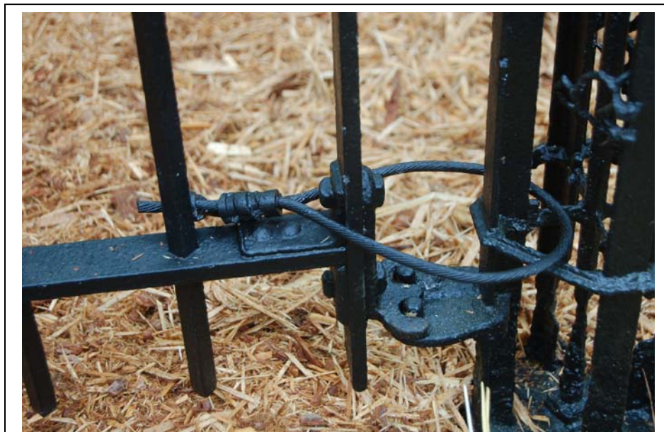
Figure 55. Example of a gate protected with stainless steel cabling that has been painted to blend with the fence.
