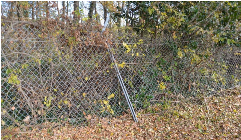
Figure 53. Fence damage, including fallen trees, overgrown fences, and collapse, that requires repair.
