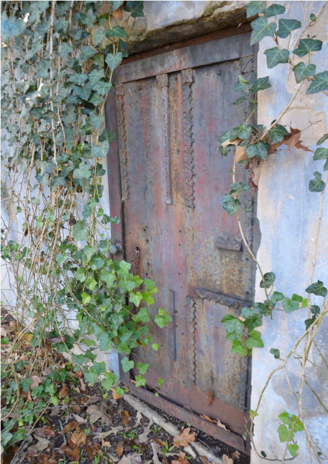
Figure 49. Holding vault. Photo of the badly damaged vault door.
