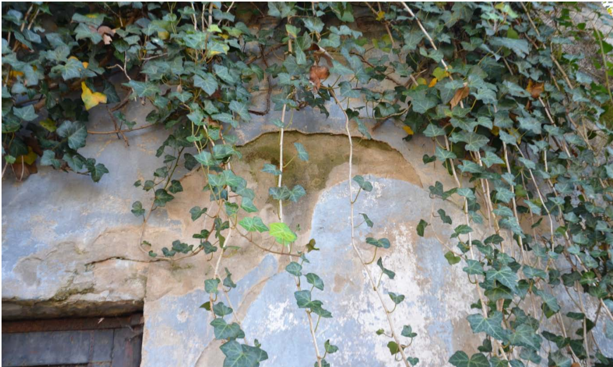
Figure 48. Holding vault. The upper photo shows the overall tomb condition. The lower photo shows spalling stucco and water damage.
