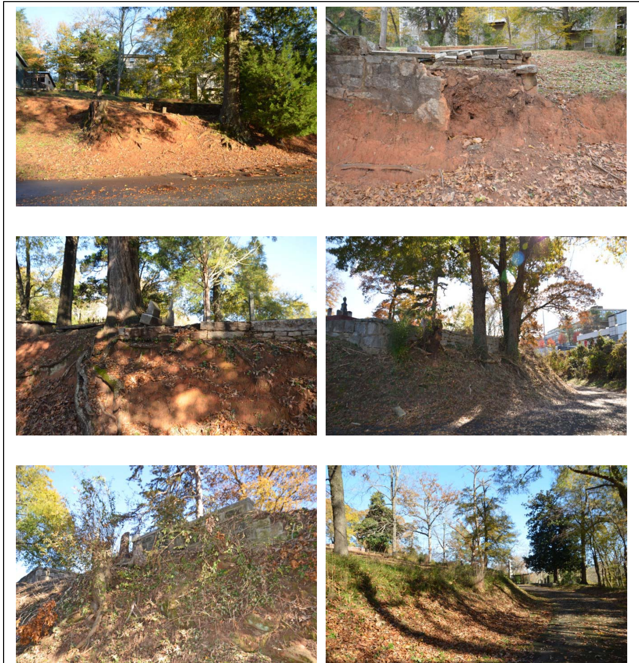
Figure 90. Erosion issues at Oconee Hill Cemetery. The upper left photo show erosion along the road at Factory Hill. The upper right photo shows the loss of a plot in the Factory Section. Additional erosion will begin to expose graves. The middle left photo shows tree roots and erosion along the Factory Section road. The middle right photo shows erosion along the west bank of West Hill. The lower left photo shows the recently cleared slope of West Hill. This will promote additional erosion. The lower right photo shows the south edge of West Hill where the bank is not as high, but erosion is still a concern.
