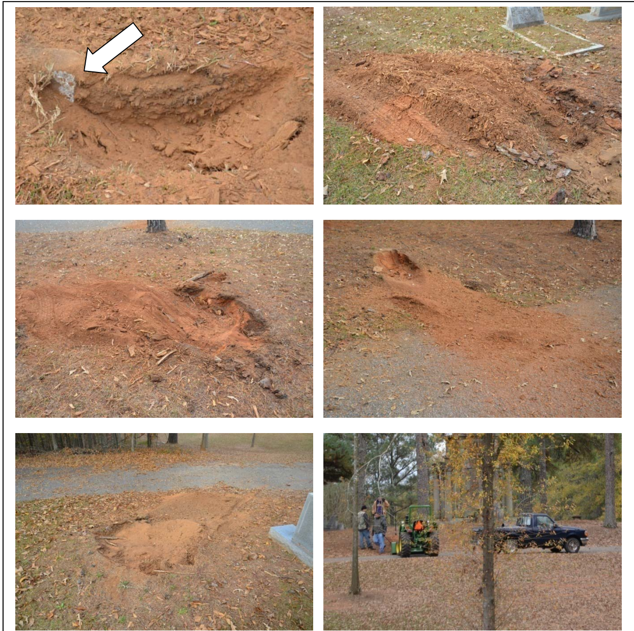
Figure 67. Stump grinding problems. Upper left, stump grinding hole, note the edge removed from the footstone by the grinder. Upper right, debris left by stump grinding. Middle left, stump grinding and debris. Middle right, stump grinding and debris left on the road by the contractor. Lower left, debris from stump grinding. Lower right, cemetery crew and cemetery equipment being used to clean up after the private stump grinding contractor. The contractor or the lot owners should have been required to correct the damage, not the cemetery.
