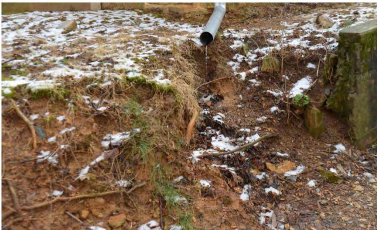
Figure 28. Erosion at the cemetery. The upper photo shows erosion along the west bank. The middle photo shows erosion from using the northwest corner as a bicycle ramp. The bottom photo shows erosion from a church building gutter draining directly onto the slope.
