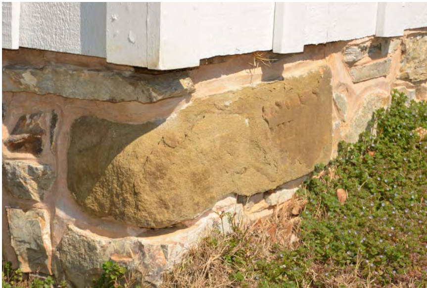
Figure 36. Cornerstone showing extensive spalling of the sandstone with the loss of most of the original carving.
