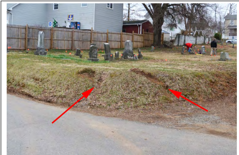
Figure 21. Rear of cemetery showing erosional areas caused by using the slope as a bike ramp. View is looking to the southeast.
