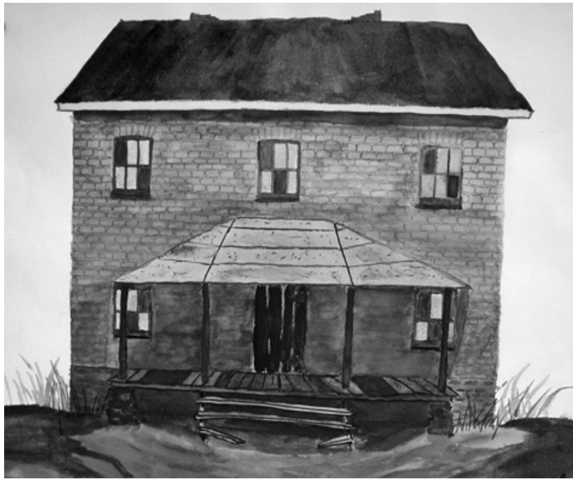
Figure 10. Allenbrook, ca. 1932 showing the porch across the front of the structure (adapted from Bass et al. 2004:Figure 6).
