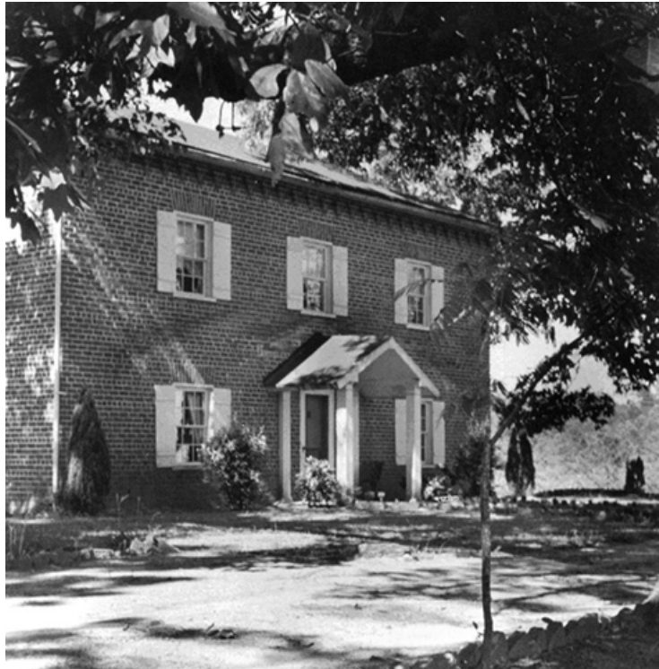
Figure 12. The replacement porch, ca. 1940 (adapted from Bass et al. 2004:Figure 10).
