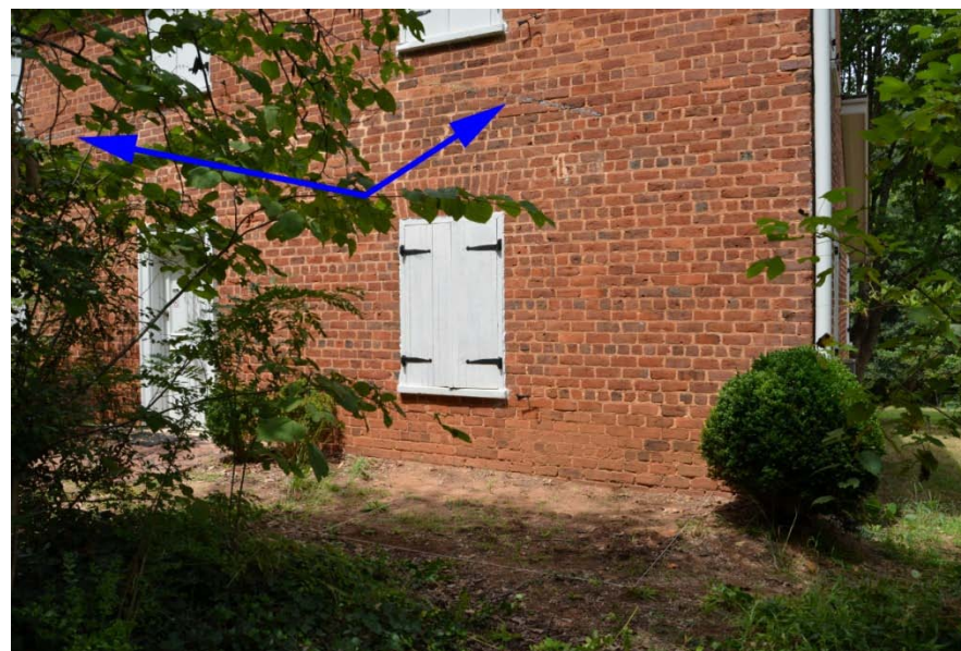
Figure 11. Shadow line (shown by blue arrows) of the original porch visible on the Allenbrook brick work.
