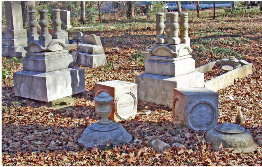
Figure 28. Collapsed monuments require resetting, often with associated repairs and pinning. In the background is a toppled monument that also requires pinning and resetting.
