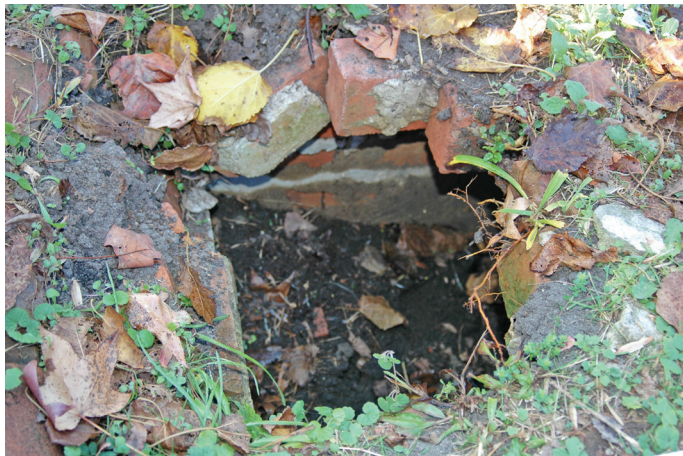
Figure 3. Area of vault prior to work. The top photograph shows the plywood covering placed by the City. The bottom photograph shows the collapsed portion of the vault looking east.
