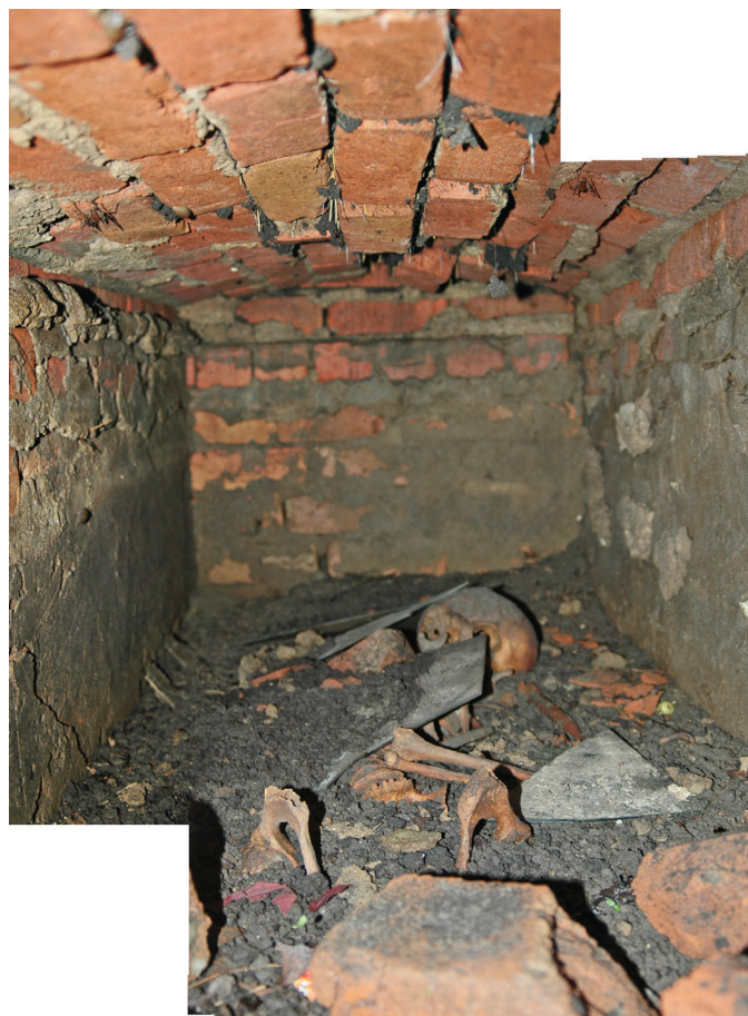
Figure 5. Interior of the vault, looking west.
