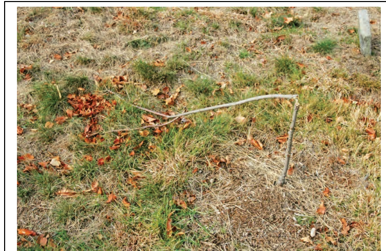
Figure 70. Example of damaged recent planting. This should be removed and replaced with a new specimen.
