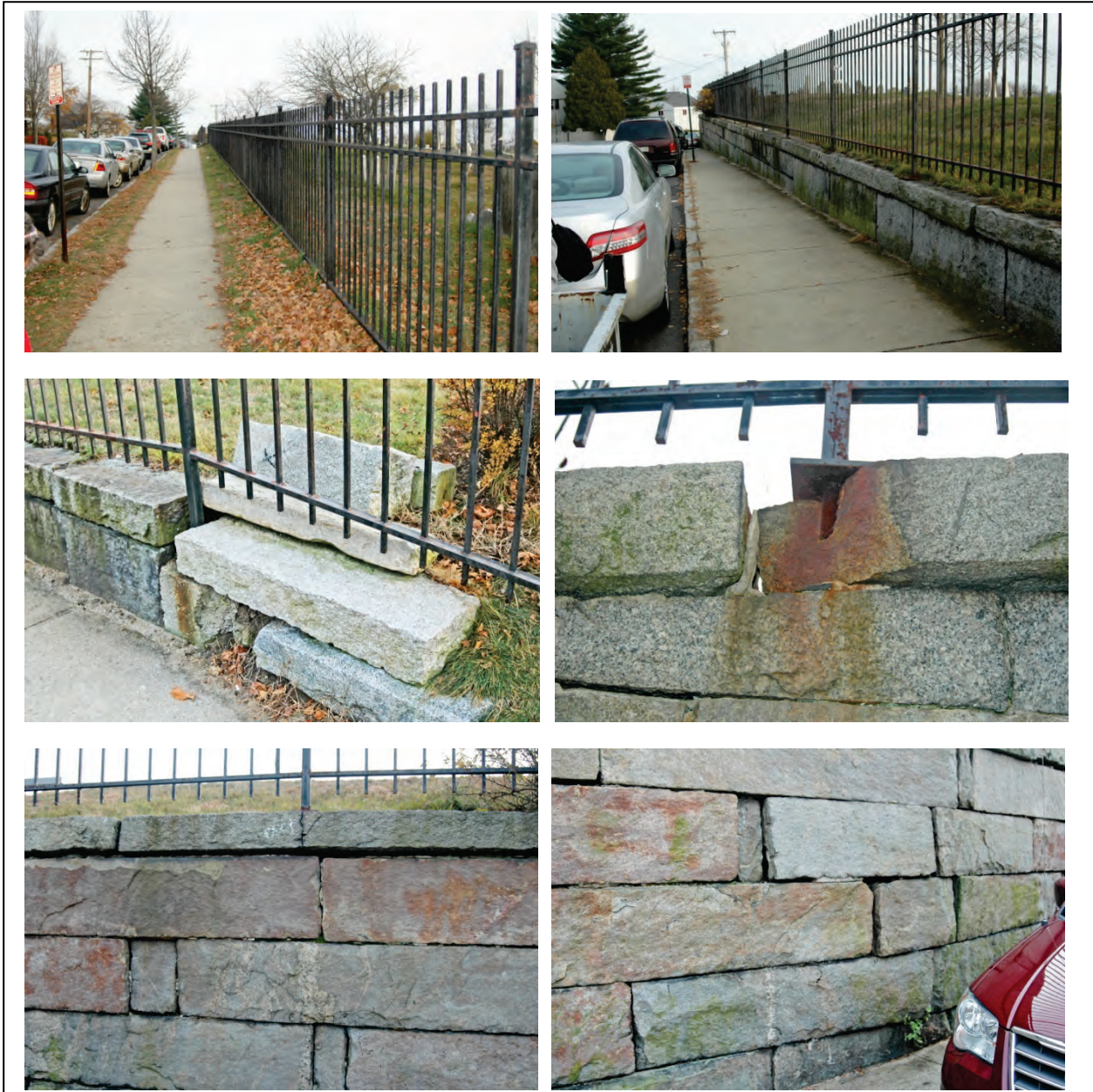
Figure 58. Mountfort Street fence and wall. Upper left photo shows the fence, looking to the northeast. Upper right shows the fence set on the granite retaining wall. Middle left shows where the granite wall has been “extended” by dumping granite coping. Middle right photo shows where iron jacking has split the granite coping. Lower left photo shows loss of mortar in the joints of the wall. Note also the crack that has formed from iron jacking at the line post in the center of the photo. Lower right shows a noticeable bulge in the wall on Mountfort. Joints are open and the retaining rock is set back in the wall, showing the movement outward.
