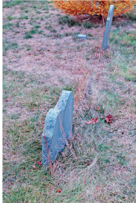
Figure 72. Height of the grass prior to the most recent mowing. In missed areas it is clear that the grass was allowed to grow to 10-14" before being mowed. This would completely hide some monuments and contribute to the damage observed in the cemetery.
