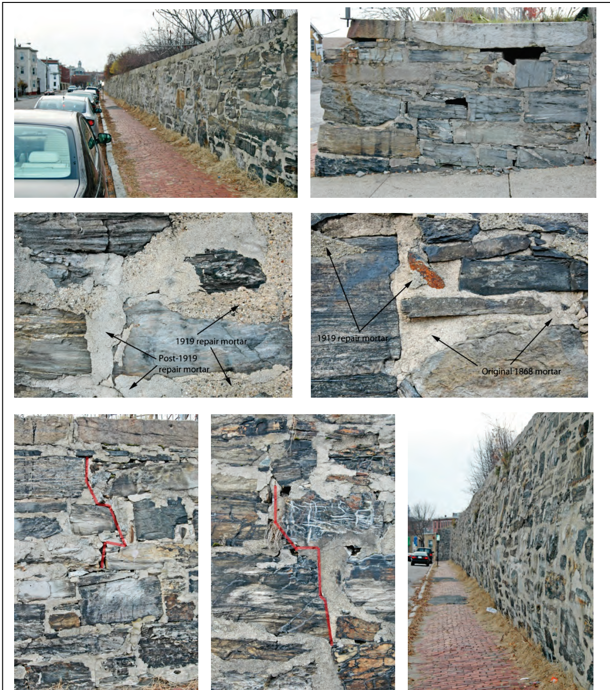
Figure 60. Federal Street wall. Upper left photo shows the wall along Federal Street, looking southeast. Upper right shows the wall along Mountfort. Note the missing stones. Middle row photos show the different mortars identified visually in the wall. Lower left and middle photos show cracks following the mortar joints. Lower right photo shows a pronounced bulge in the wall, affecting an area measuring about 30 feet along the street and the full height of the wall.
