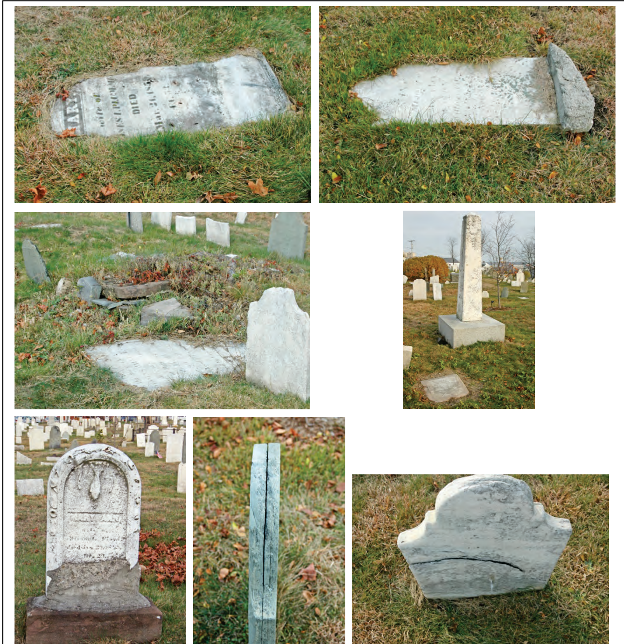
Figure 82. Conservation issues. The top row illustrates two fallen stones that should be reset to prevent additional damage. The photo on the right shows a stone that had previously been reset using a hard Portland cement. Not only did this not keep the stone upright, but it could cause additional damage. A conservator should carefully remove the concrete, allowing the stone to be reset in a pea gravel bed. The middle row, left photo shows a collapsed box tomb. The ledger is intact, but laying on the ground is subject to additional damage. The image on the right shows an obelisk reset without an intervening base (shown in the left foreground). The bottom row left illustrates the inappropriate use of Portland cement to “repair” a stone. Bottom row middle and right photos show spalling slate and marble.
