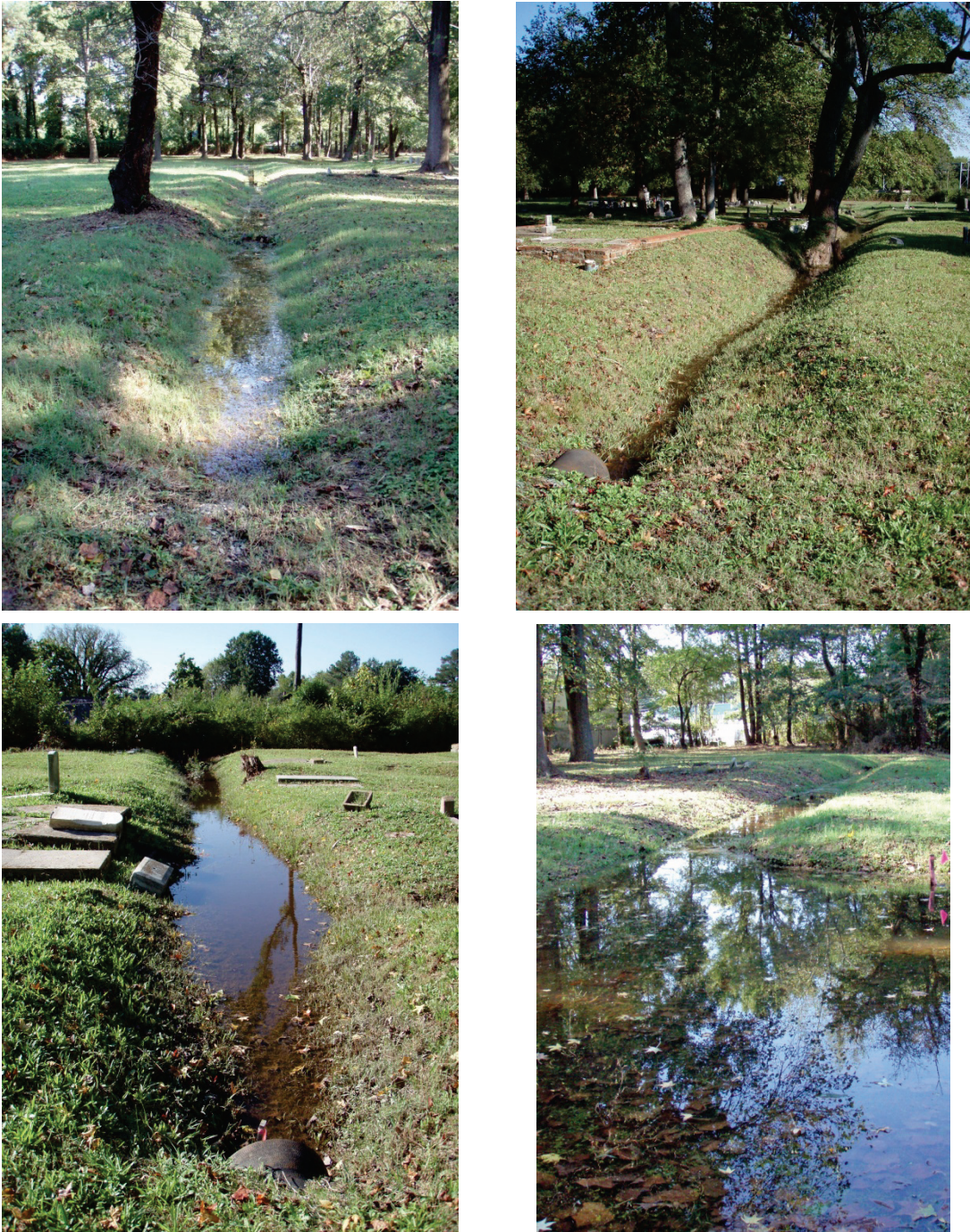
Figure 23. Water drainage in the cemetery after several days without rain. Upper left, north-south ditch near the west end of Mount Olive looking north. Upper right, north-south ditch between Mount Calvary and Mount Olive looking north. Lower left, north-south drain between Mount Calvary and Mount Olive looking south. Lower right, ditch and ponded area at the northwest corner of Mount Olive, looking southwest.
