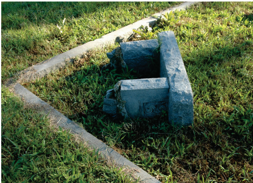
Figure 31. This monumental bench lacked an appropriate foundation, evidencing improper construction.
