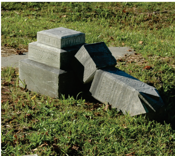
Figure 28. This stone was likely vandalized (the base is relatively level and there are no trees or stumps nearby).
