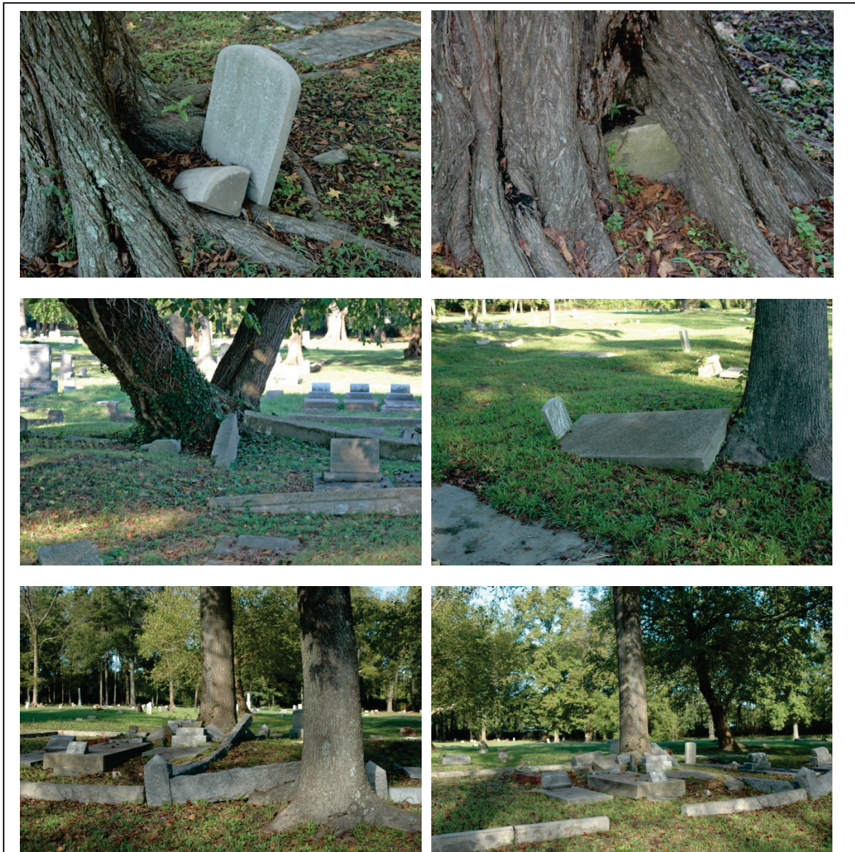
Figure 35. Examples of plots or stones damaged by tree growth. The top left photo shows a large tree with roots beginning to encompass a tablet. Here it may be possible to remove the stone without damage to the tree. The top right photo shows a stone completely grown into a tree. The stone cannot be recovered without killing the tree – which we do not recommend. Middle row left photo shows coping displaced by a large tree. We recommend relocating the coping to avoid the tree. Middle row right photo shows a large tree growing into a vault. It may be possible to relocate the vault cover and tablet. Lower row left and right photos show extensive damage to coping and stones by a large tree. Here it may be possible to relocate coping and stones to avoid the tree. In most cases the tree, if mature and healthy, should be retained.
