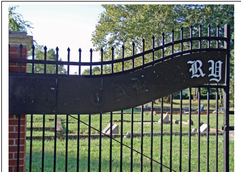
Figure 30. Entrance gate to Mount Calvary showing the loss of letters that require replacement.
