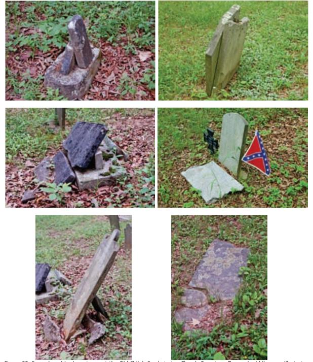
Figure 25. Examples of broken stones at the Old Shiloh Presbyterian Church Cemetery. Top and middle rows illustrate a variety of stone breaks. Bottom left illustrates a broken stone propped up. Should the stone fall it will certainly break again, increasing repair costs. The stone at the bottom right lying on the ground is subject to mower and pedestrian damage.
