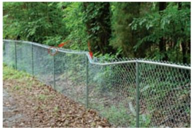
Figure 15. Damaged fence section showing dislodged top cap and severely bent top rail. This requires immediate replacement.
