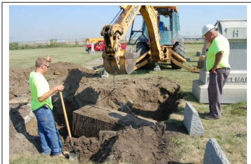
Figure 14. Vault removal by Geils Funeral Home and Stark & Son Excavating.
