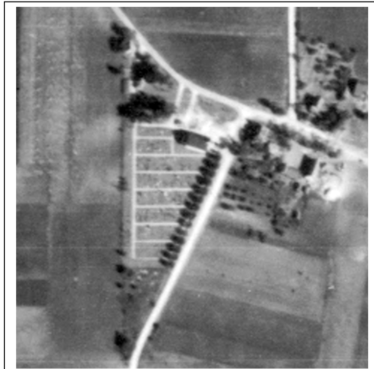
Figure 11. 1939 aerial photograph of St. Johannes Cemetery. Pathways are clearly visible, as is the church in the northeast corner of the cemetery. Note also the farms to the northeast and east of the cemetery.
