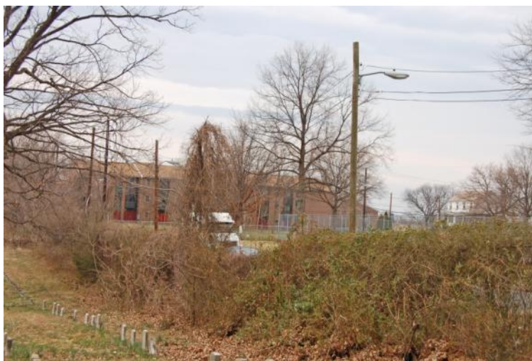
Figure 30. Example of cobra lamps along Robinson Place at the north edge of the cemetery. Note also the dilapidated and overgrown condition of the fence.
