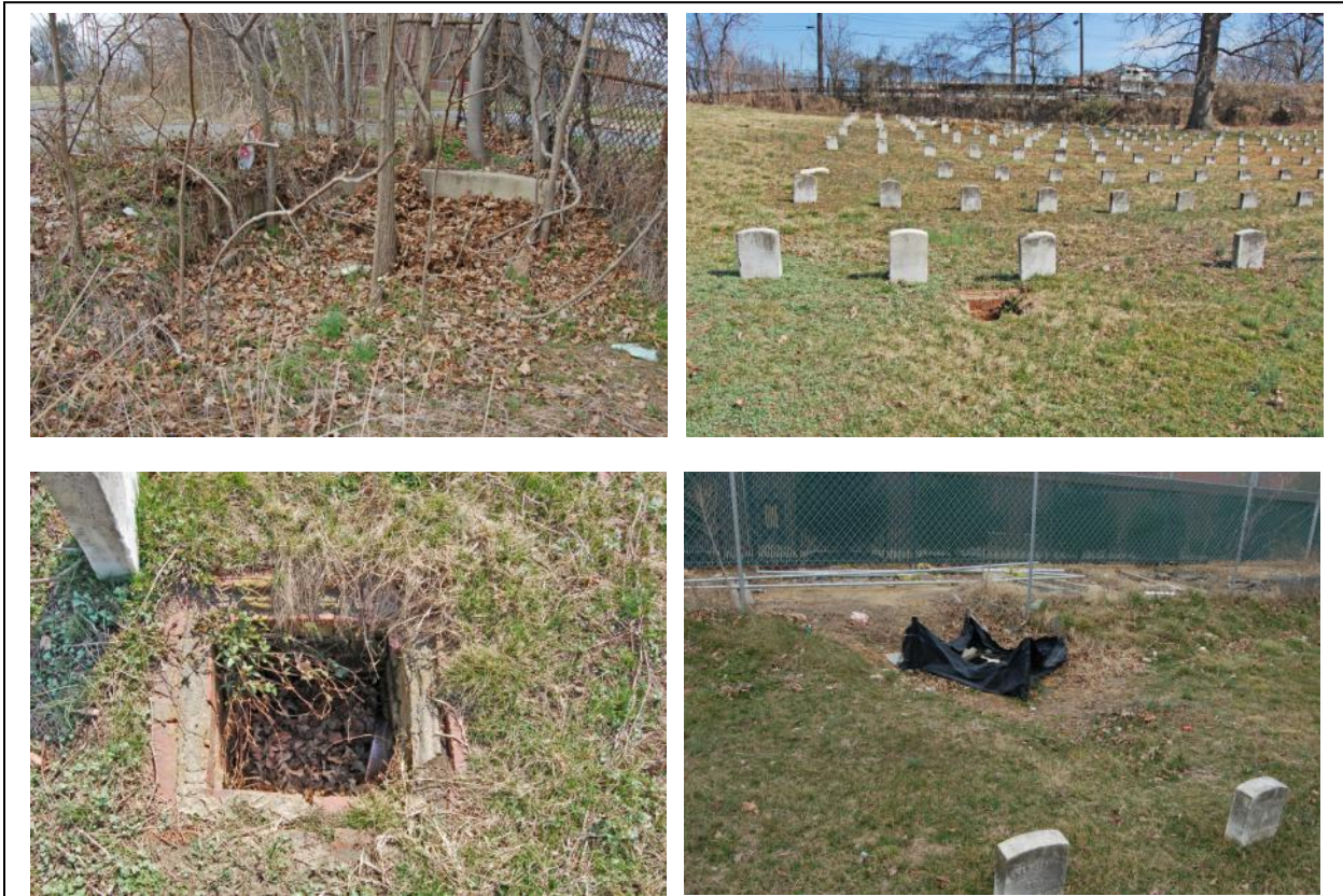
Figure 29. Drains in the East Campus Cemetery. Upper left shows what appears to be a box culvert running under Robinson Place that requires cleaning and evaluation. Upper right shows one of two brick box drains at the southern edge of Section 3. These require cleaning and video inspection. Lower left shows a close-up of the western brick box drain. Note the glazed drain pipe running southward to a modern drain close to the southern entrance gate. Lower right photo shows a modern drain at the south edge of Section 13.
