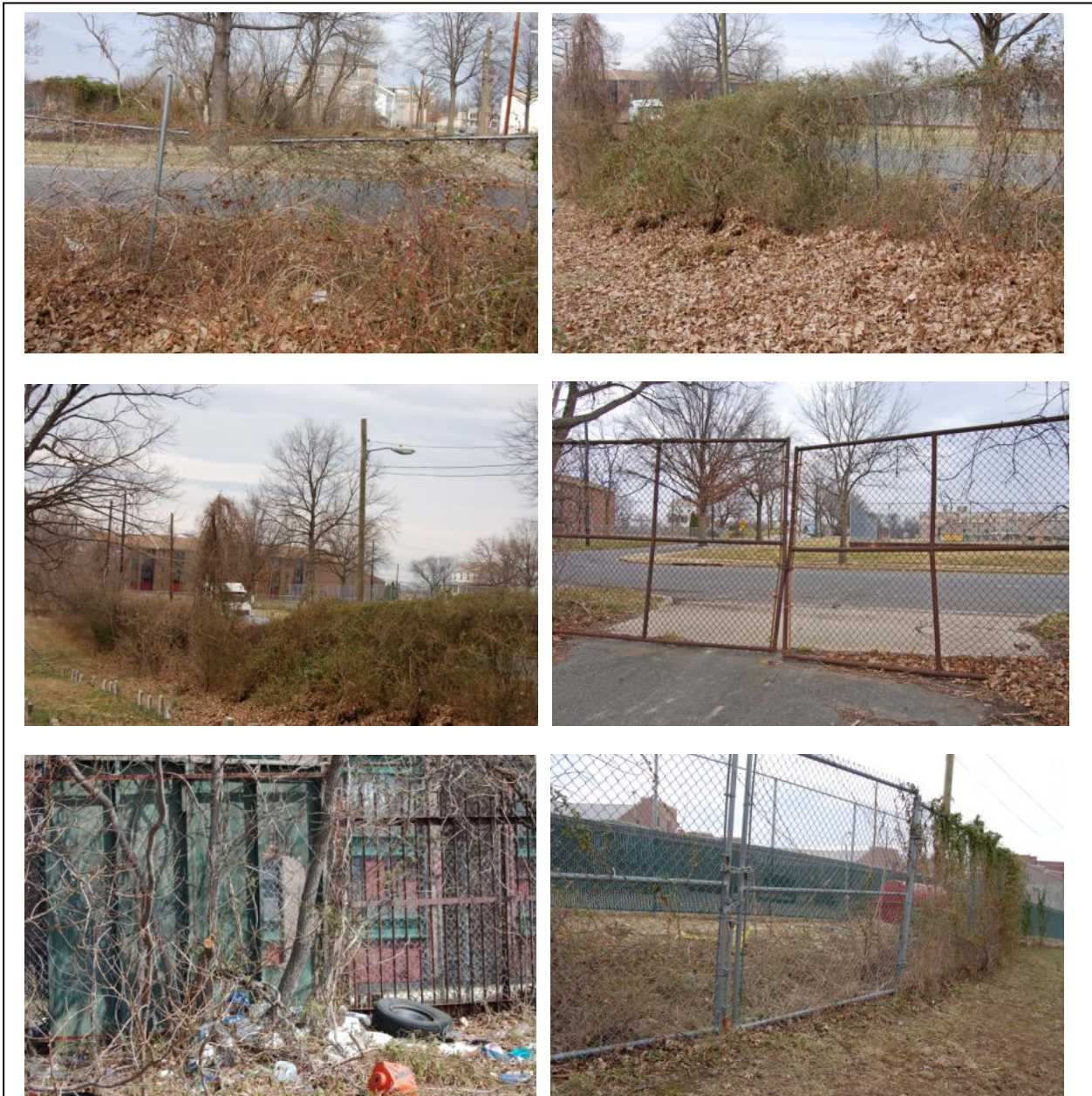
Figure 32. Problems with the existing cemetery fence. Upper left shows damaged fence along Robinson Place that can be easily scaled. Upper right shows the fence with dense vegetation. Middle left shows the same fence with so much vegetation that its condition can't be adequately assessed. All of this vegetation should be removed. Middle right shows the existing gates on Robinson Place that should be removed. Lower left shows an iron fence that offers almost no security. A section is missing and replaced with a wood insert, part of which has been chopped away, allowing easy access into the cemetery. Lower right shows the existing southern gate. A maintenance gate is needed, but probably does not need to be this wide.
