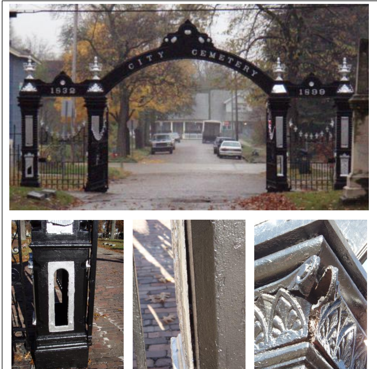
Figure 21. Gate problems. The top photo shows the entrance gate from within the cemetery looking toward Colfax Avenue. Below from left to right, an example of missing fabric (above is part of a cover plate that has been broken), a joint in the post that requires careful caulking prior to painting, and damaged decorative design and old weld that has broken apart (repair will require disassembly of the column, although water can be repelled by careful caulking until the repair can be afforded).
