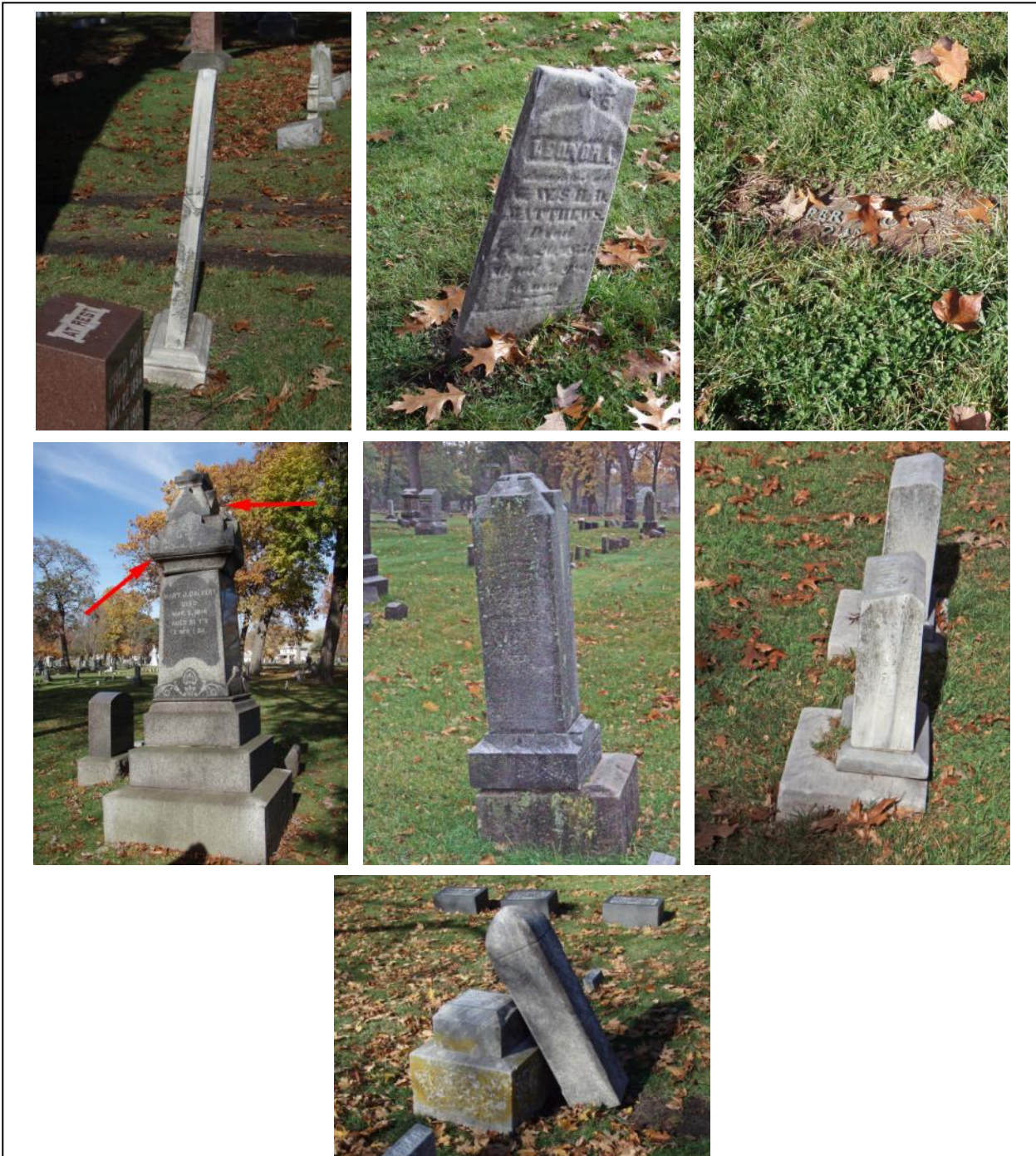
Figure 36. Examples of stones that require resetting. The top row illustrates simple resets that could be done by staff or volunteers with little training. Middle row left and middle illustrate two stones that could be a hazard to the public and require immediate conservation intervention. Middle row right shows a small stone that can be reset by volunteers. Bottom row illustrates the eventual result without treatment
