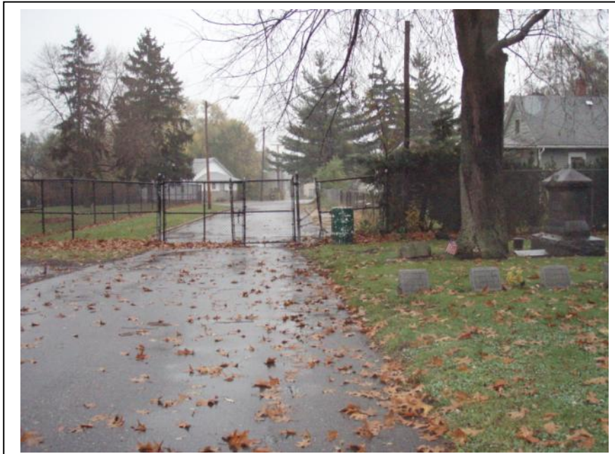
Figure 16. Improperly set gate on the east side of the cemetery at Linden Avenue. This requires immediate attention to eliminate the pedestrian passageway.
