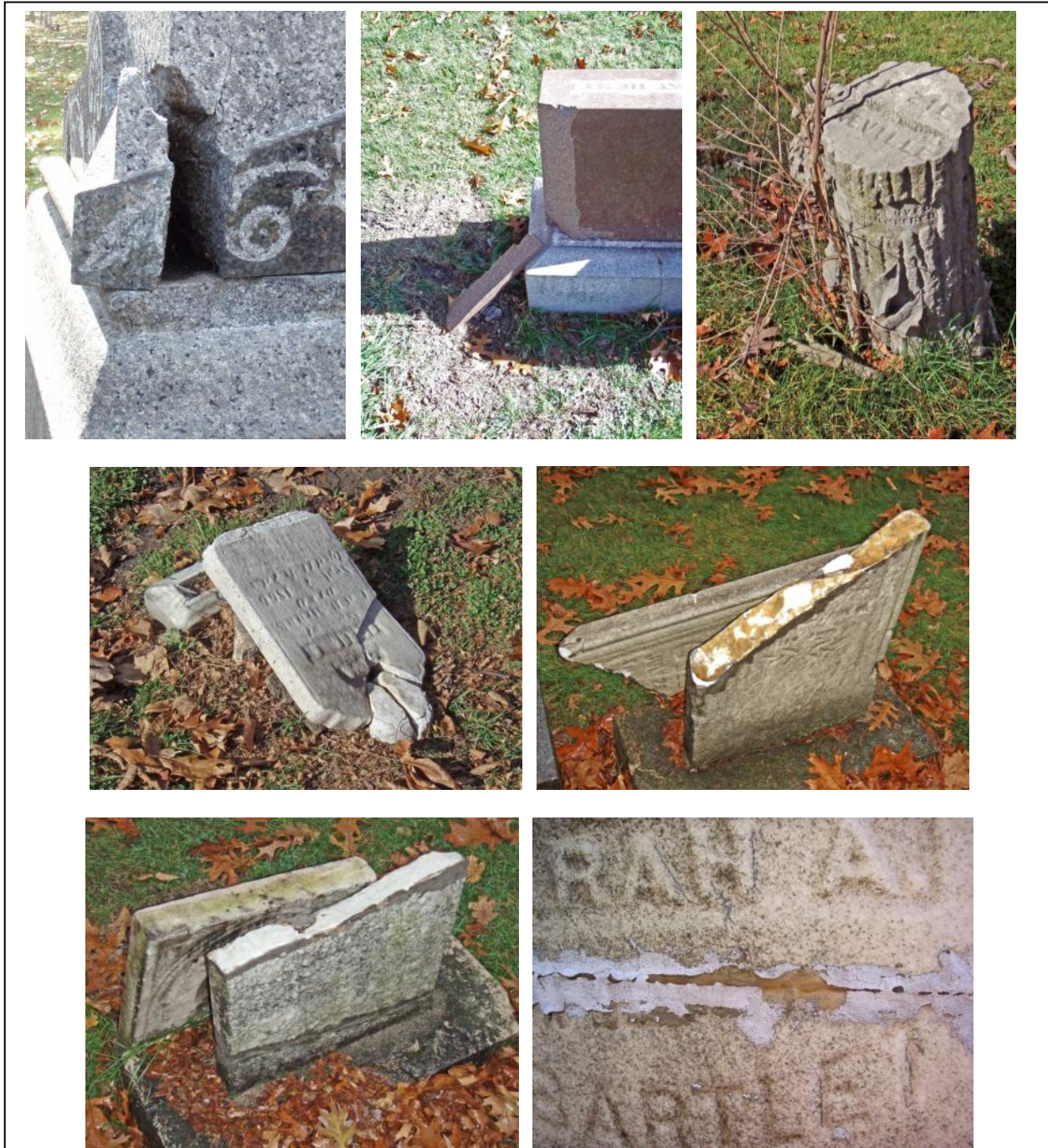
Figure 34. Examples of broken and improperly repaired stones. Top left and middle photos show tree damaged granite markers. Top right shows a sandstone marker with a fragment broken off and lying on the ground. Middle left shows a marble tab in socket stone that has fallen and shattered. Middle right shows one of the many failed "simple epoxy" repairs in the cemetery; note the yellowing epoxy smeared on the stone face. Bottom left shows another failed repair. Bottom right shows where smeared epoxy is being covered by white paint.
