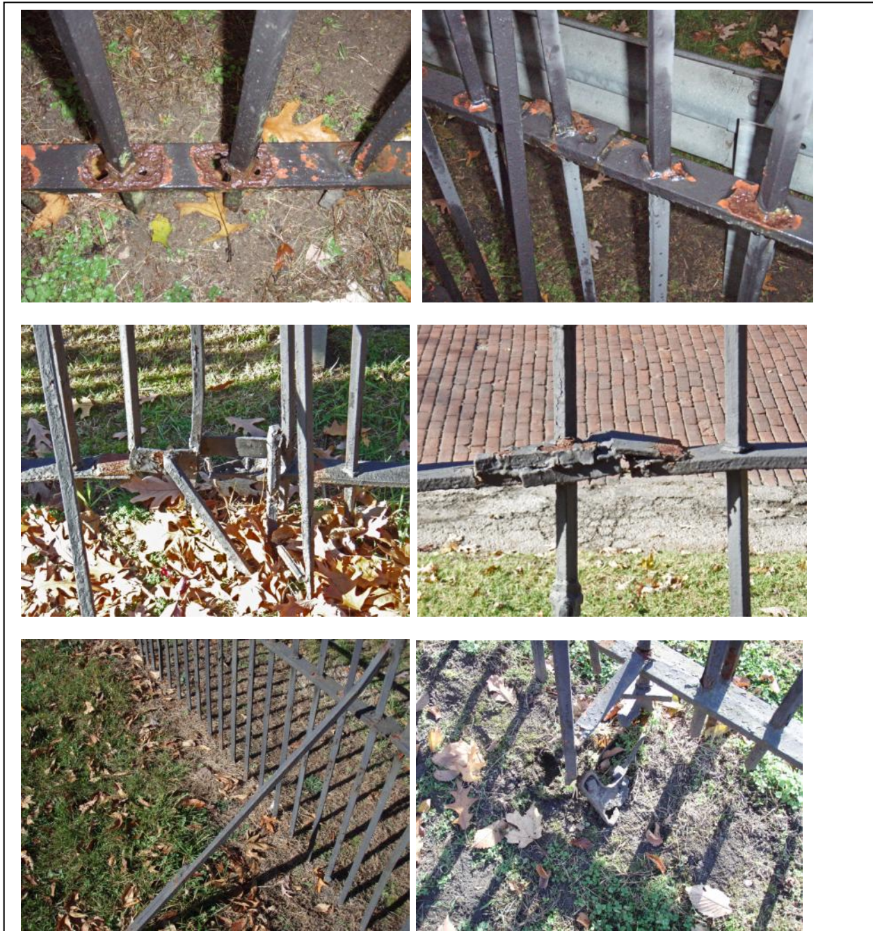
Figure 20. Problems with the City Cemetery boundary fence. Upper left shows an example of extensive corrosion and failing paint. Upper right is an example of failing paint. The middle row shows two examples of the very poor workmanship used in fence repairs. This quality of work must not be allowed on historic fabric and all such repairs must be removed. Lower left shows the bottom rail buried in soil. The lower right shows a loose part lying on the ground and a line support completely corroded through.
