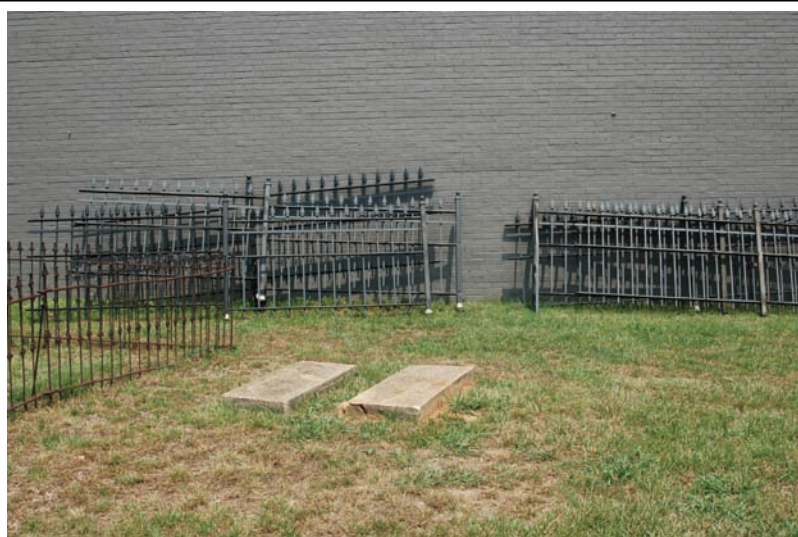
Figure 23. Loose sections of the boundary fence should be secured together to minimize the potential for their theft.
