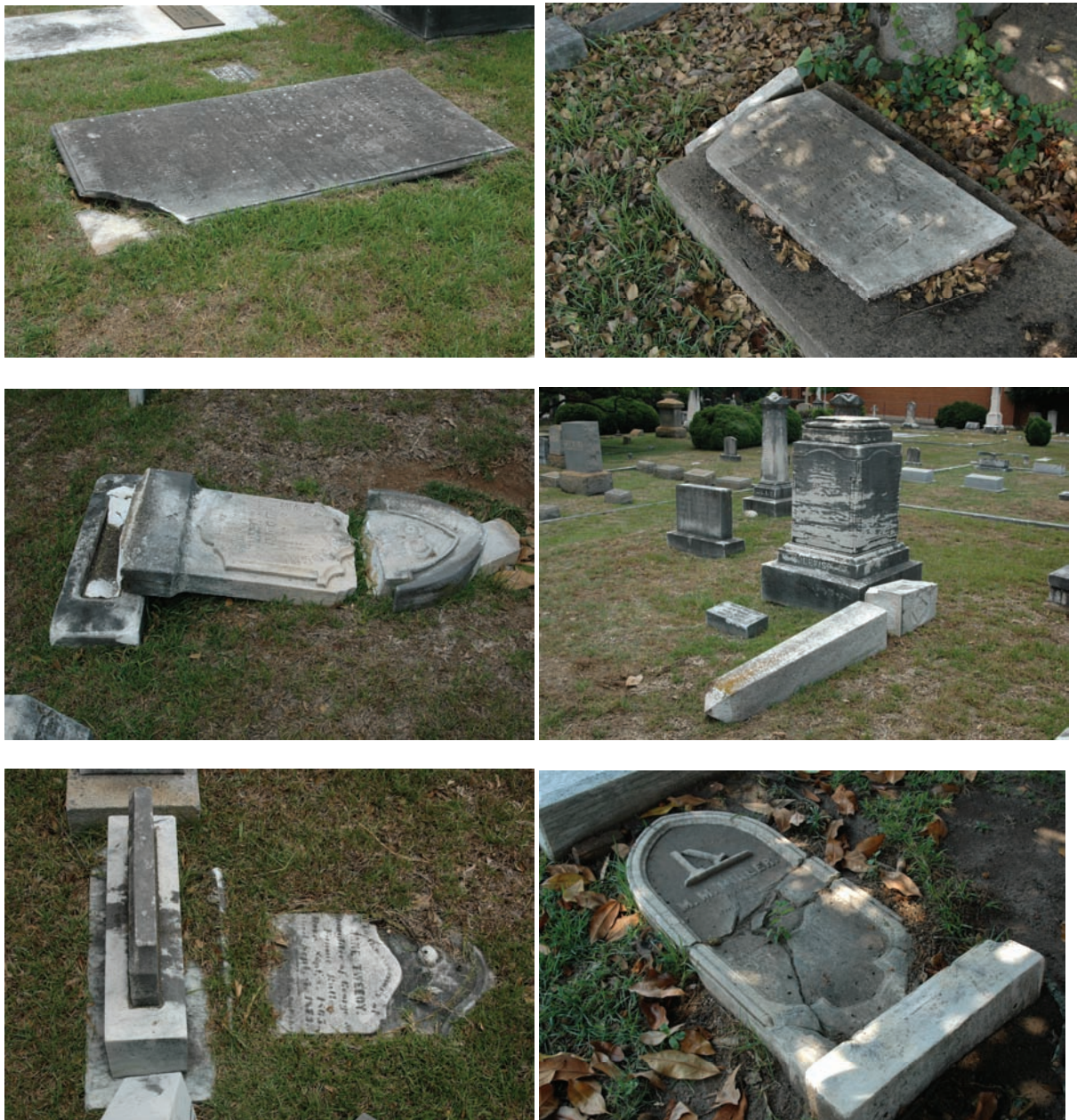
Figure 54. Examples of broken stones requiring professional conservation. Upper left shows a broken ledger that exposed a vault below; this is a serious trip hazard. Upper right shows a broken headstone. Middle left shows a broken tab in socket; the upper portion shows a failed epoxy repair, illustrating the problem with using epoxy. Middle right shows a broken obelisk that will require pinning, as well as pinning to its base to ensure safety to the public. Lower left shows a stone broken so long ago that grass is beginning to grow over it. Lower right shows another very old damaged stone. All of these stone require drilling and pinning, with the breaks then infilled with a repair mortar.
