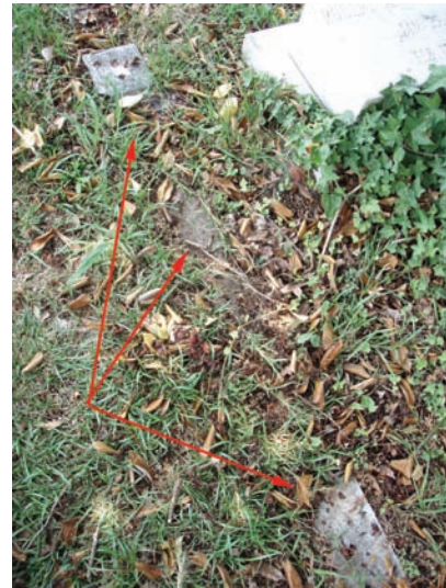
Figure 52. Marker and coping disappearing below the ground surface.
