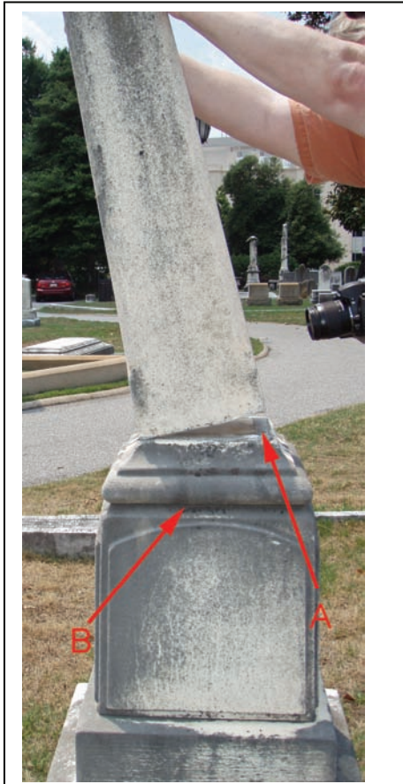
Figure 53. Example of improper repair. Monument setting compound was used to reset the obelisk at A, but this has failed with very little force. In addition, the base is also unattached at B. This monument represents a serious threat to the public.
