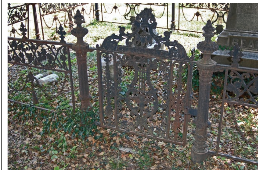
Figure 23. Gates such as these are unsecured and provide an easy target for thieves.
