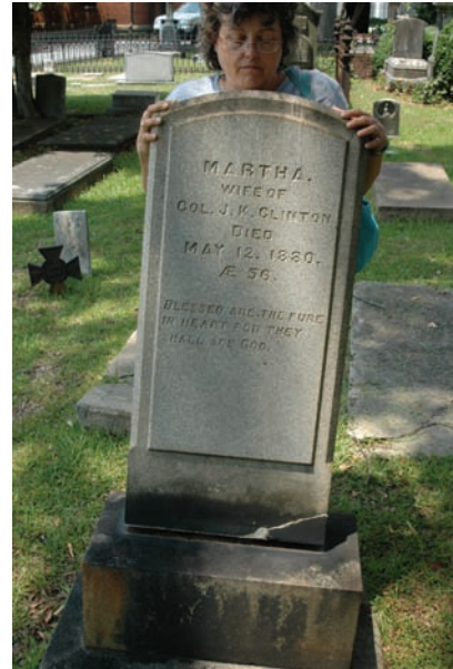
Figure 56. Inappropriate use of setting compound to “reattach” the corner of this monument did nothing to deal with the more serious problem of the monuments instability – resulting in a significant liability to the church.
