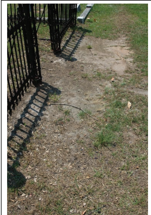
Figure 46. Examples of heavily compacted area requiring renovation.
