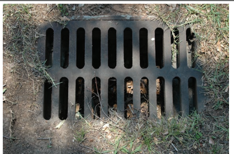
Figure 19. One of the cemetery drains, showing an accumulation of leaves and other debris. These should be cleaned on a yearly basis.
