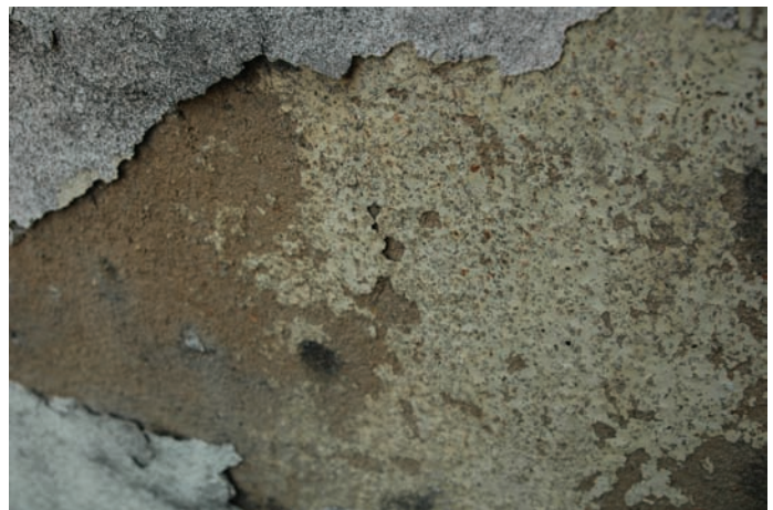
Figure 27. Failing non-breathable coating that has been applied to the mausoleum. Bottom photo shows the original colored whitewash over the lime-based stucco.
