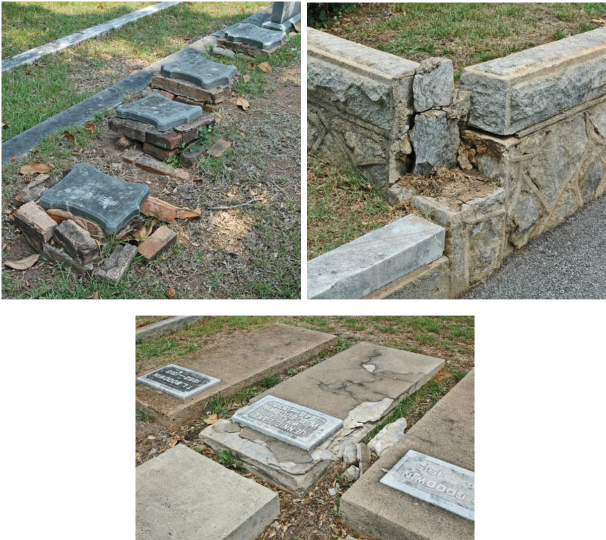
Figure 58. Examples of masonry and concrete deterioration.
