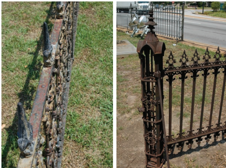
Figure 24. Two examples of ironwork that require cleaning and painting. The example on the left illustrates a failed coating, while the fence on the right exhibits only bare metal.
