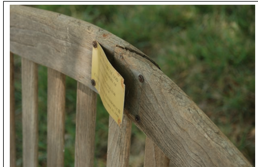
Figure 30. Cemetery bench placed in 1998 that requires replacement or maintenance.
