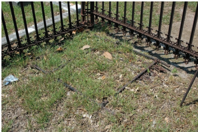
Figure 25. Examples of loose fence parts that should be collected and safely stored.
