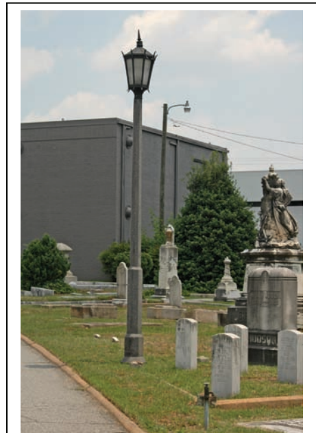
Figure 20. Example of the two types of lighting fixtures in the cemetery. In the foreground is a pole lamp with underground service. In the background is a “cobra head” lamp with overhead wiring.
