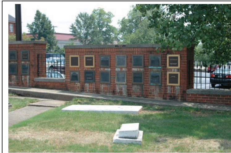
Figure 28. Columbarium showing evidence of bronze disease and salt staining.
