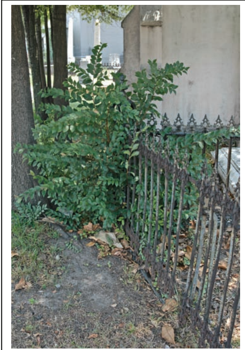
Figure 38. Example of volunteer growth that should be removed before it harms the ironwork.
