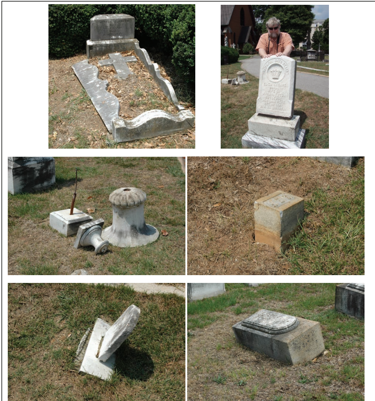
Figure 55. Other stone problems. Upper right photo shows a displaced cradle side board. The cross on the interior does not belong with this monument and should be collected and stored safely until its monument is found. Upper right monument requires pinning. Middle left monument shows an impalement hazard to the public. Middle right is an example of a monument that could easily be reset by the cemetery staff. Lower row shows examples of tilted monuments that can be reset by the cemetery staff.
