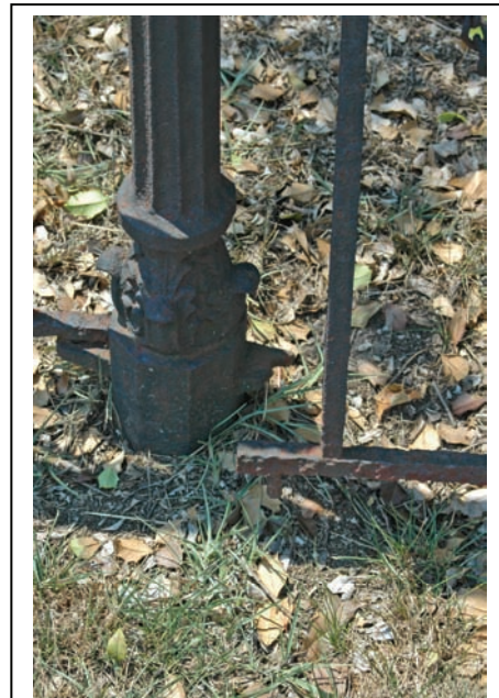
Figure 26. Example of a broken connector where welding is an inappropriate repair technique.
