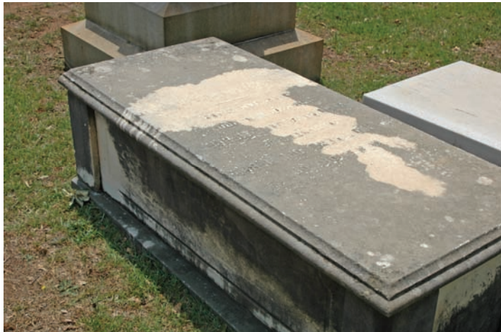
Figure 57. Bleach spilled on this stone has caused a significant disfigurement.
