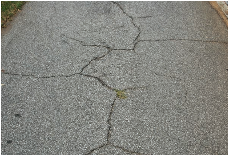
Figure 15.Examples of the road deterioration in the cemetery.
