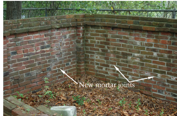
Figure 20. Two areas of wall repair. Note the light colored (new) mortar and the loss of the original bonding pattern. Note also on the left photo areas of brickwork requiring repointing, as well as sections of old wall lying on the ground.
