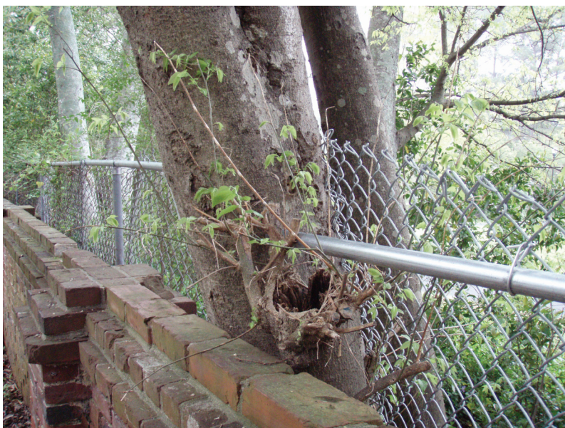
Figure 13. Dilapidated chain link fence between the cemetery and park, showing loss of the barbwire and damage from the tree.
