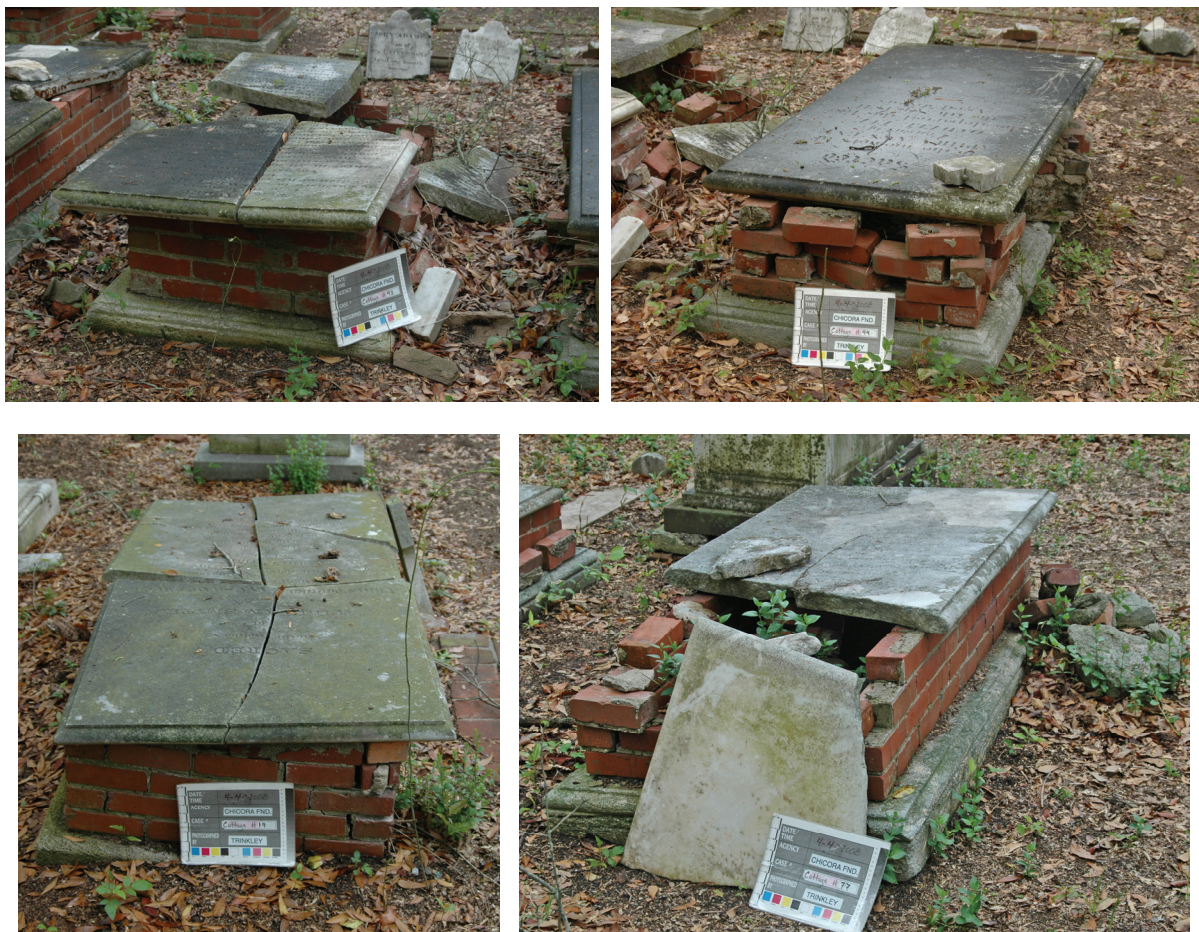
Figure 25. Examples of collapsing brick box tombs that require repair.
