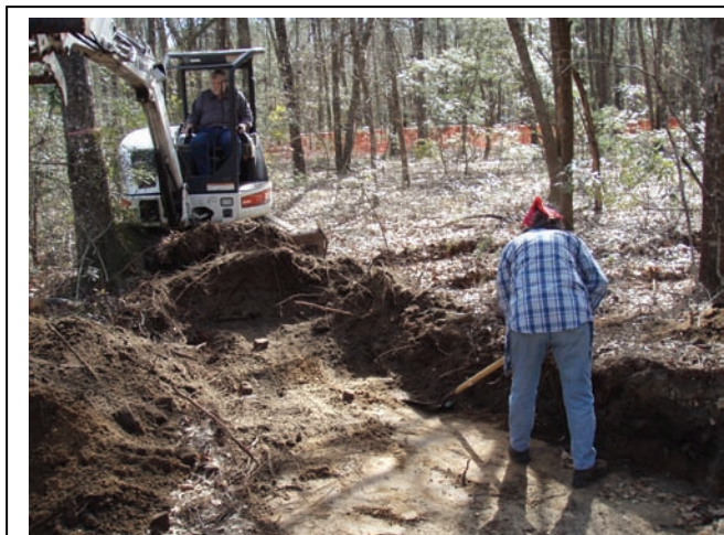
Figure 7. Stripping using a Bobcat and a toothless bucket followed by flat shoveling.
