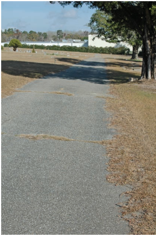
Figure 54. The paved roads in the new section of Magnolia Cemetery are cracked and require filling or sealing. The roads should also be regularly edged.
