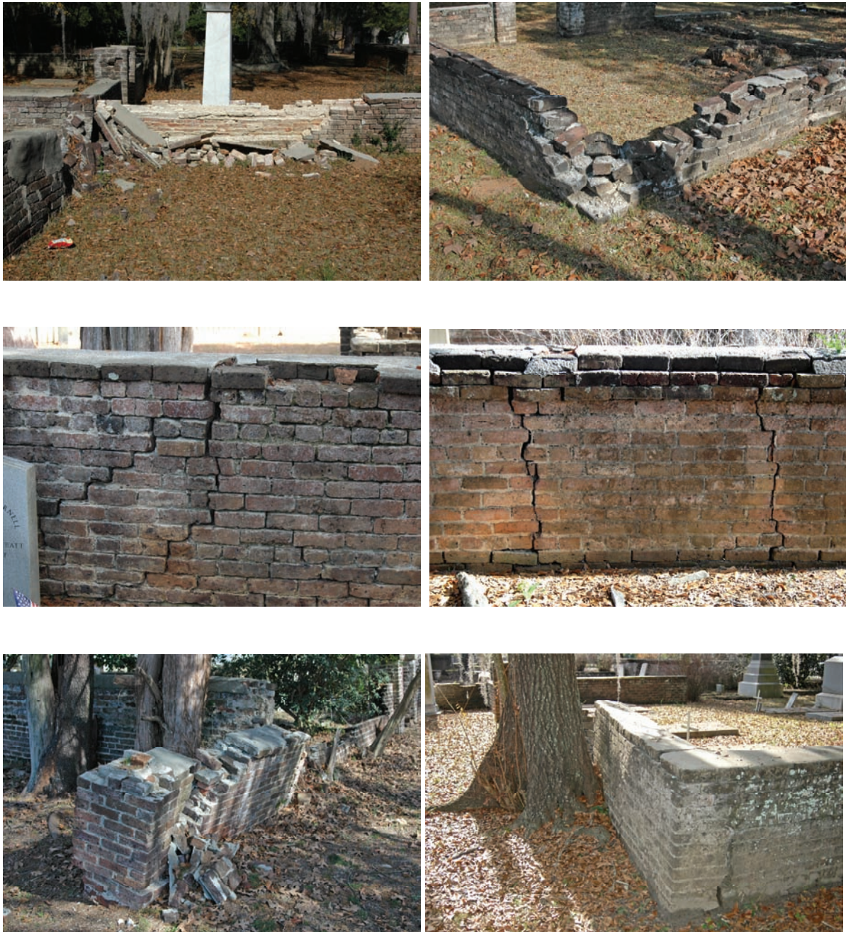
Figure 32. Brick wall problems at Old Cemetery. The top two photographs show walls that have collapsed. Substantial portions of these walls will need to be rebuilt. The middle two photographs reveal extensive cracking and settling. Some cracks may be repaired, others will necessitate rebuilding a section of the wall after foundation repair. The bottom two photographs show walls damaged by trees. In these cases the health of the trees will determine if the tree can be removed and the wall rebuilt.
