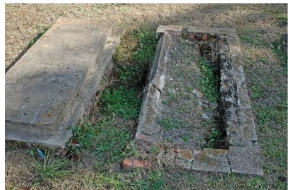
Figure 78. Examples of collapsing ledgers.
