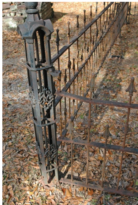
Figure 16. Damaged connectors on a plot fence. Note also the lack of a protective coating.
