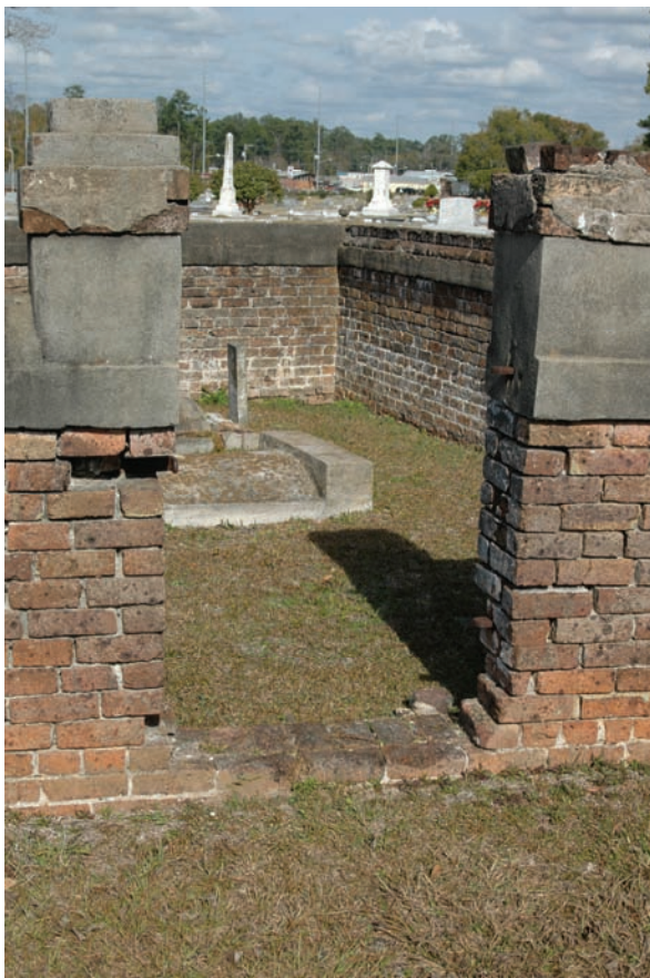
Figure 112. Brick plot that requires repointing.
