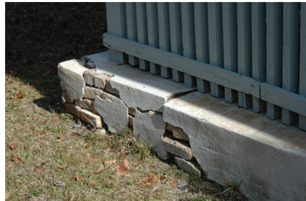
Figure 29. Old Cemetery gazebo showing roof deterioration, rotted trim, and foundation collapse.
