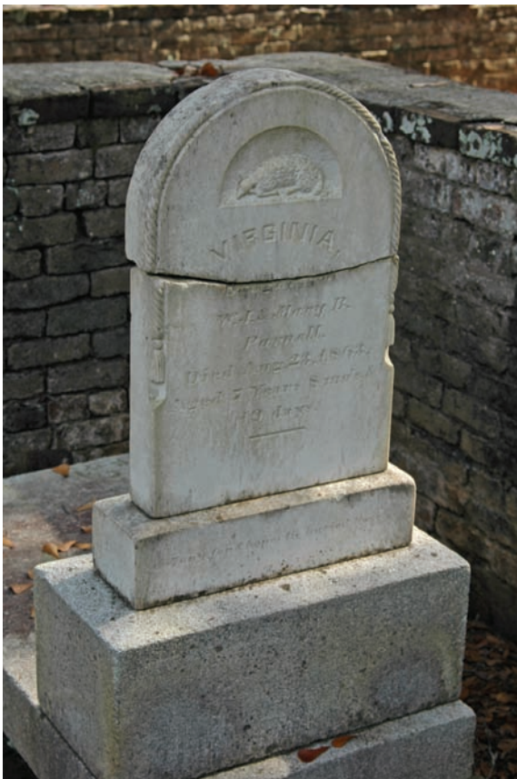
Figure 30. Broken, unstable stone that is a hazard to the public. Repair should be a high priority.
