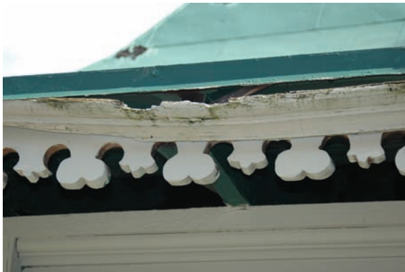
Figure 29. Old Cemetery gazebo showing roof deterioration, rotted trim, and foundation collapse.
