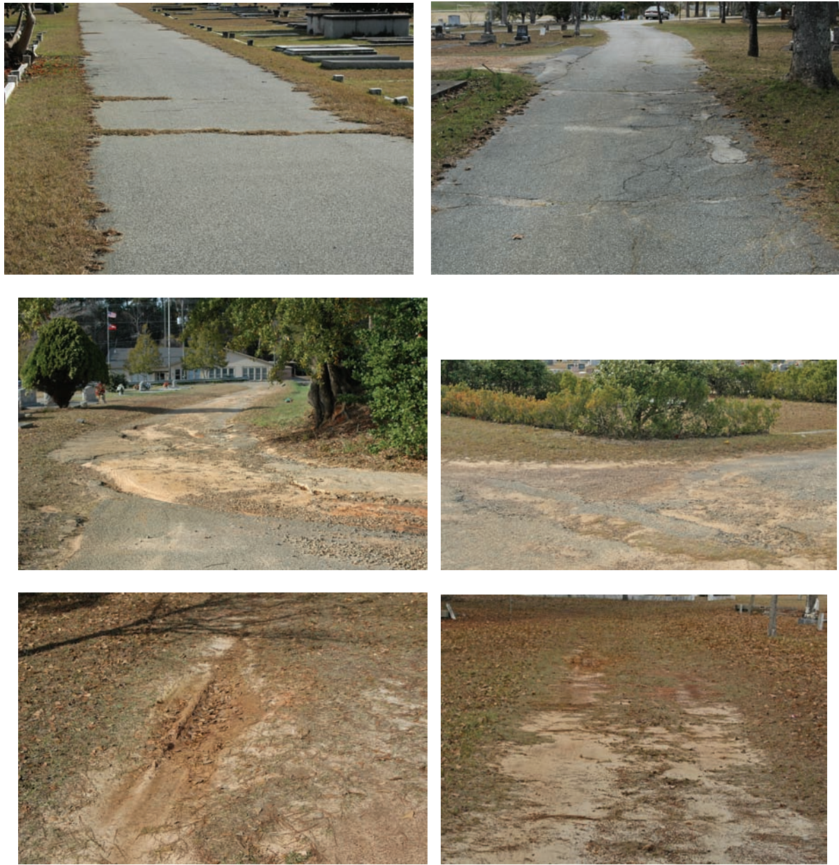
Figure 83. Road problems in Laurel Hill Cemetery. From upper left to lower right: paved road in the new section showing cracking, note that grass is not being edged; paved road in the old section showing cracking and previous patch repairs, again note the absence of edging; deteriorated roadway showing erosion and inappropriate (and ineffective) concrete patch; deteriorated roadway in the new section; rutted dirt roadway in the old section, indicating that these roads get muddy during rainy weather; heavily compacted dirt roadway in the old section that disappears with no clear or certain pathway.
