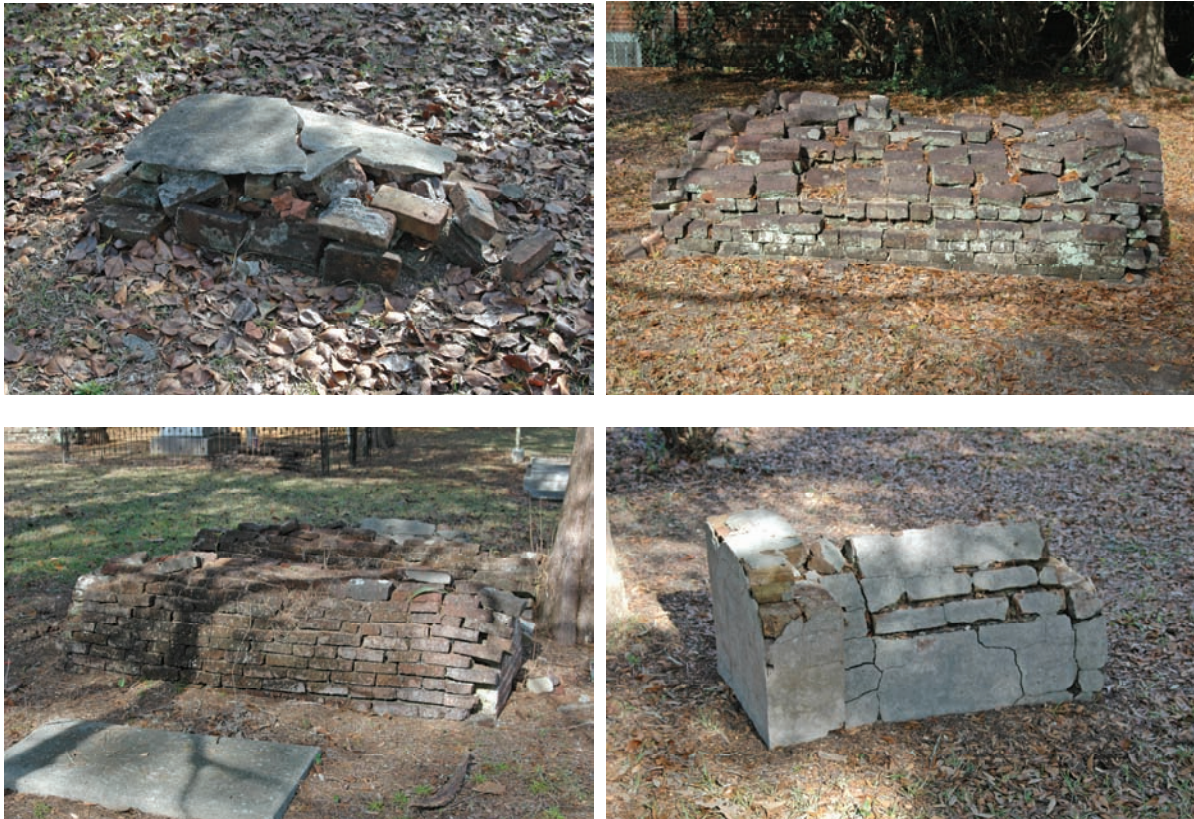
Figure 33. Brick tomb problems at Old Cemetery. These “oven” tombs are in poor condition and will require extensive reconstruction. The use of hard Portland cement stucco is especially problematical and much will need to be stripped off.
