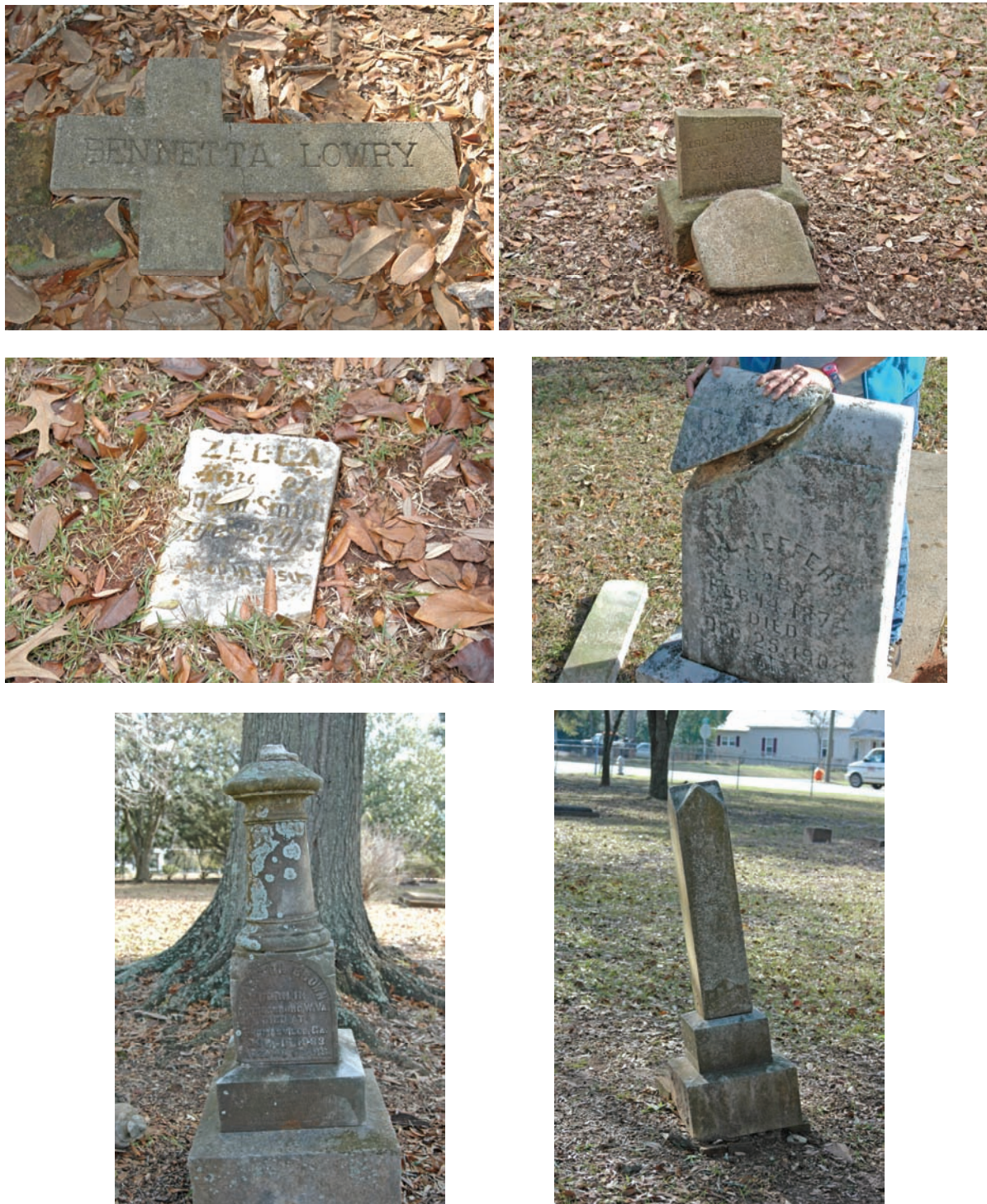
Figure 49. Conservation issues at Flipper Cemetery. Top photos illustrate broken concrete monuments. Middle photos illustrate broken marble stones. Bottom photos illustrate severely leaning monuments that require resetting.
