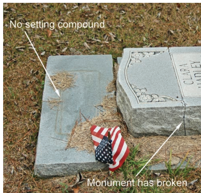
Figure 6. This granite die on base monument was set without using setting compound. This allowed the die to be easily displaced – and as it fell it broke. Its repair will be a significant expense ($600) that could have been prevented using $5 worth of setting compound.
