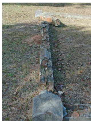
Figure 50. Top photo illustrates brick wall with missing sections and brick requiring repointing. The bottom photo illustrates brick coping deteriorated through Portland cement stucco and mechanical damage.
