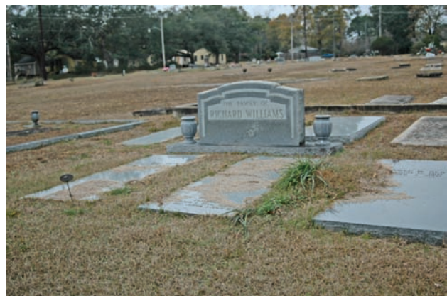
Figure 68. Examples of grass left on monuments in both the old and new sections of Magnolia. Some grass has been on monuments for so long it has begun to mulch down, staining the marble.
