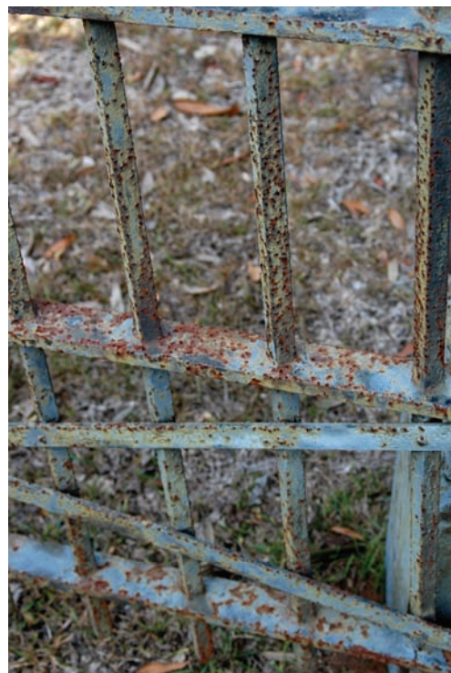
Figure 18. Example of heavy corrosion on the cemetery's boundary
