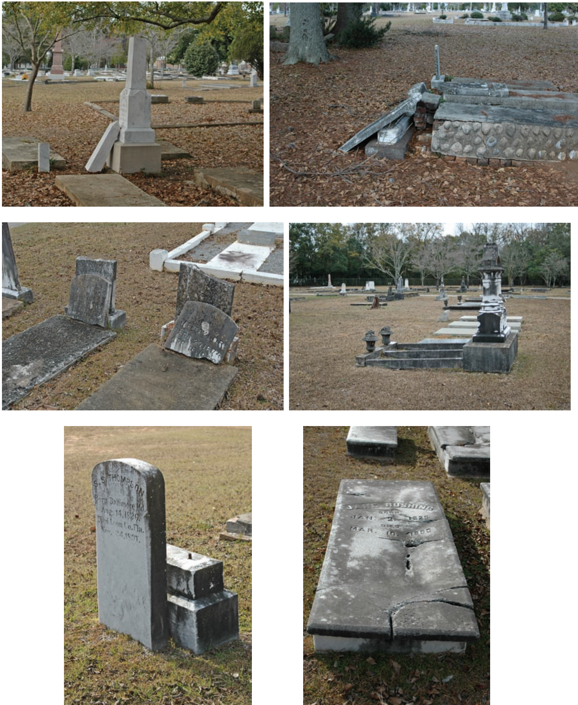
Figure 108. Typical stone conservation issues at Laurel Hill. From upper left to lower right: broken obelisk; tab in socket with broken tab; broken headstones; elevated monument with cradle side boards elevated; die on base with ferrous pins; extensively sugaring and warping ledger.
