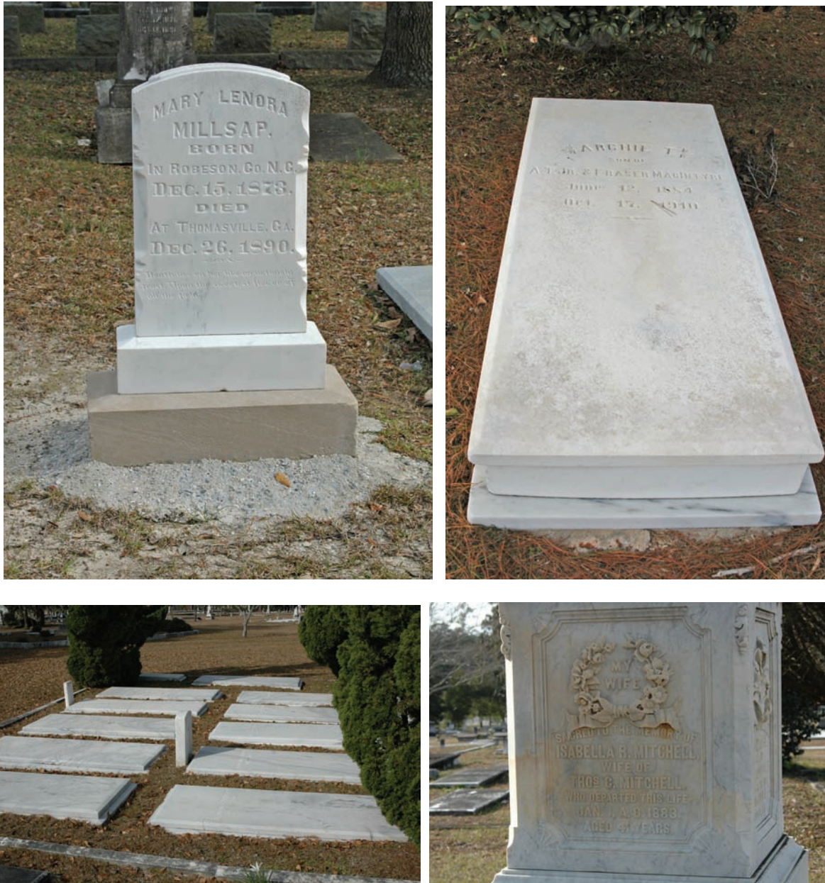
Figure 110. Examples of incorrect cleaning are found throughout Laurel Hill and these practices are causing significant damage and disfigurement. From upper left to lower right: monument cleaned using acid, resulting in surface erosion (this monument is also set too high, on a mass of Portland cement); ledger inappropriately cleaned with acid; entire plot cleaned with acid which destroys the historic patina and makes it appear as though the stones were set yesterday; monument cleaned with sodium hypochlorite leaving a yellow stain.
