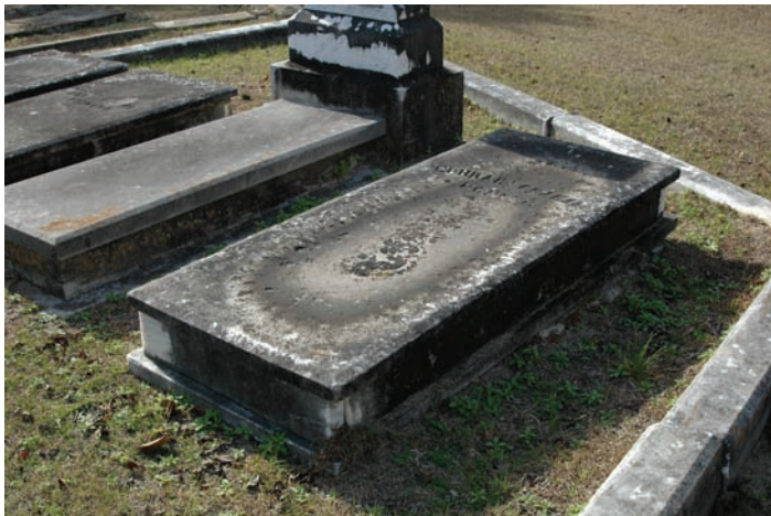
Figure 109. Example of a warped ledger showing water ponding on it.
