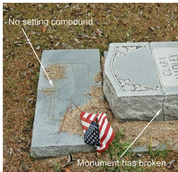
Figure 73. One example of an incorrectly set monument that has fallen and is now broken.
