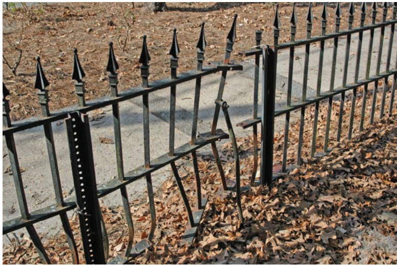
Figure 19. Damaged fence section. This requires disassembly, straightening, and replacement. Note also the sign supports holding up the fence.
