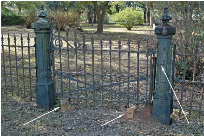
Figure 20. Boundary fence gate supported by bricks and wire.
