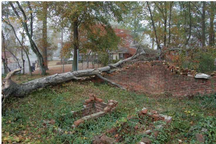
Figure 14. Rotted hackberry branch and pre-existing damage to the cemetery wall.
