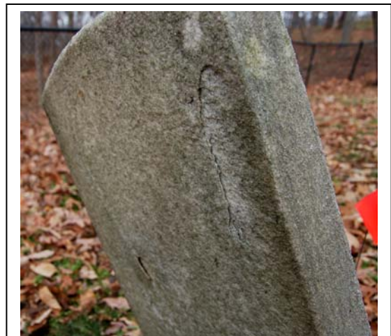
Figure 40. Example of spalling marble.
