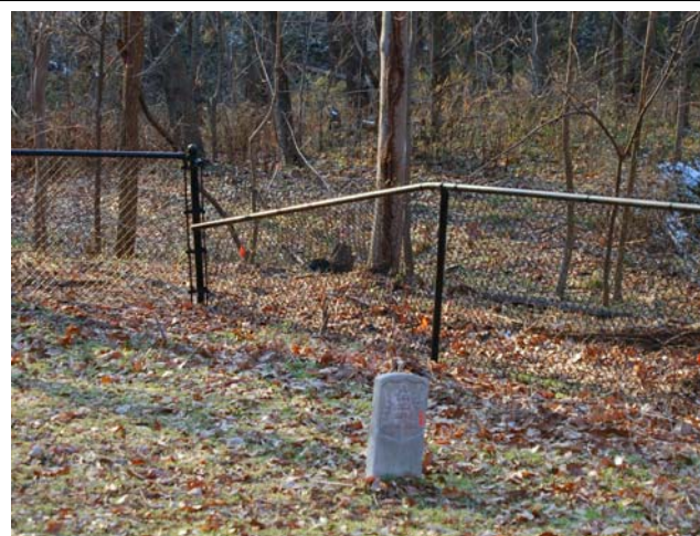
Figure 30. Damage to the chain link fence at the cemetery.
