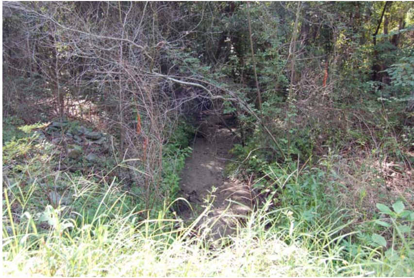
Figure 4. View of a ditch running through the project area.
