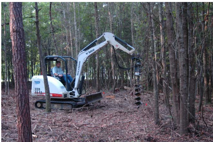
Figure 5. Using a Bobcat to auger at 38CH1693.
