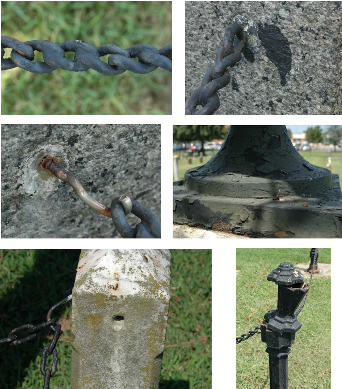
Figure 13. Extensive problems with historic fencing and monuments in the cemetery. Upper left, paint so heavily applied that details are obscured and the chain links are bonded; upper right, paint applied to the stone; middle left, inappropriate repair; middle right, heavy paint flaking and corrosion on the urn; lower left, missing and damaged connectors; lower right, heavily damaged fence post showing corrosion resulting from water penetration.
