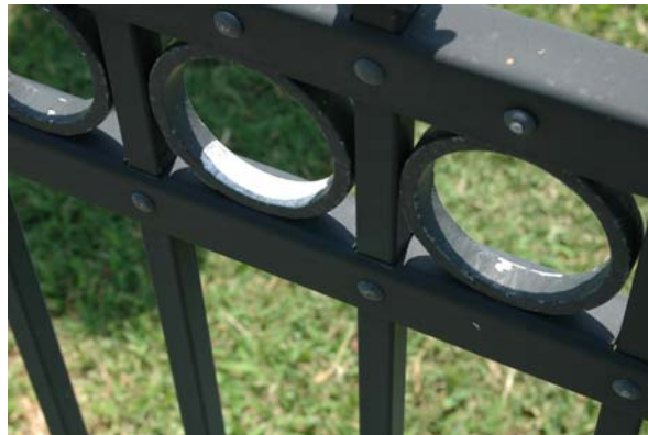
Figure 11. Modern boundary fence. The top photograph shows the heavy, out of scale appearance of the fence. The lower photographs illustrate paint dulling, chips with underlying corrosion, and flaking from galvanized trim. Note also the abundant use of rivets that detracts from the overall appearance.
