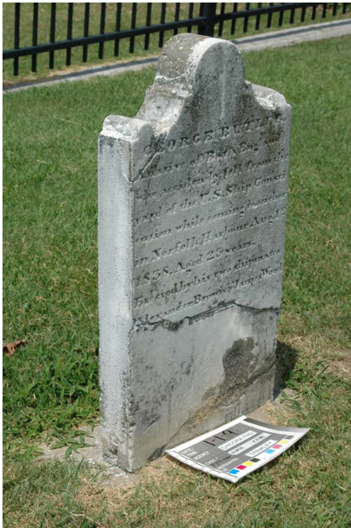
Figure 23. Use of white Portland cement to reinforce a monument, dramatically increasing its thickness and changing its overall character.
