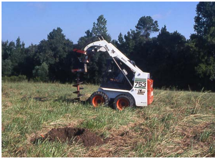
Figure 6. Auger testing with 18-inch power auger.
