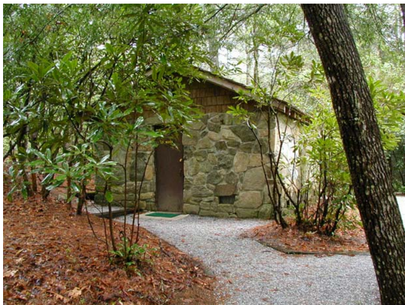
Figure 22. Van Hook bathroom structure.
