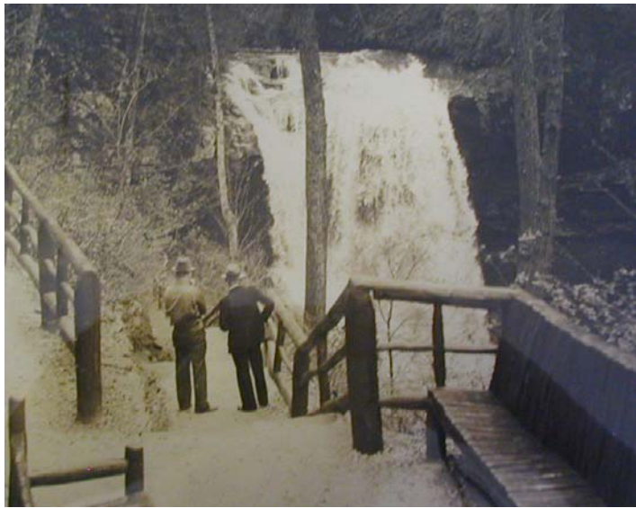
Figure 21. Historic photograph of Dry Falls, showing what was probably the original CCC wood railing and wood bench – none of which remains today.
