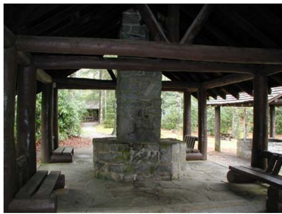
Large pavilion (C, Cook Shelter, in Figure 16). Note infilling of cook hearths.
