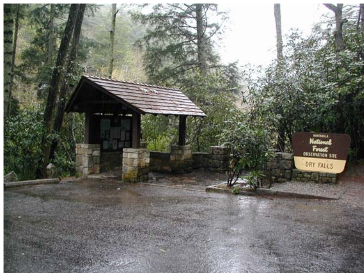
Figure 20. Entrance to the Dry Falls site today. Note the rebuilt registration shelter and different rock work at the entrance.
