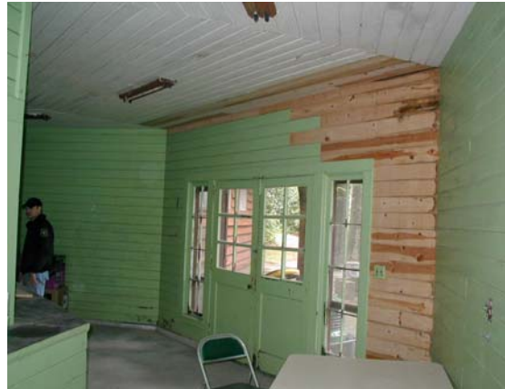
Interior of bath house with repairs.
