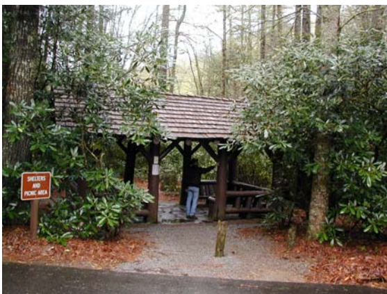
Small pavilion (B, Registry Shelter, in Figure 16).
