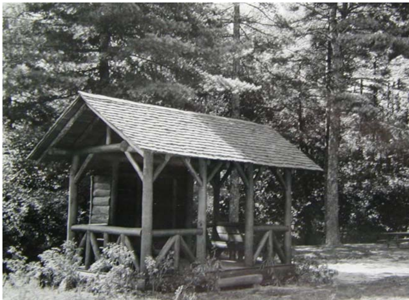
Figure 23. Registration shelter at Van Hook, possibly of CCC construction, that is no longer present.
