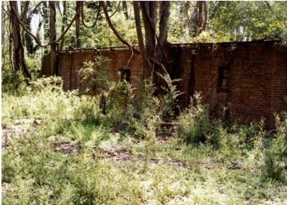
Kitchen building, looking to the southwest. Note the use of narrow gage rails for shed roof.
