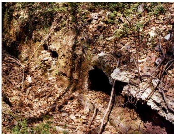
Section of exposed brick flue, showing flues running to kilns.
