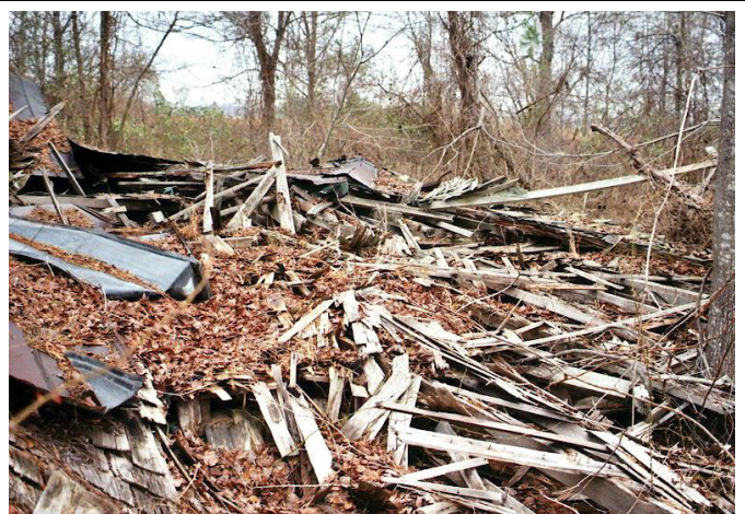
Figure 6. View of collapsed structure, looking west.
