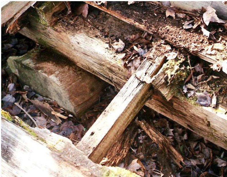
Figure 7. View of central rough hewn sill, joist with circular saw marks and log pier, looking to the southwest.
