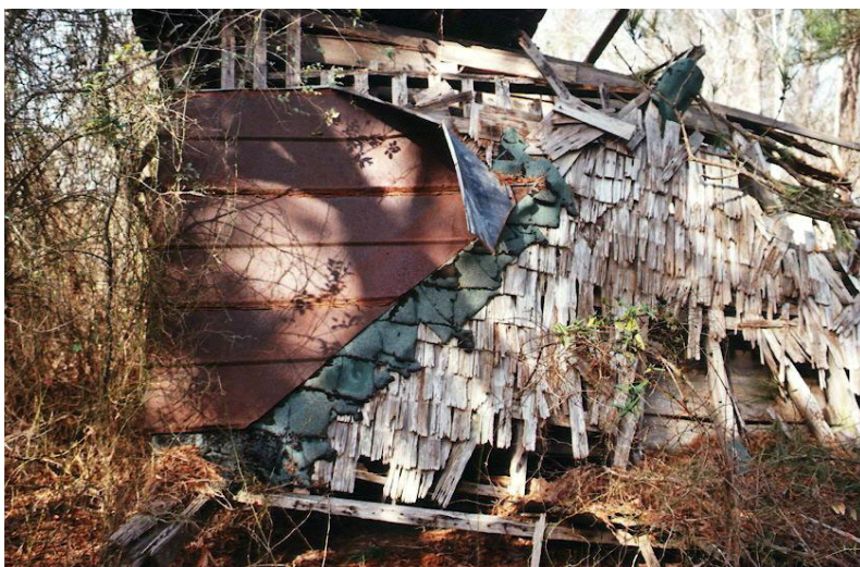
Figure 8. Roofing materials. View to the north.
