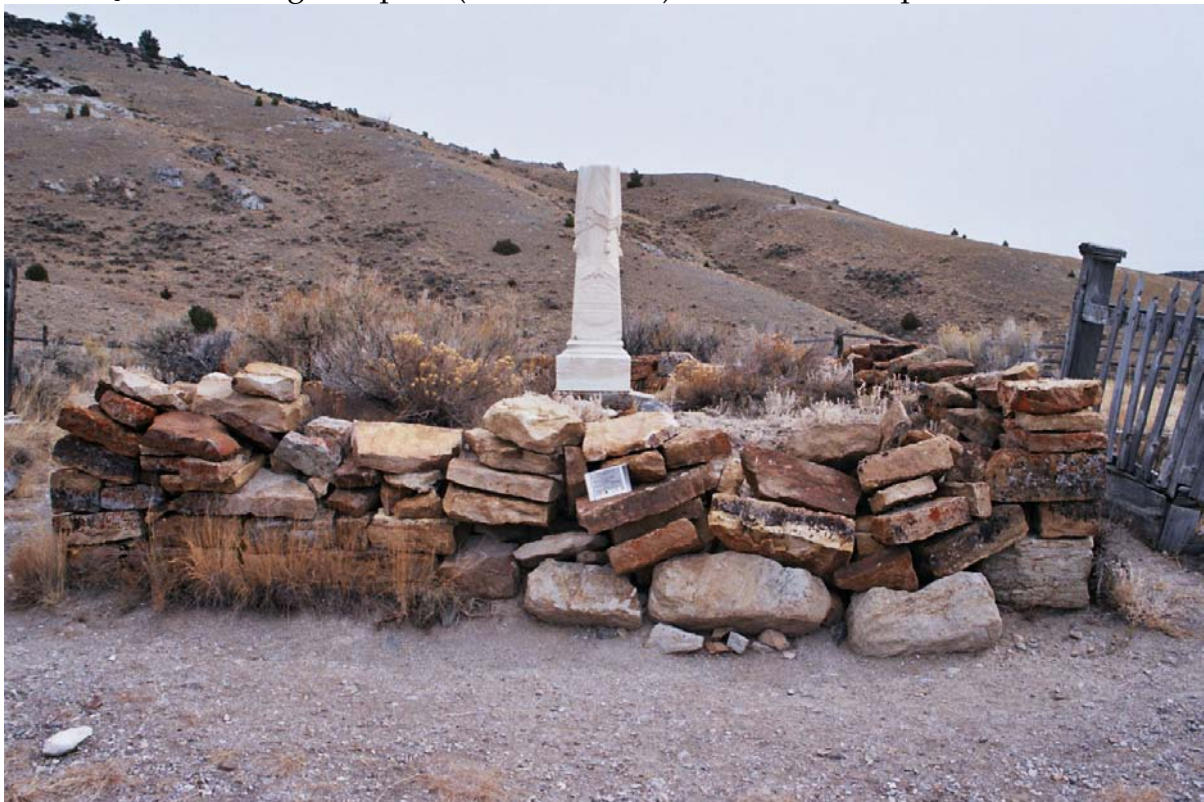
West façade showing collapsed (and restacked) wall and Trask pedestal tomb
