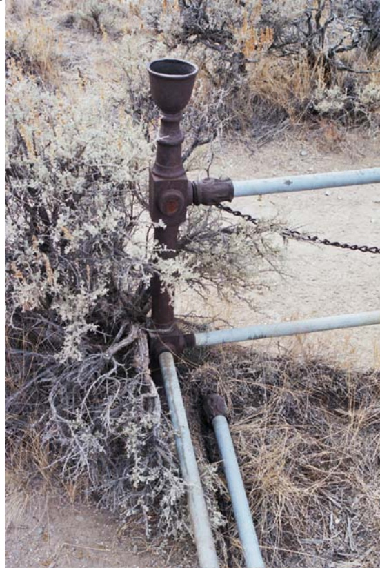
Fence at Plot 22, close-up of corner post design
