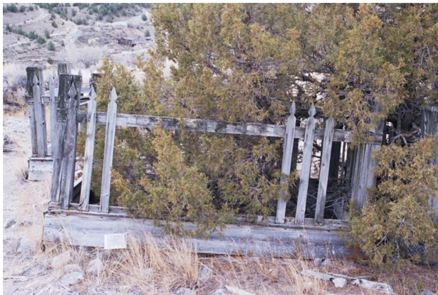
Figure 7. Example of a grave fence (Grave 21) in better condition showing the loss of fabric. The juniper tree, a recent volunteer, should be removed.
