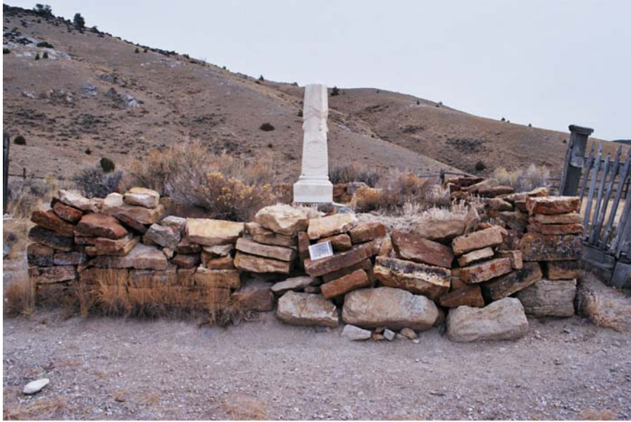
Figure 4. The Trask monument and associated dry-laid cut sandstone wall. View is to the southeast.
