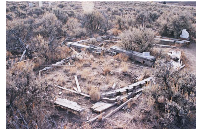
Figure 26. Fence at Plot 97 showing collapsed fence. In such a case a new skeleton fence should be erected and whitewashed, while the original fence is documented and allowed to remain in place.
