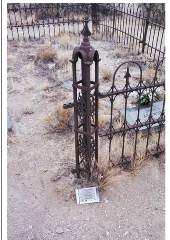
Figure 18. Fence at Plot 5 showing the open or scroll gate posts, bow and picket design on the front sections, and simple picket design on the remaining sides.
