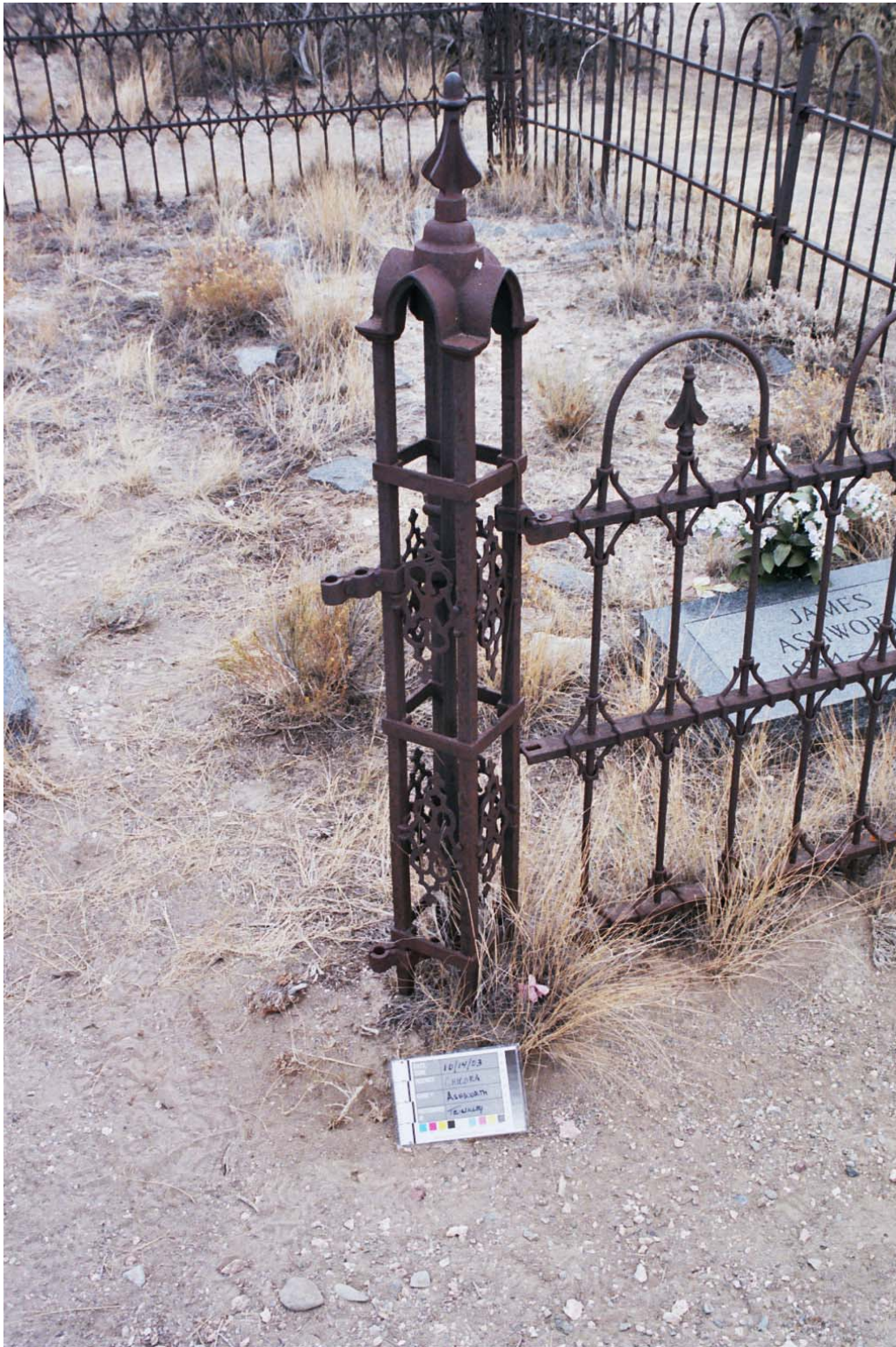
James Ashworth stone to the right; note also two types of ironwork design comprising fence
