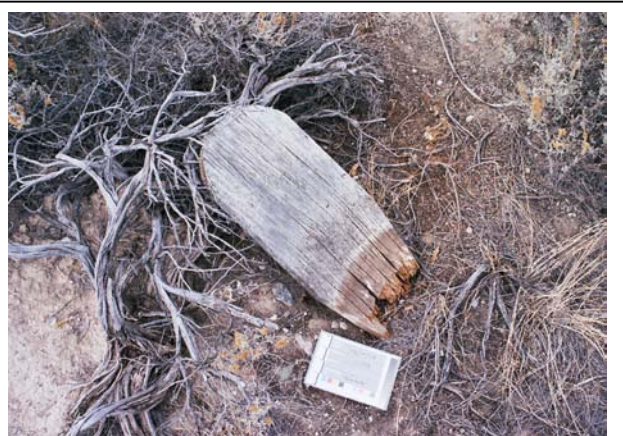
Figure 31. Example of wooden marker vandalized and broken off at ground level. This should be repaired using epoxy and stainless steel straps.
