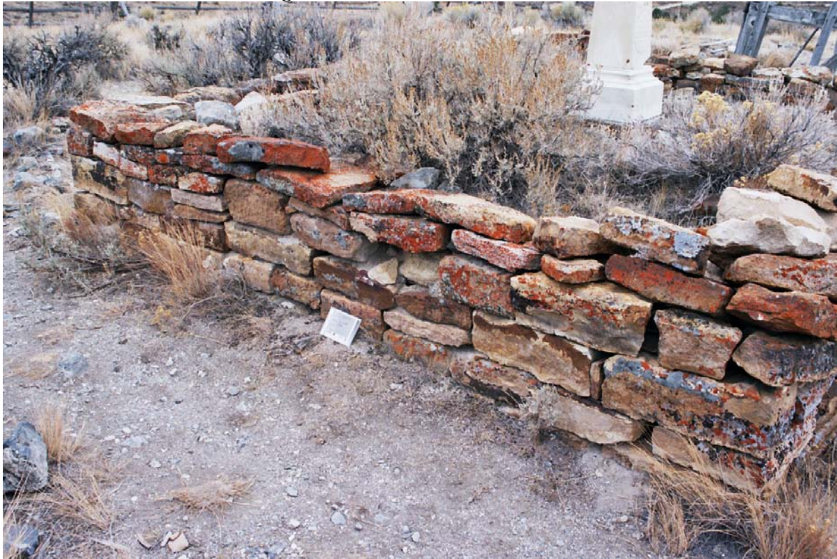
South façade of wall showing intact wall
