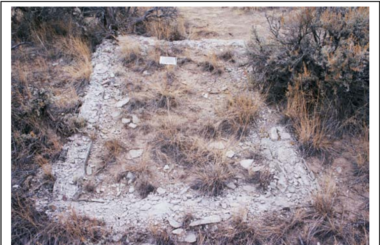
Figure 28. Grave coping at Plot 112 that has failed. Note the large cobbles used for aggregate.
