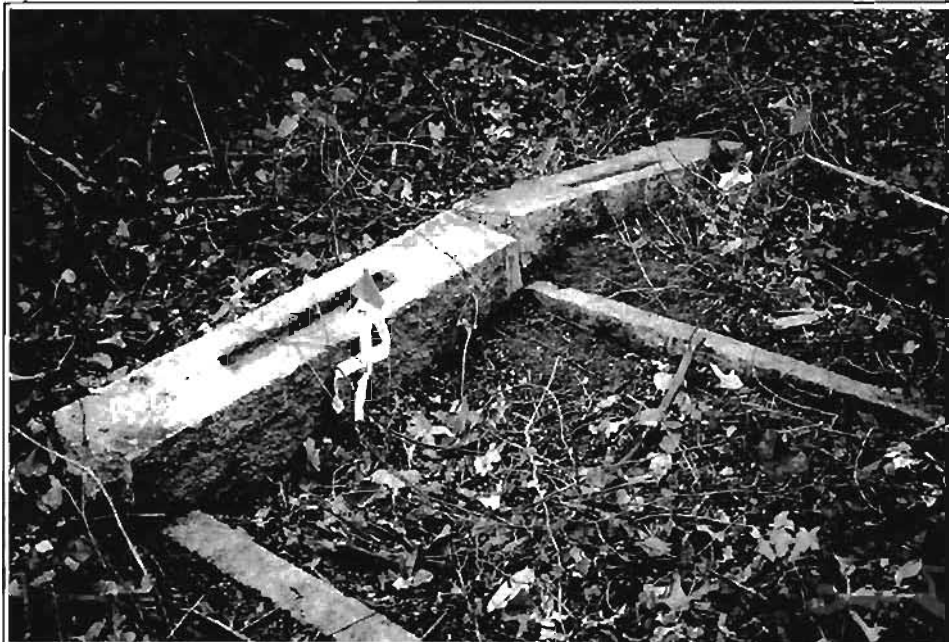
Figure 13. Granite bases with tabs and coping, view to the northwest. Dies are missing and the graves are collapsed, causing the bases and coping to be displaced.
