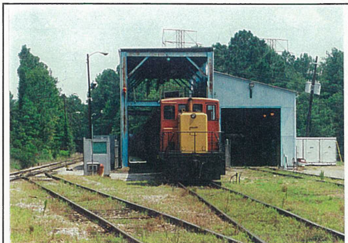
Figure 82. McMeekin Track Hopper House (2430127.06), view to the south.
