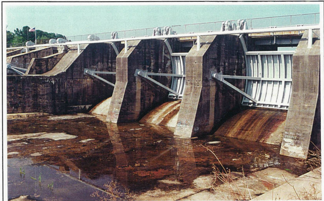
Figure 79. Tainter gates and spillway, site 2430127.03, view to the southwest.
