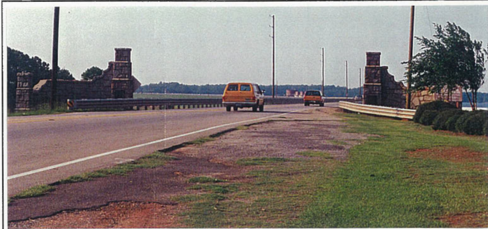
Figure 78. Stone entryway (2430127.02) at the north side of Lake Murray on S.C. 6, view to the south.
