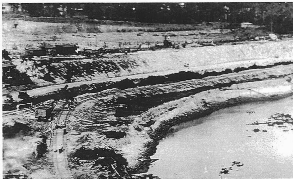
Figure 27. View east of the north bank of the Saluda, east of the dam in 1930. Note the extensive construction disturbance, including complete denuding of the floodplain area (courtesy of SCE&G).
