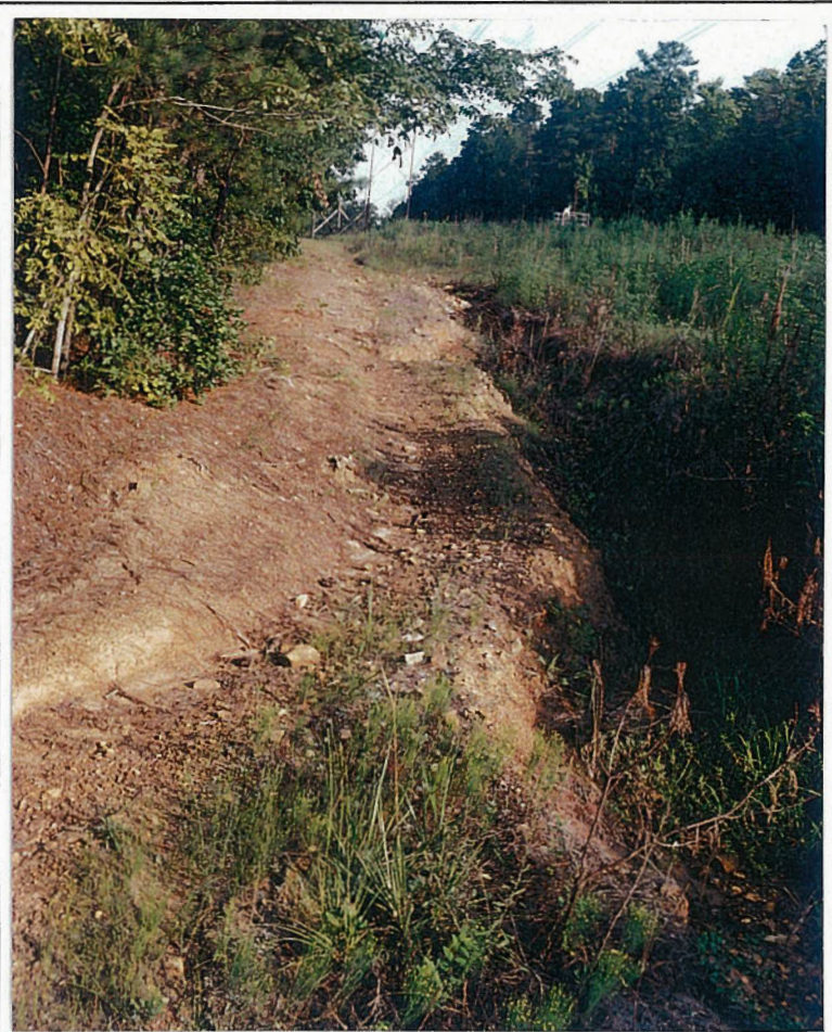
Figure 5. Area of still active erosion on a road adjacent to a powerline easement in the study area.
