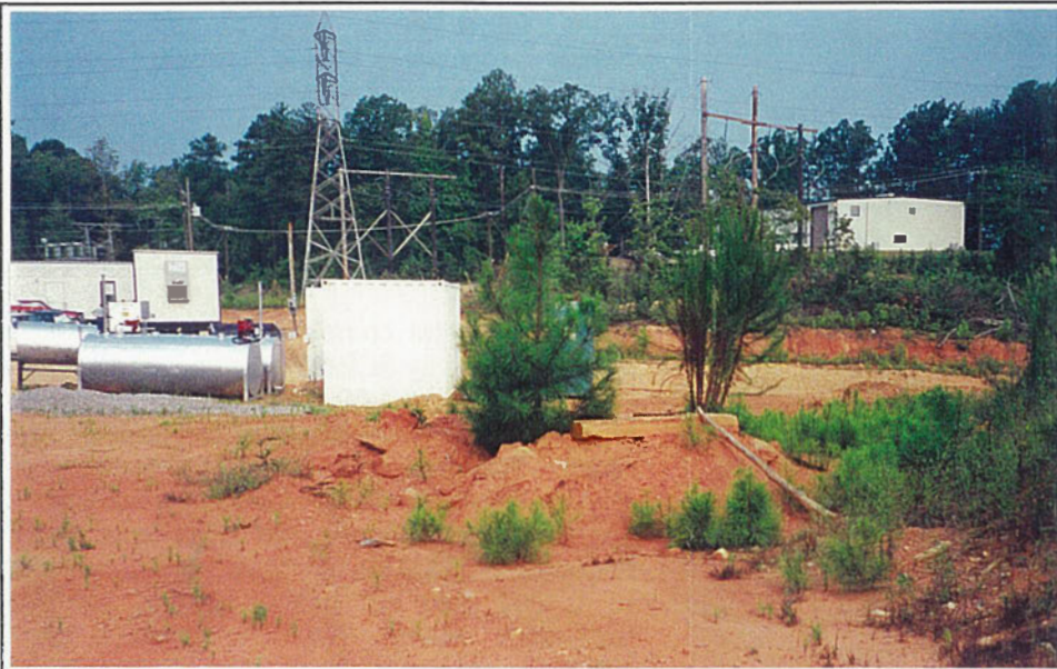
Figure 75. Vicinity of 38LX455, view to the north.
