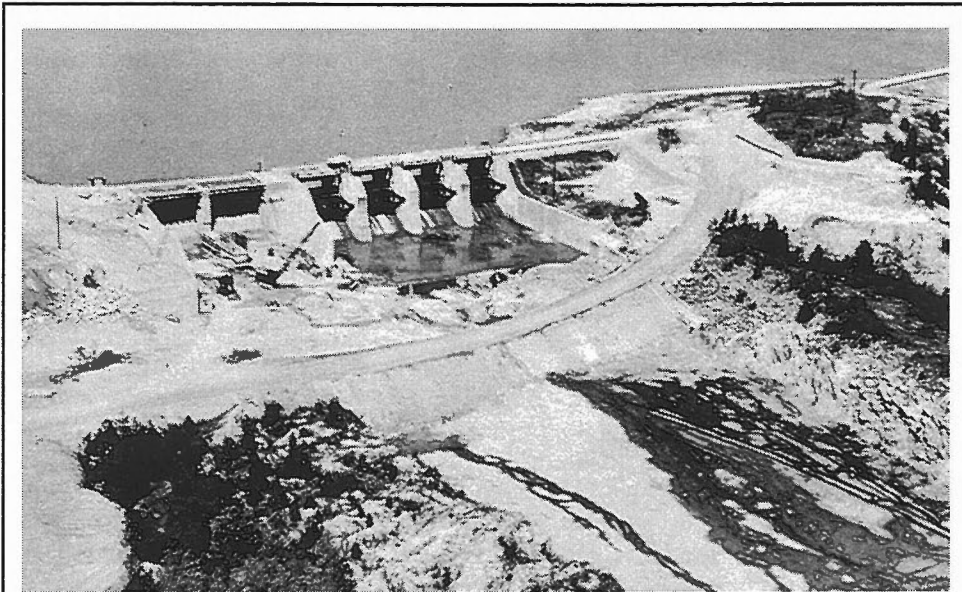
Figure 33. View of spillway gate construction, ca. 1945. The Yninger Cemetery is shown at the far right of the photograph (courtesy of SCE&G).
