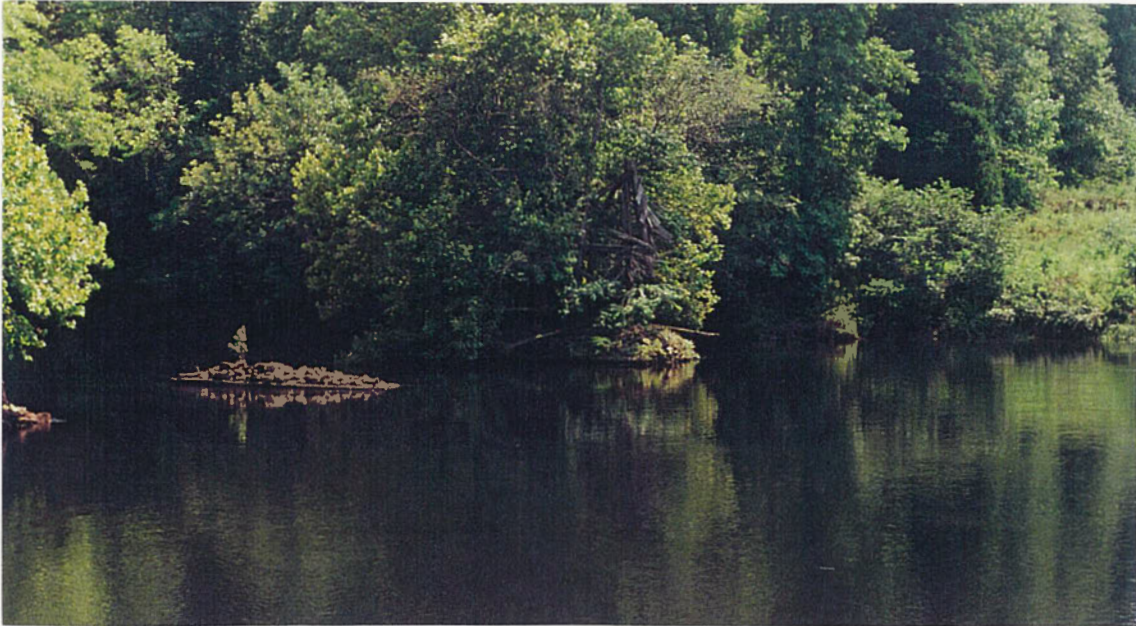
Figure 84. Remnant caissons for the temporary bridge across the Saluda River (2430128), view to the southwest.
