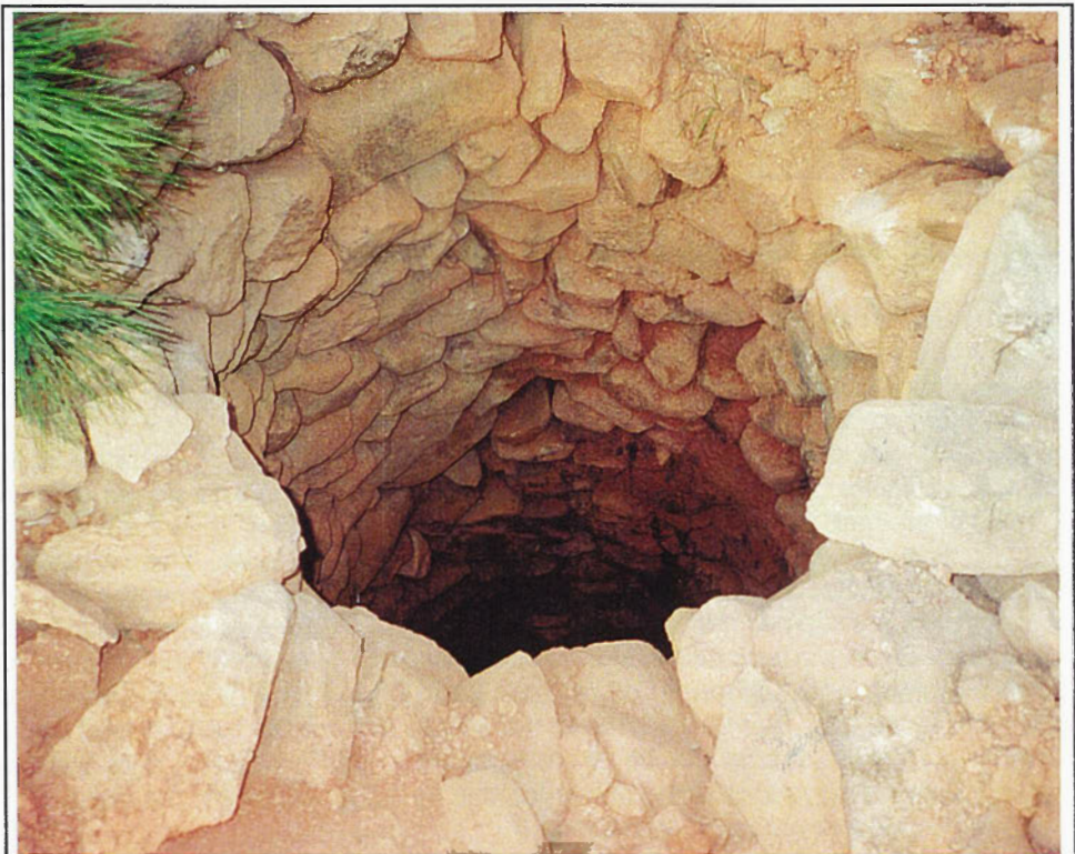
Figure 76. View of well showing construction using dry laid field stones.
