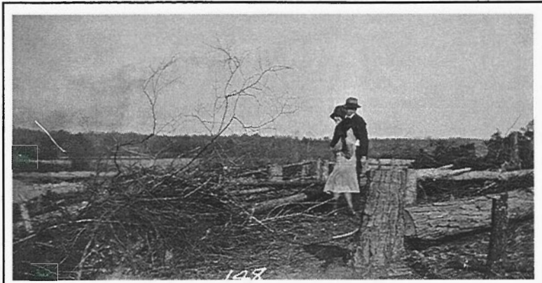
Figure 17. View of floodpool during logging (courtesy of SCE&G).
