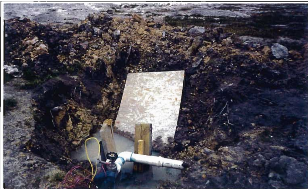
Figure 22. Example of construction activities that are likely to have damaged African American burials at the S.C. State Hospital Cemetery for African American patients.
