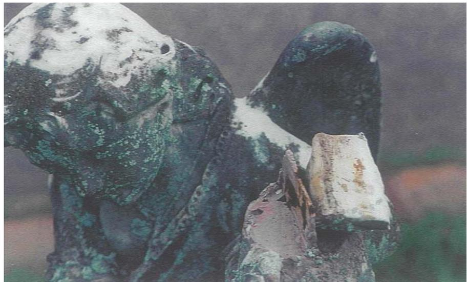
Figure 21. Broken cross (Lot I). Metal wedge will need to be removed before any repairs can be done.
