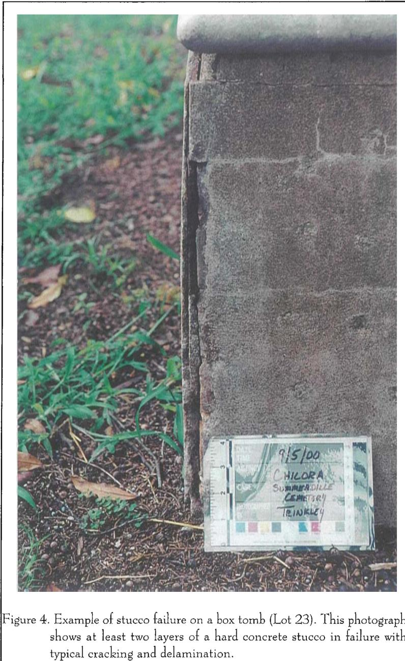
Figure 4. Example of stucco failure on a box tomb (Lot 23). This photograph shows at least two layers of a hard concrete stucco in failure with typical cracking and delamination.
