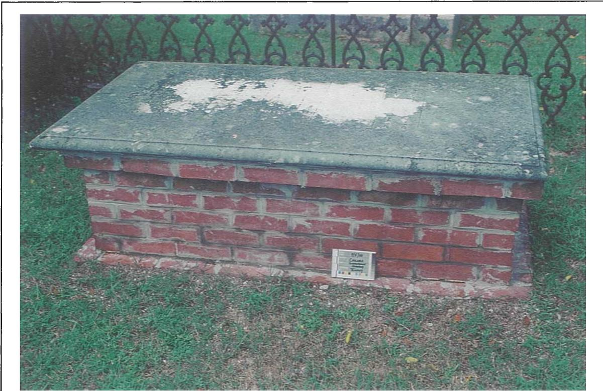
Figure 2. Rebuilt box tomb (Lot C). The use of modern brick and hard mortar, coupled with a lack of care in finishing the joints and cleaning the brick has resulted in an inappropriate “restoration” that detracts from the historic integrity of Summerville Cemetery. Such work should not be allowed.
