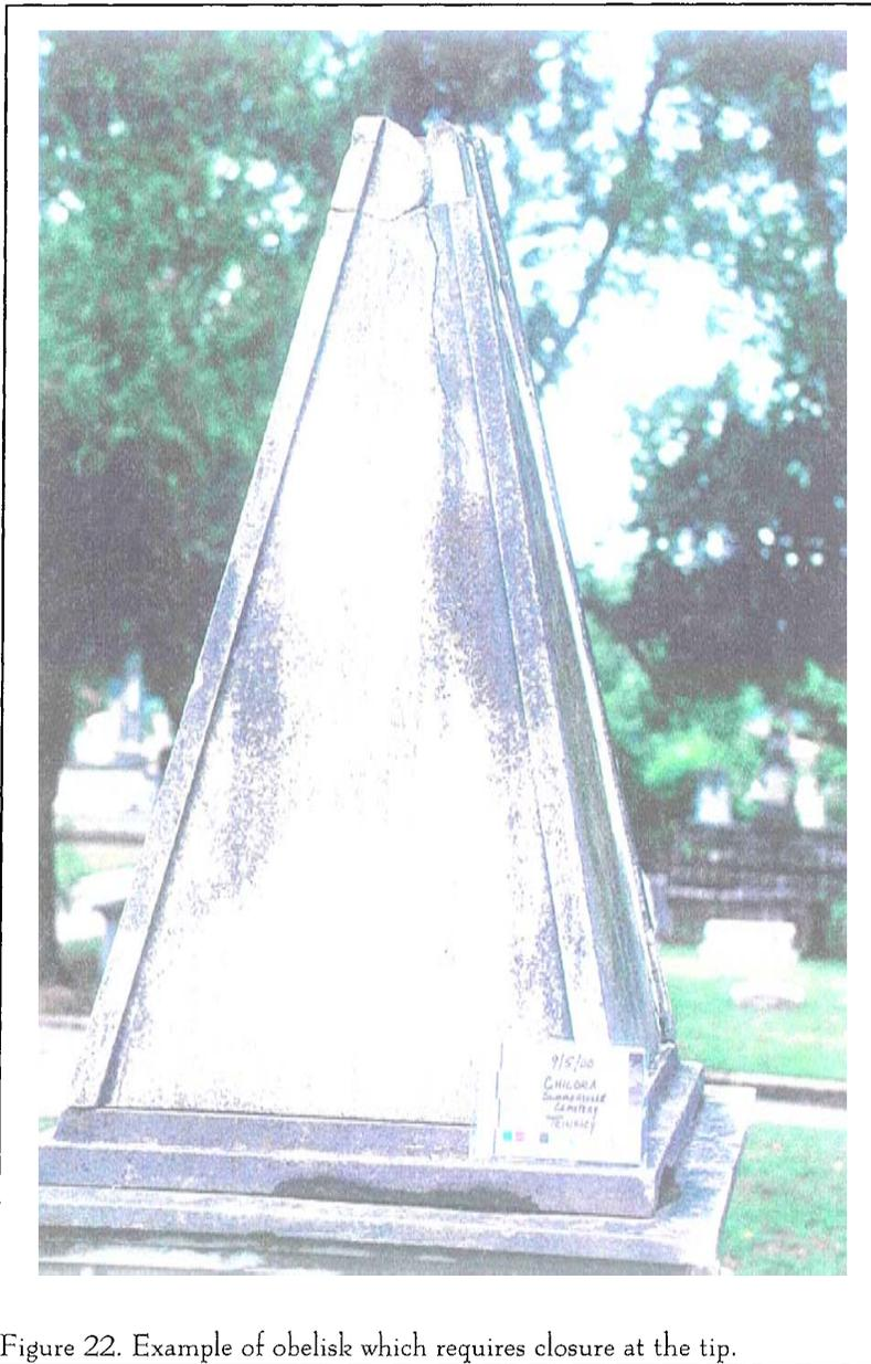
Figure 22. Example of obelisk which requires closure at the tip.
