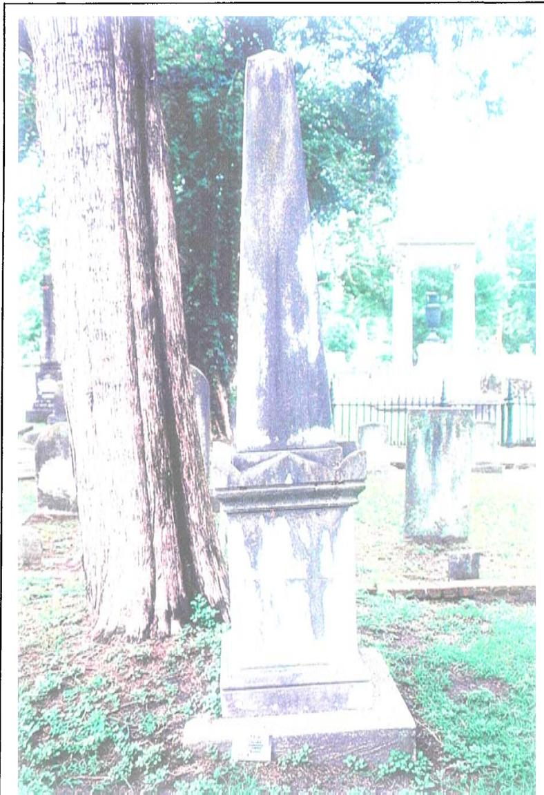
Figure 15. Example of leaning obelisk (Lot7). This stone will need to be disassembled, a foundation established, and the stone erected again.
