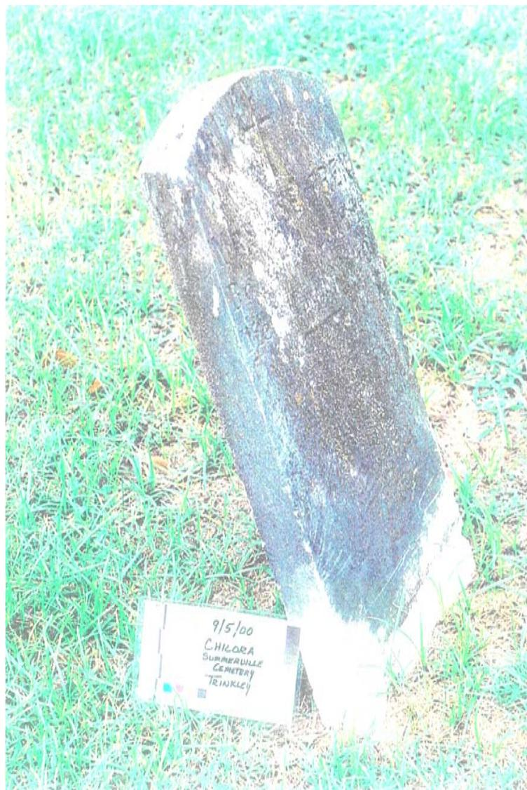
Figure 5. Example of mower damage (Lot 45). This marble head stone, which needs to be reset, also shows evidence of extensive mower damage (the nicks and lost material on the edges) as well as improper use of nylon string trimmer (the parallel “scratches” across the stone face). This is evidence of improper mowing techniques and a lack of care.
