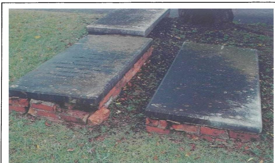
Figure 27. Deteriorating brick supports for ledgers (Lot 147).
