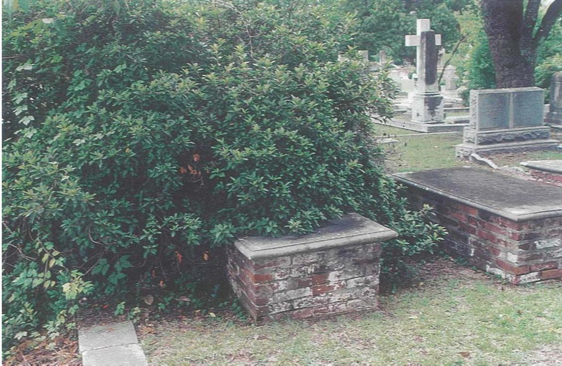
Figure 6. Example of unpruned plant taking over Lot 40. This azalea needs careful pruning for both its health and also to remove it from the box tomb. This dense vegetation will ultimately result in deterioration of the marble and the mortar joints.
