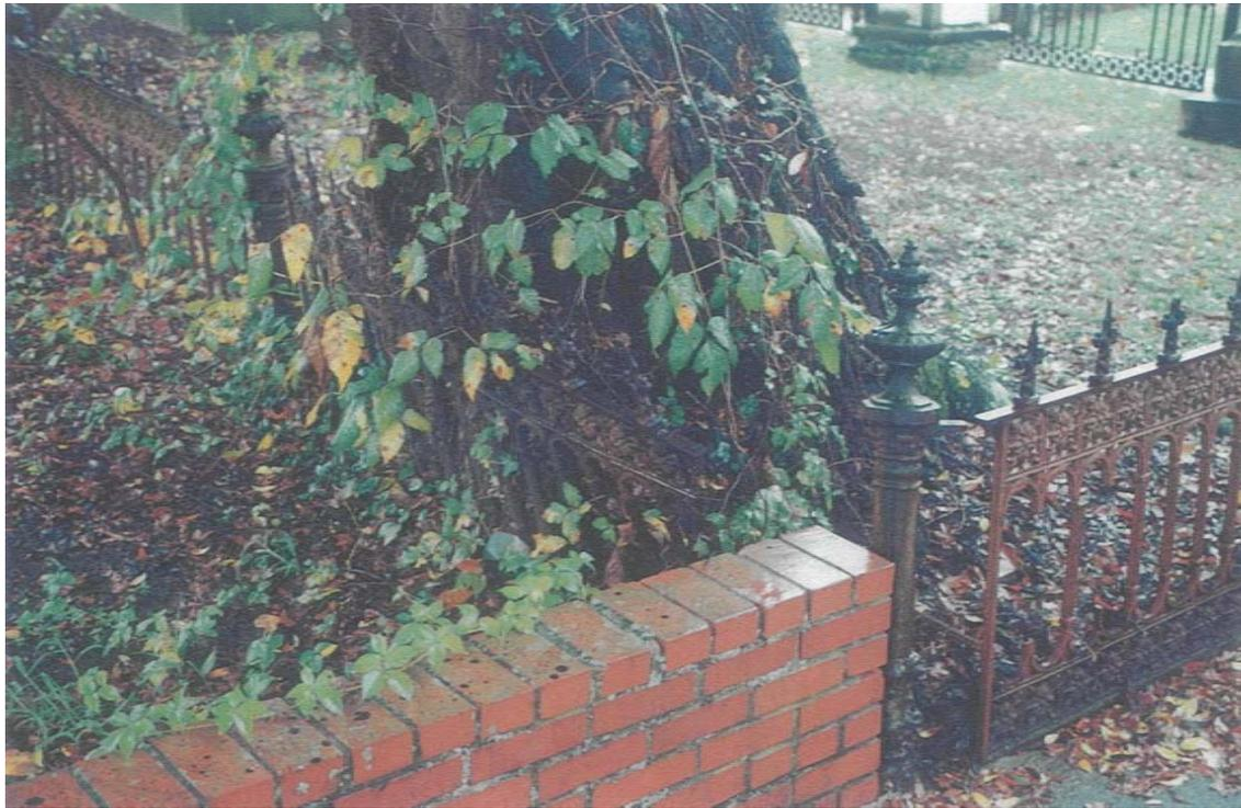
Figure 29. Example of tree which has been allowed to damage a fence segment (Lots 16/17). In this case the only choice is to remove the fence section and place it in storage. The aisle way segment should also be reattached to the corner newel post. This photograph also illustrates the large quantity of poison ivy which has been allowed to grow unchecked in the cemetery. This must be removed before any ironwork can begin.
