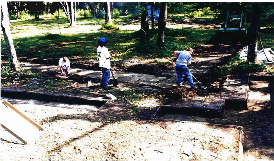
Figure 16. Cleaning bulldozer trenches.
