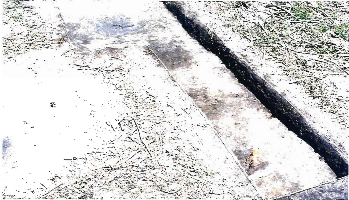
Figure 18. Displaced pier in TU3.
