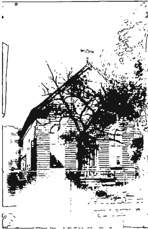
Figure 7. The first Immaculate Conception Church at the corner of Shepard and Coming streets, built in 1880. This photograph shows a rear addition and likely dates from the 1930s.
