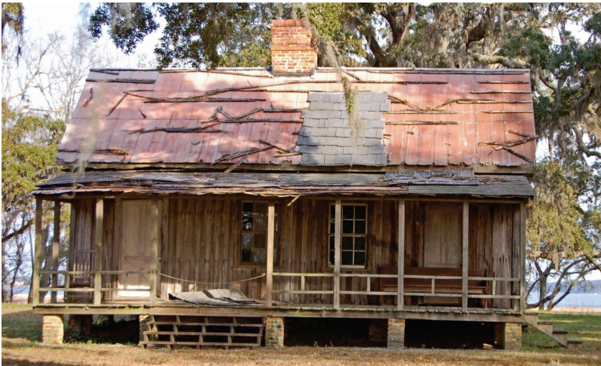
Figure 92. Standing structure at 31BW787**7. Top photograph is an oblique view to the southeast. Below is a view of the front, looking east.
