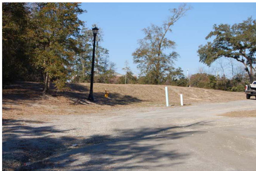
Figure 10. View of roads and utilities already put in the project area (site was located at the top of the hill).
