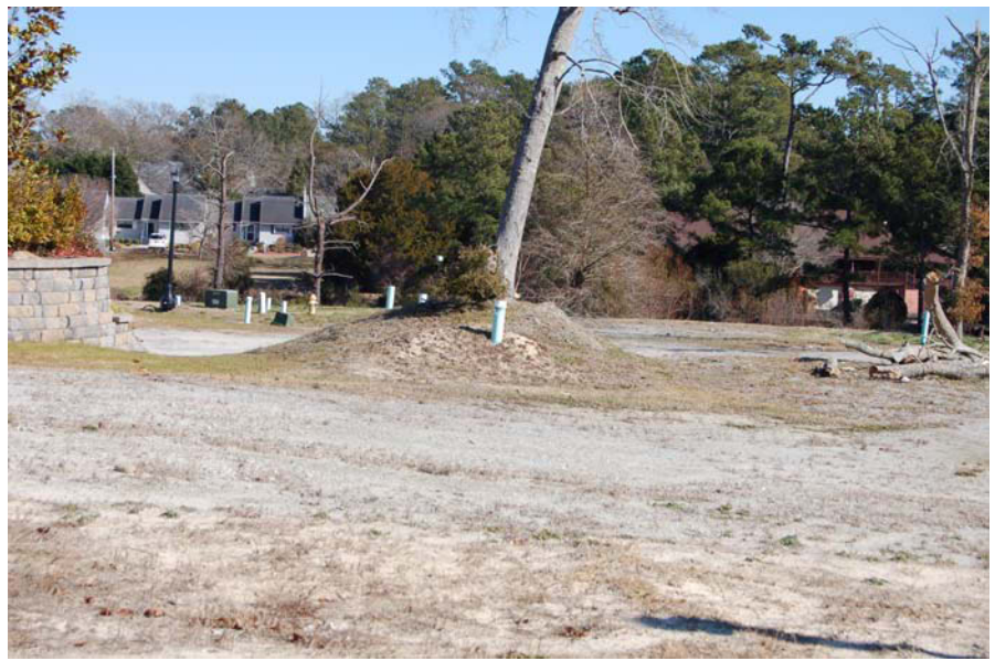
Figure 3. View of the former ground surface showing the large amount of soil displaced.
